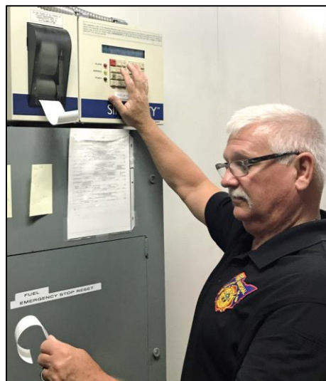
Fig. 4 - Automatic tank gauging (ATG)
