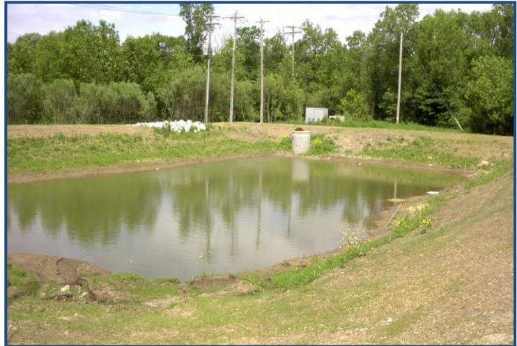
A sediment basin/trap can be an effective method to control runoff. Ohio EPA file photo.
