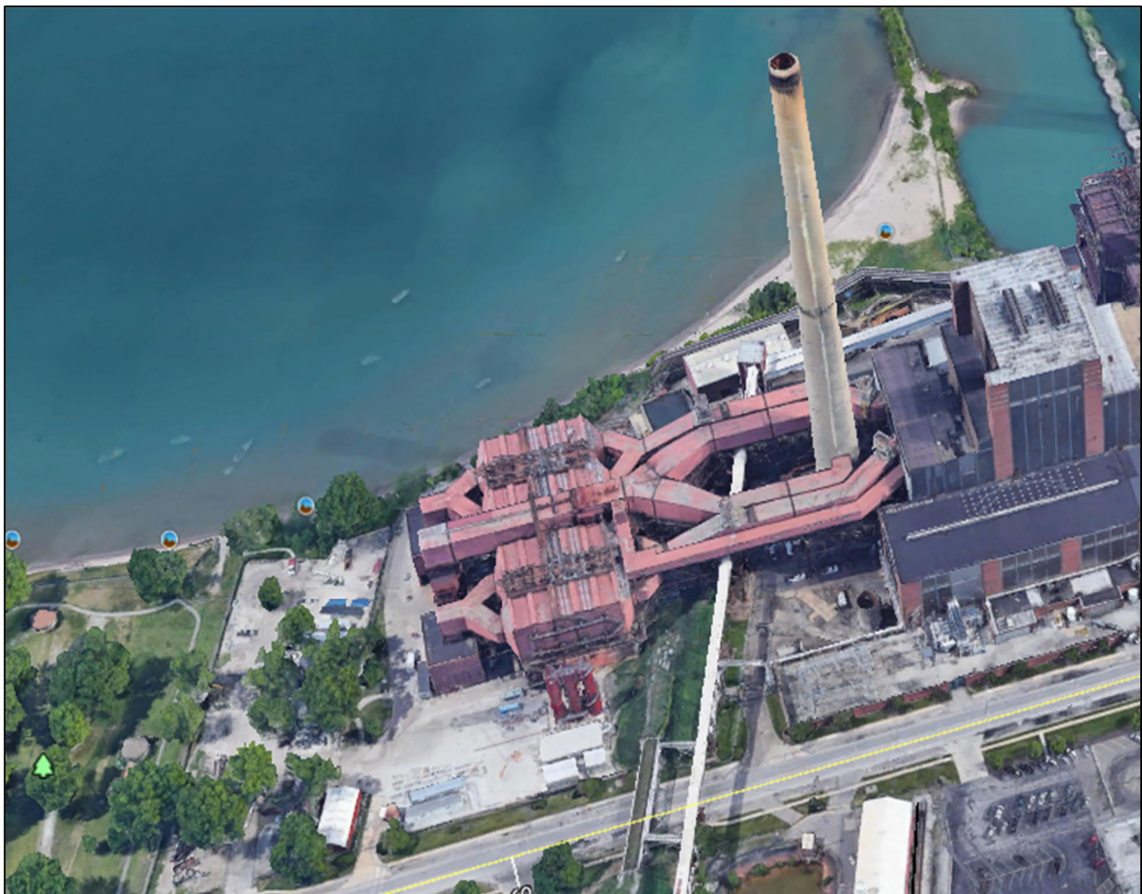
Figure 5-1 Avon Lake Power Plant Unit 9
