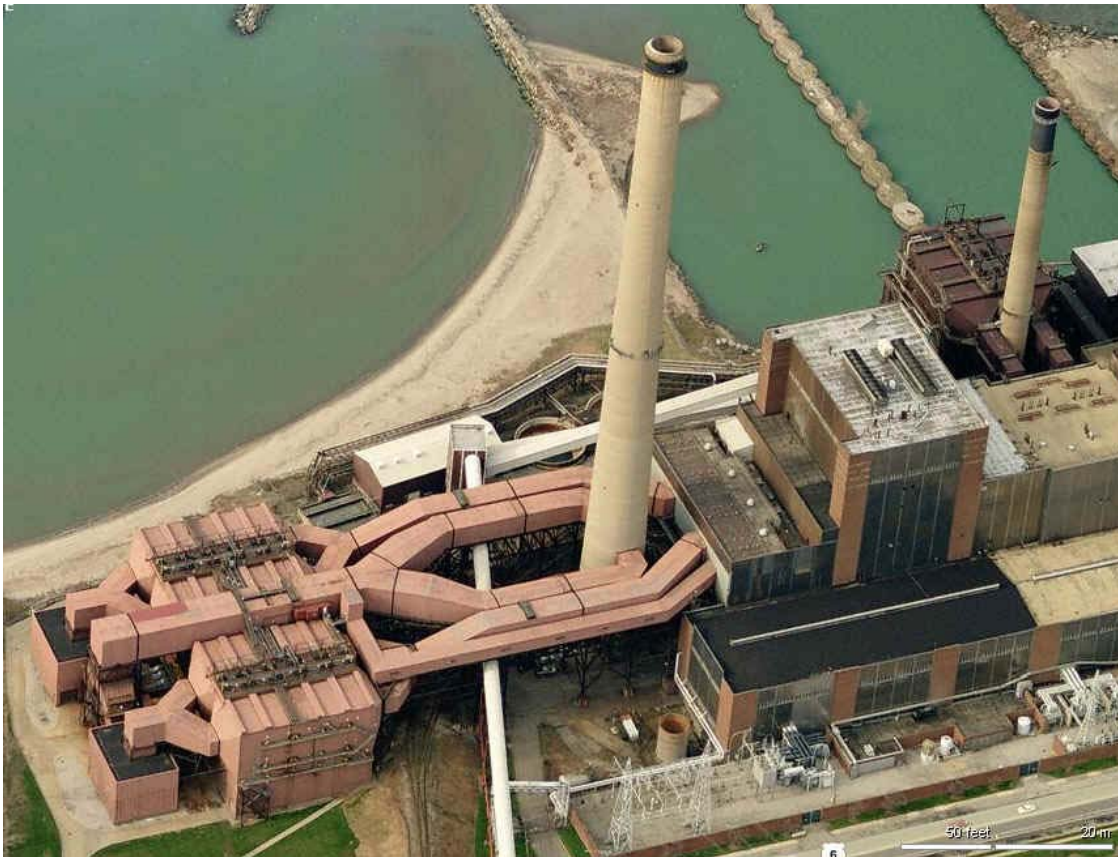
Figure 2.0-1: Aerial View of Avon Lake Unit 9.
