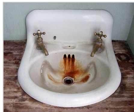
Figure 2. Sink discolored from high iron content in the water.
