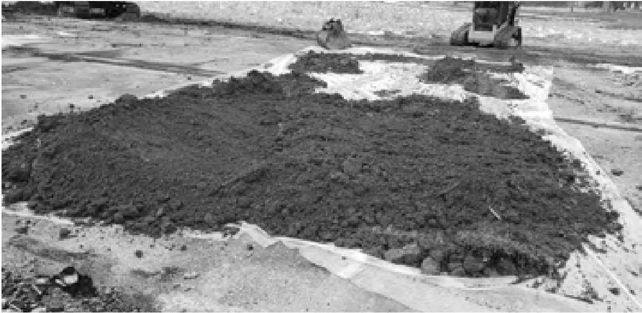
Fig. 15 Start of stockpile on concrete pad from top one foot of soil from REM-1.
