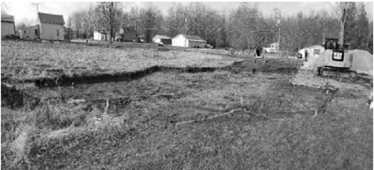
Fig. 16 Top one foot of soil removal from REM-1, facing northwest. Stockpile of excavated top one foot of soil is staged on pad and covered on the right.
