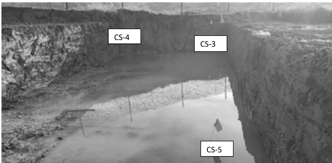
Fig. 21 Flags denote confirmation sample locations, (from left background to foreground on right) CS-4, CS-3, and CS-5 (floor sample).
