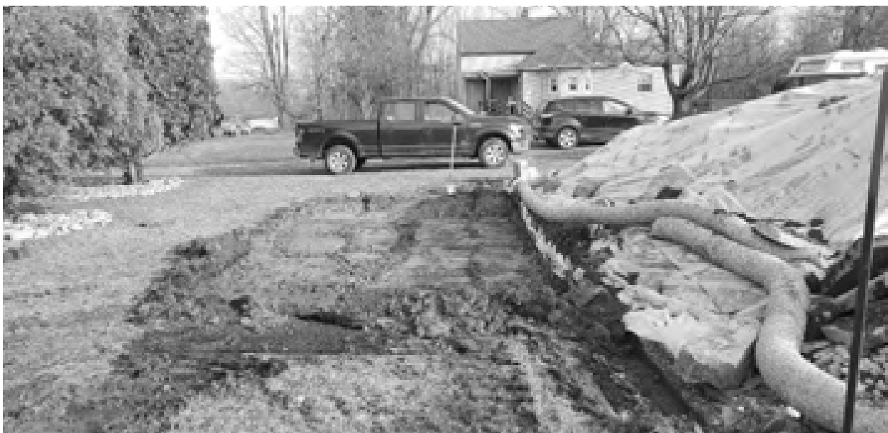
Fig. 19 REM-2 post excavation of top one foot of soil on left. Covered stockpile on right.
