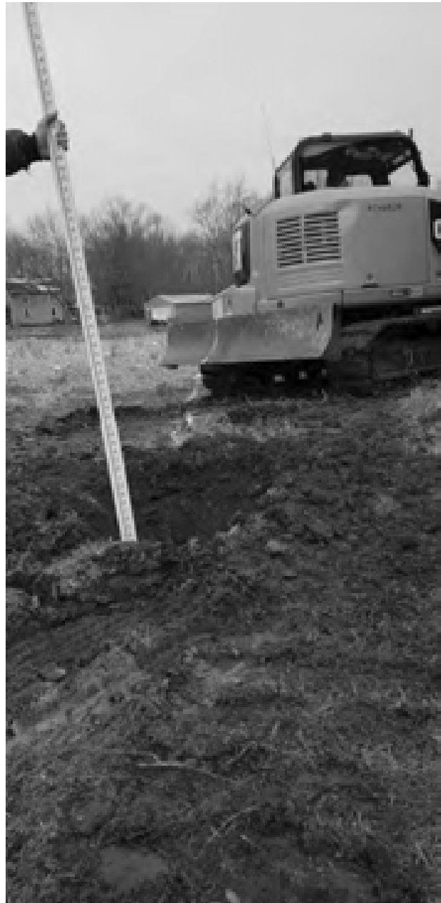
Fig. 14 Excavation down to 2.5 ft. at SO-19.
