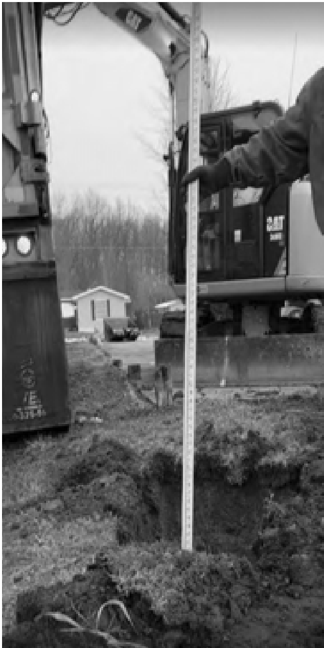
Fig. 13 AS-6 excavated to 4.5 ft.
