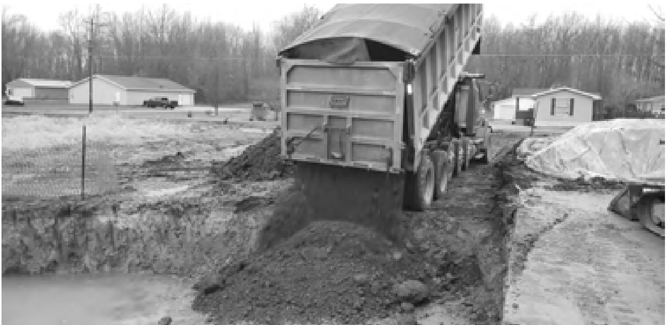
Fig. 26 Beginning of backfill activities.
