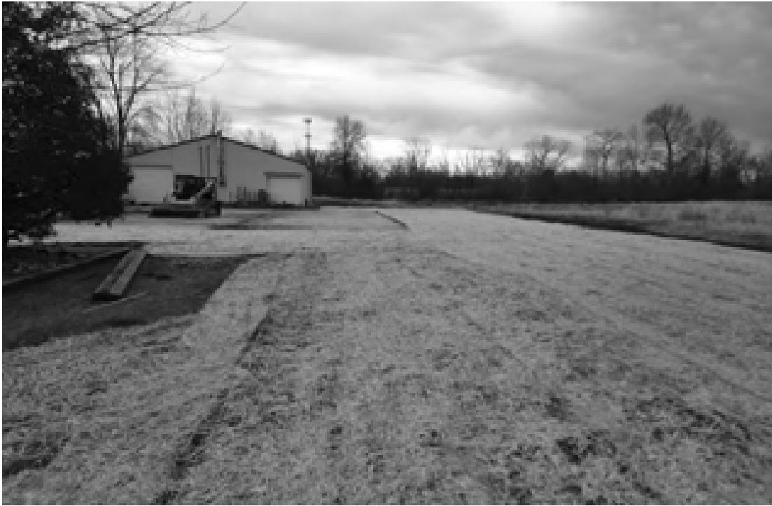
Fig. 31 Seed and straw applied to entire work area.
