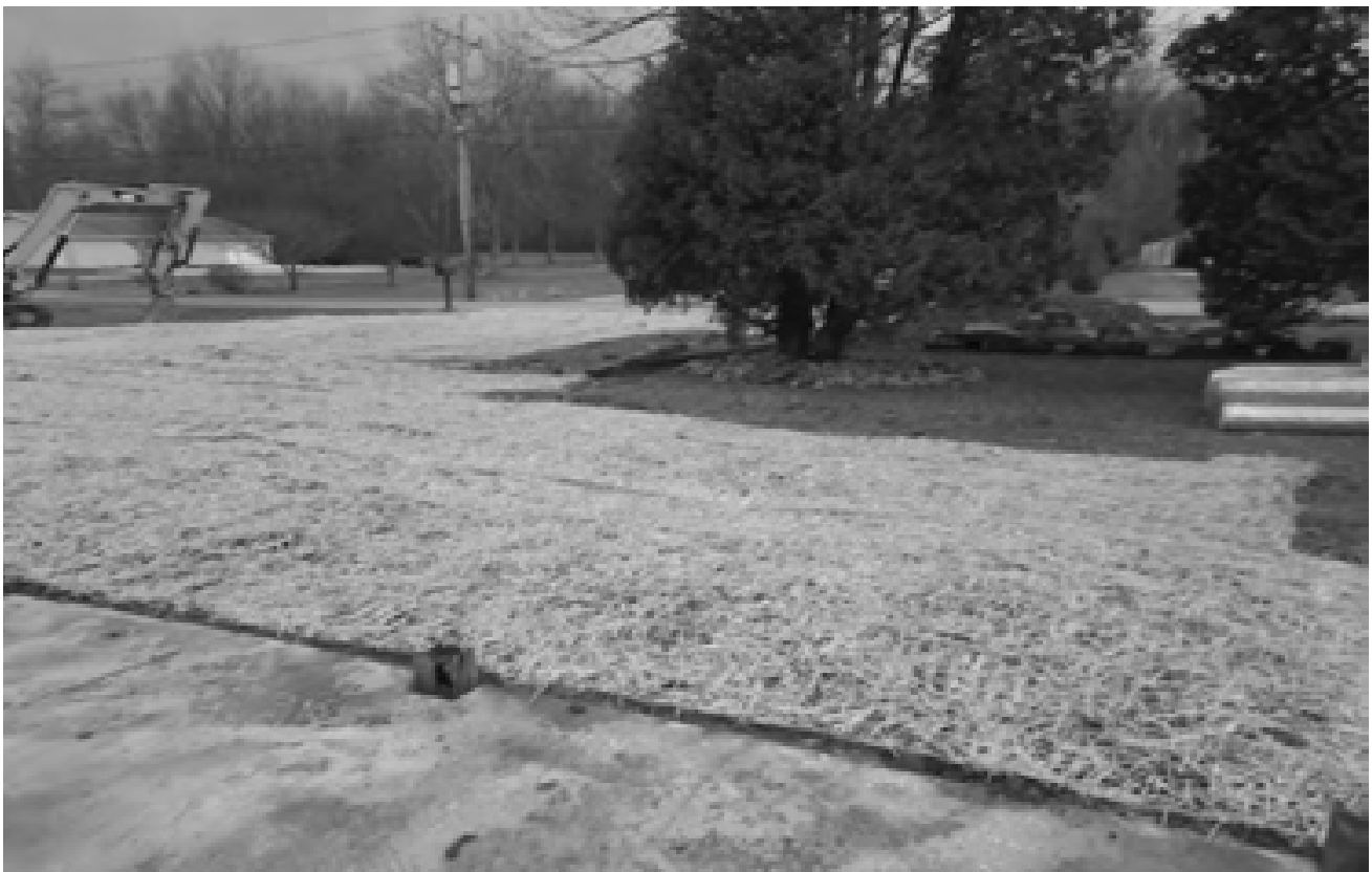
Fig. 30 Seed and straw applied to backfilled areas, REM-2 in foreground.
