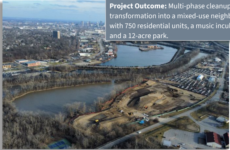
Photograph 5 – Aerial view of the property circa Fall 2024 from Thrive Companies.
