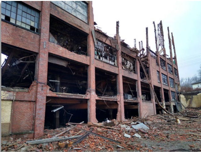
Photograph 3 – The property mid- demolition in January 2024. Courtesy of Mark Price, Akron Beacon Journal.
