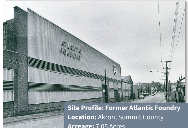
Photograph 1 – The Property prior to remediation, circa 1989.
