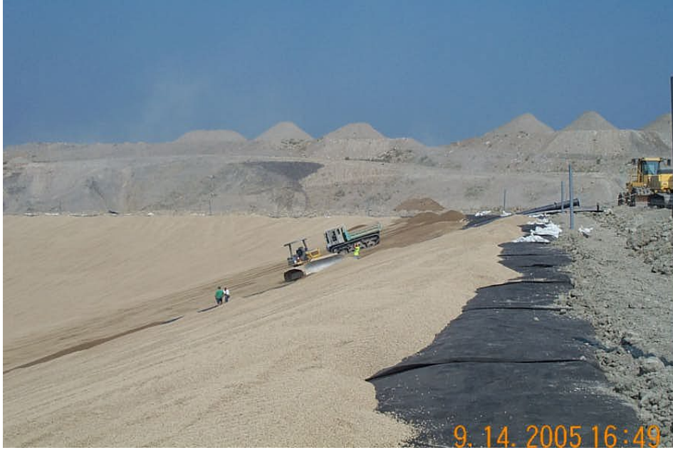
Figure 9-6, Stable slope of 1 ft of pea gravel on 3 to 1 slope after being placed with a low ground pressure Caterpillar D6 and IHI crawler carrier (5.8 psi). The calculated factor of safety for equipment loading conditions was 1.041 (interface \approx a=70 psf and \delta=18.3^\circ , drainage layer \approx c=0 psf and \phi=37^\circ ).
