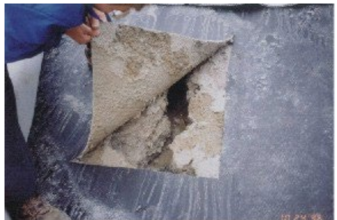
Figure 7-5 Piping failure in recompacted soil liner at an Ohio landfill
