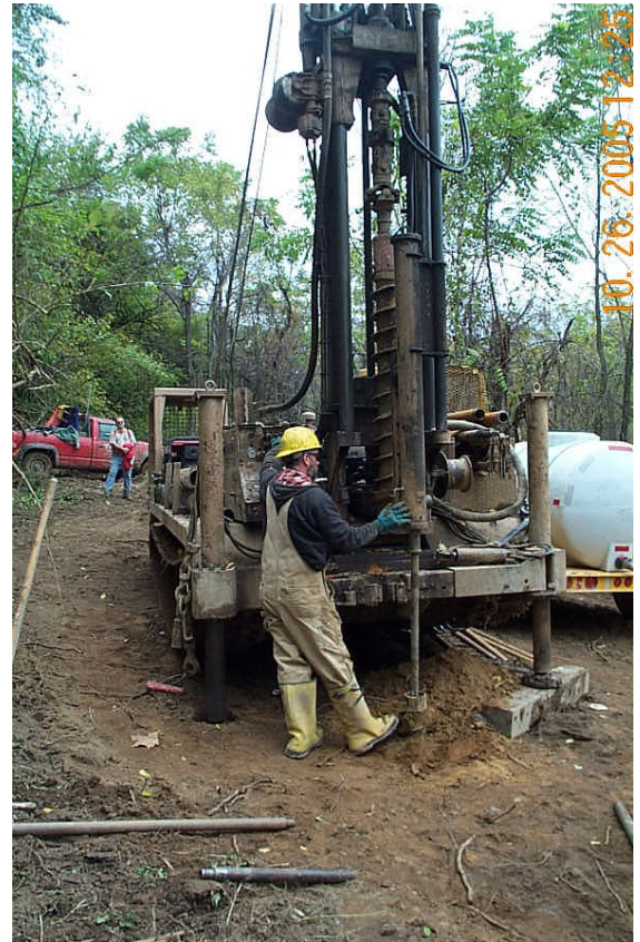
Figure 3-1: Drill rig and operator conducting a standard penetration test (SPT).
