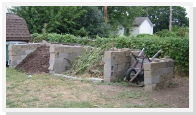
A 3-bin composting system in Montgomery County, Ohio.
