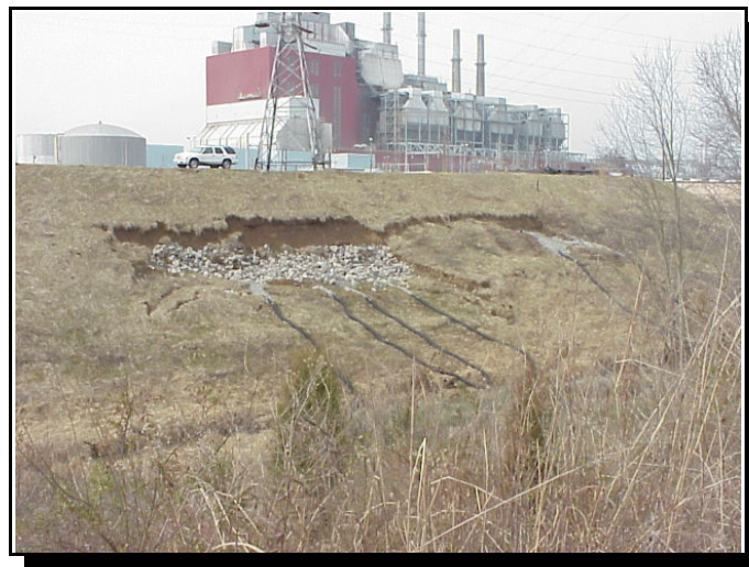
Figure 9-5 A shallow rotational failure in a containment berm at an ash settling pond in Ohio.
