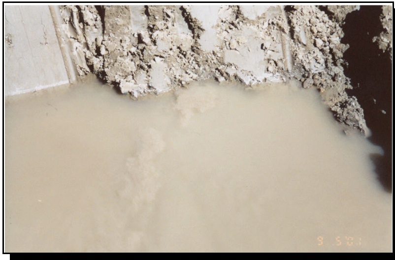
Figure 7-6 This is another example of hydrostatic pressures at an Ohio landfill causing flow through more than 20 feet of heavy in situ clay materials resulting in flooding of the excavation. Note that in this case, the presence of water cannot be taken into account due to precipitation. The flow of uplift water is evidenced only by a cloudy disturbance in the flooded excavation.
