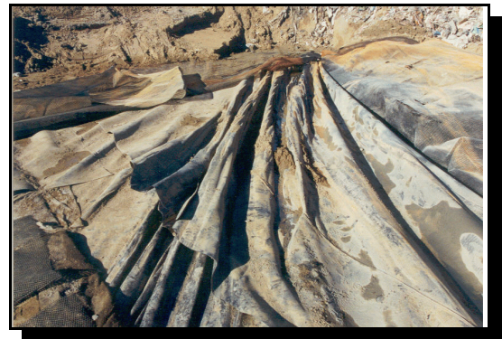
Figure 8-8 Damage to FML of an Ohio landfill at the bottom of a slope from a deep-seated translational failure involving RSL and unreinforced GCL. Contrast this with the tension crack near the top of the same slope shown Figure 8-7 .
