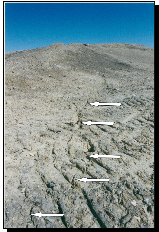
Figure 8-7 Expansion crack (marked by white arrows) that developed at the top of a slope of an Ohio landfill that had experienced a deep-seated translational failure involving RSL and unreinforced GCL. Contrast this with the damage at the toe of the same slope shown in Figure 8-8 .
