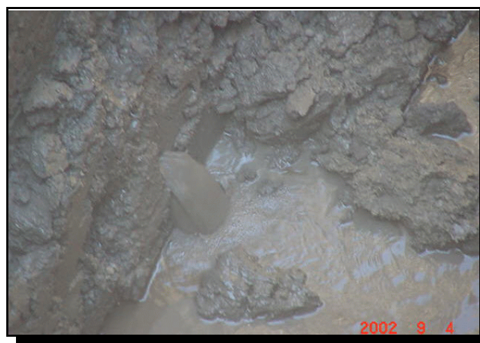
Figure 7-4 This is another example of hydrostatic pressures at an Ohio landfill creating flow through more than 20 feet of heavy in situ clay materials causing flooding of the excavation.
