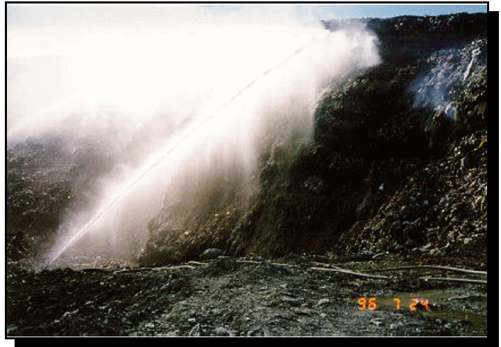
Figure 1-1 An Ohio landfill near Cincinnati experienced a massive slope failure in 1996 that resulted in 18 fires during the 9 months it took to cover the exposed waste.
