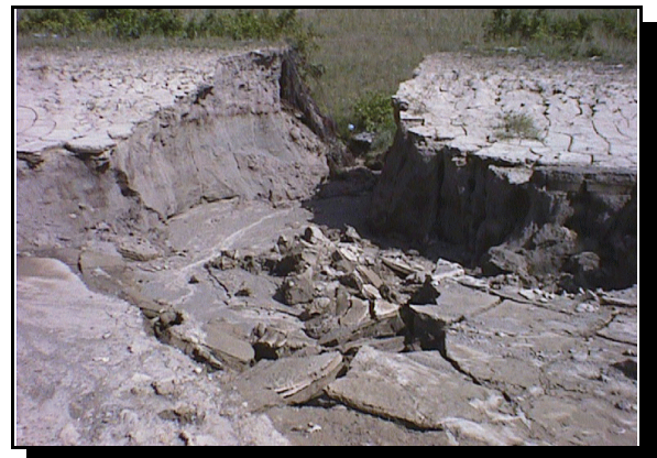
Figure 8-4 Looking through the failed containment berm of a storm water retention basin that was located in Cuyahoga County. The outlet was plugged, causing the phreatic surface in the basin to become unexpectedly high. As a result, it overwhelmed the shear strength of the soil materials used to construct the berm and caused it to collapse.
