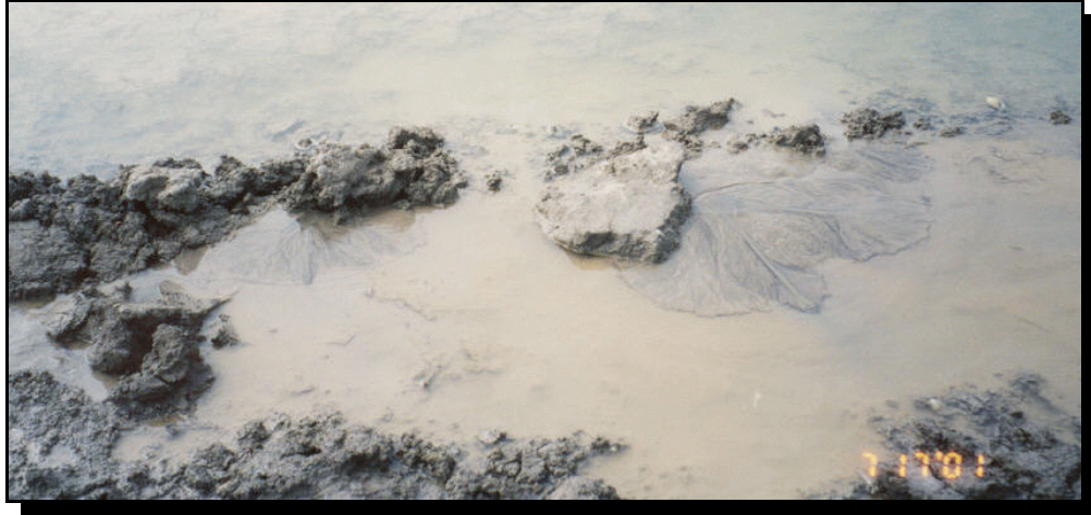
Figure 7-1 Hydrostatic pressure can cause in situ materials to fracture and allow the passage of the underlying ground water into an excavation, causing flooding of the excavation and weakening the in situ materials. Note the two delta formations in the above picture that are obvious evidence of flow through the in situ materials, which at this Ohio landfill, are over 20 feet thick.
