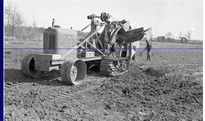
Laying subsurface drain tile with a machine. Shallow tiles and ditches were generally dug by hand. About four miles west of Dawson, Lac qui Parle County, circa 1906. (MHS photo)
