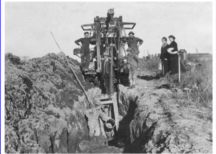
Laying subsurface drain tile with a machine. Shallow tiles and ditches were generally dug by hand. About four miles west of Dawson, Lac qui Parle County, circa 1906. (MHS photo)
