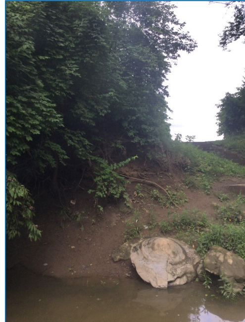
Steep, exposed banks at Mingo Park. Photo courtesy of Erin Wolfe.
