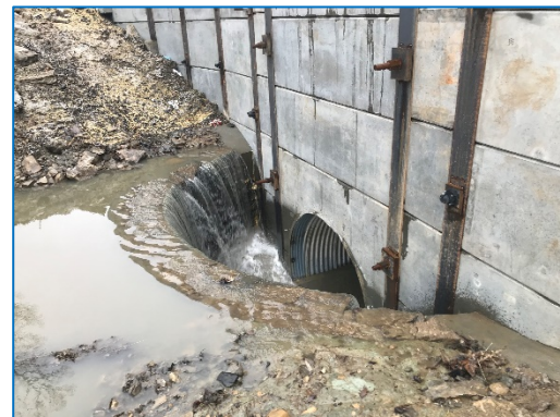
New spillway and culvert along Sugar Run
