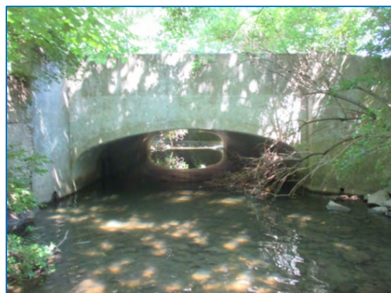
Delaware Run is highly channelized and constrained by development. Photo from E.P. Ferris and Associates, 2020.
