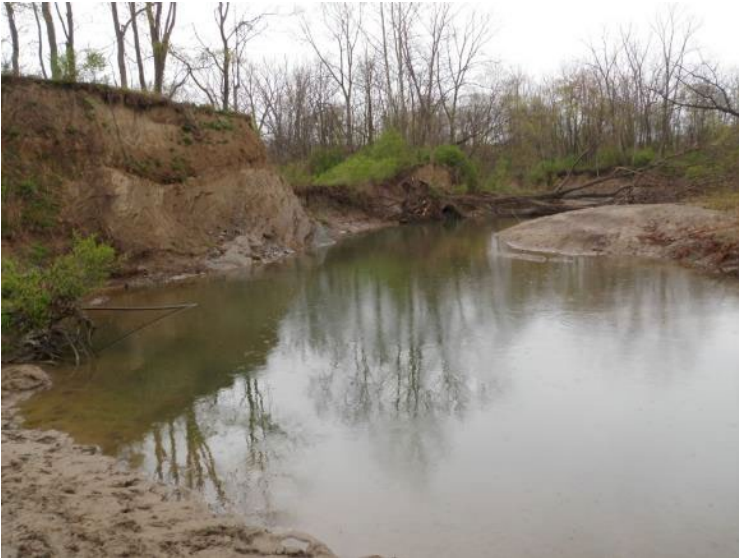
Figure 29: Streambank erosion (left bank shown) on the East Branch at RM 13.2 in the City of Kirtland. (CRWP, September 2016)
