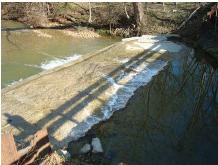
Figure 34: The Sperry Road bridge and associated silt trap are barrier to fish migration on an unnamed tributary to the East Branch (tributary enters the East Branch at RM 14.80).
