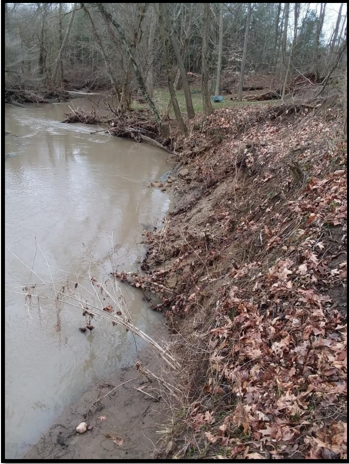
Figure 29: Common streambank erosion that can be found along the Olentangy River.
