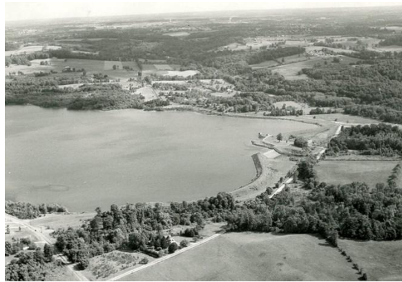
Clear Fork Reservoir Dam in 1967. Photo from the Richland SWCD website.
