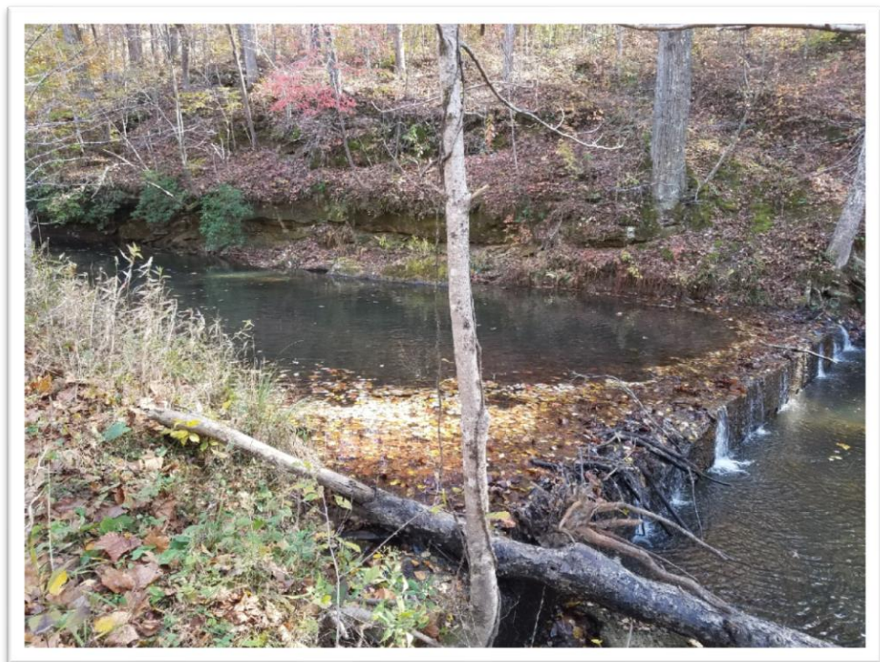
Figure 10. Slow moving pool behind the low-head dam. This structure impounds water for approximately 0.1 mile upstream. Photo Credit: Brooke Sanderson (Ohio University)
