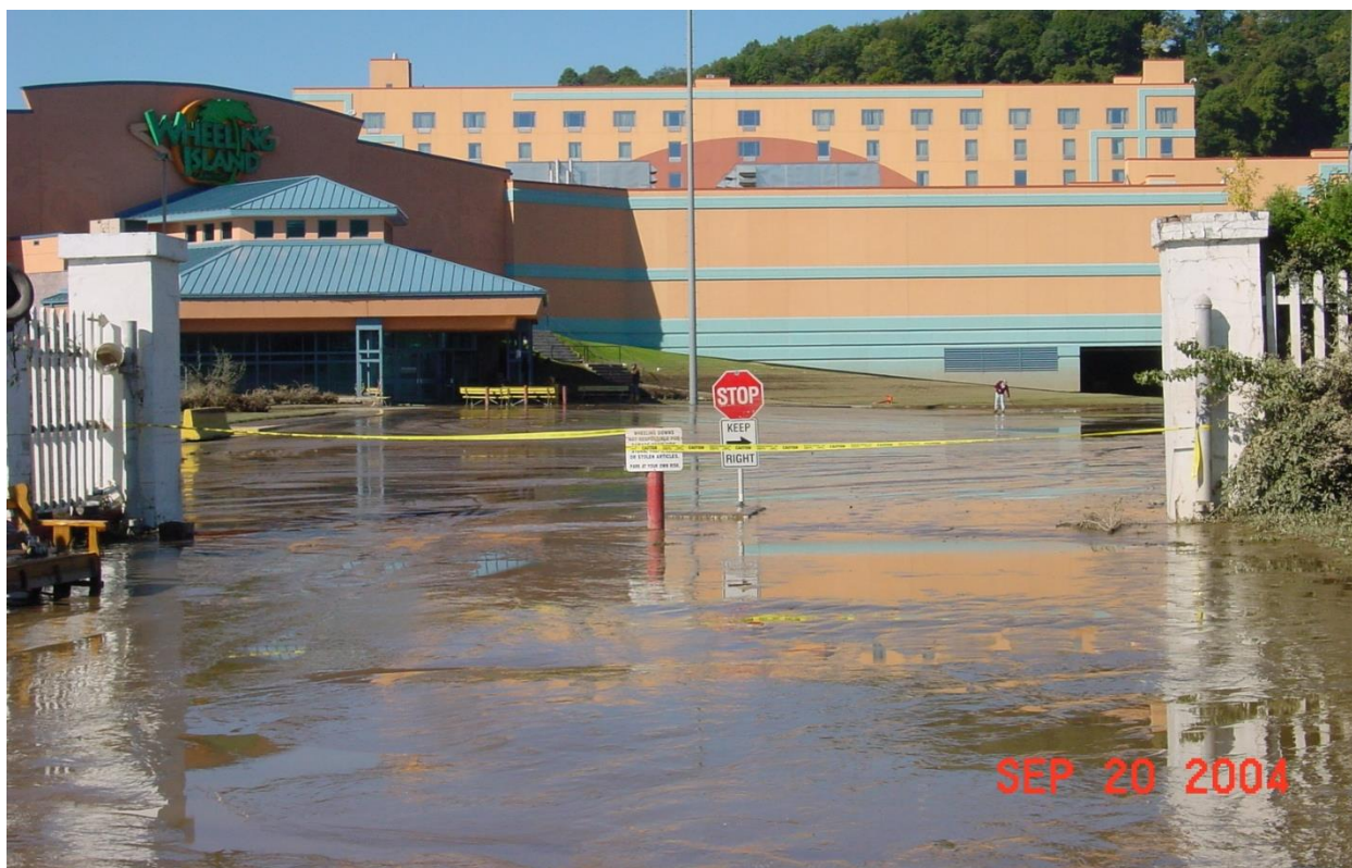
Figure 12 – Post Ohio River flooding after Hurricane Ivan in September 2004, which shows silts and clays deposited on the Wheeling Island floodplain. The pollutants attached to these silts and clays have been removed from the channel, which provides for enormous water quality benefits.
