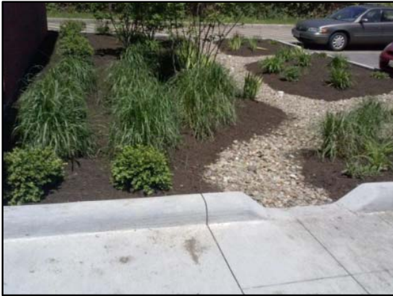
Planted bioretention area with sidewalk curb cut in foreground. Stormwater runoff is conveyed through gravel to shallow depression of bioretention area. Credit: Northeast Ohio Regional Sewer District
