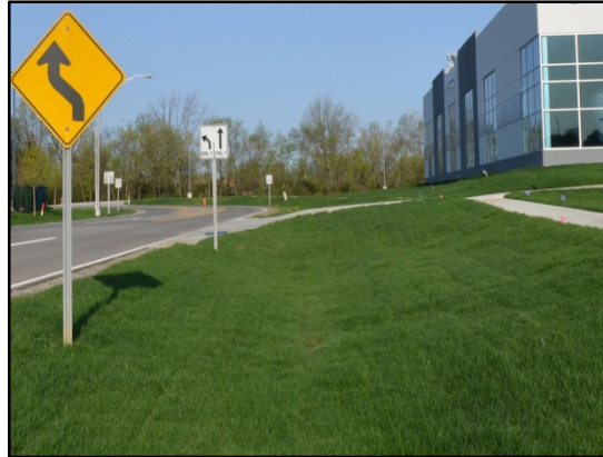
Maintained turf grass protects underlying specialized soils from erosion and slows flow through the swale. Credit: Ohio Department of Natural Resources Division of Soil & Water Resources.
