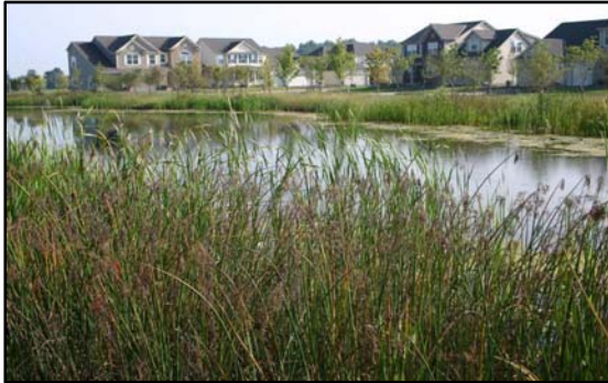
Wet pond with maintained shoreline containing aquatic bench for wetland vegetation to improve pollutant removal. Credit: Ohio Department of Natural Resources Division of Soil & Water Resources.
