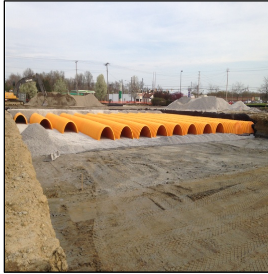
Open-bottom underground detention pipe segments awaiting installation into gravel backfilled storage layer. Credit: StormTech a Division of ADS, Inc.
