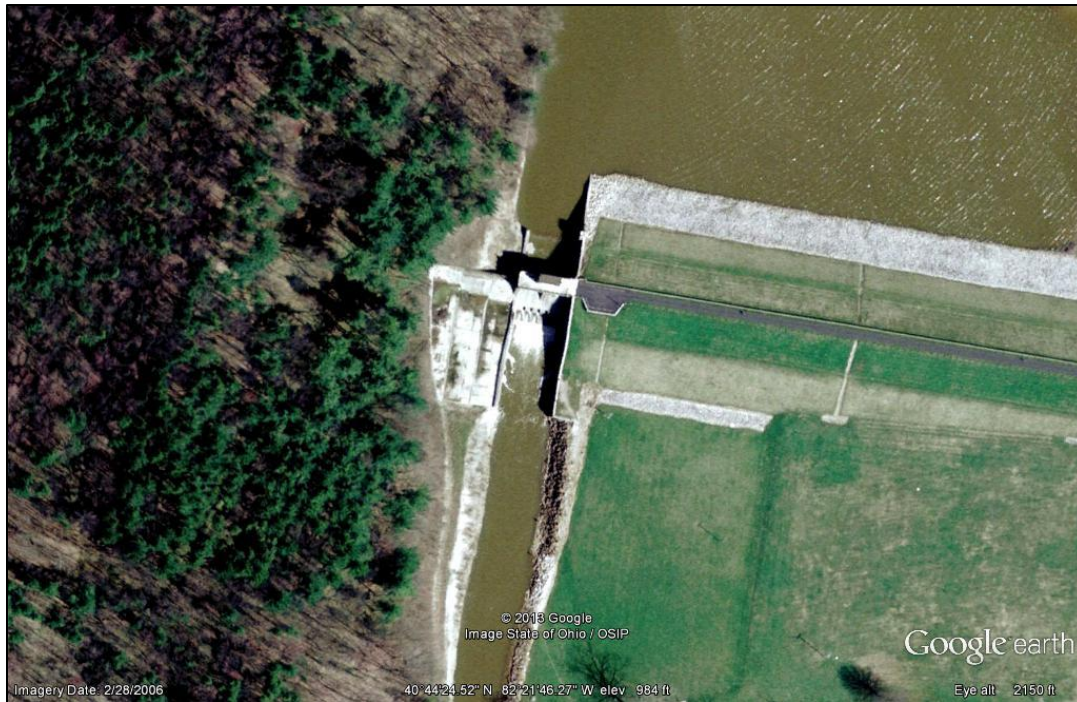
Figure 4-3. Charles Mill Dam – shows bottom discharge.
