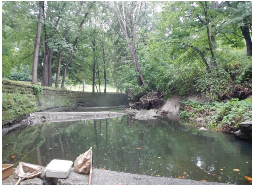
Figure 10. Doan Brook, RM 2.27, upstream view. Throughout this reach, Doan Brook is a concrete lined and channelized with a series of dams. Like all the streams sampled in Cuyahoga County, legacy sediment contamination, CSOs, habitat alteration, and urban runoff severely impact the macroinvertebrate community in this watershed.
