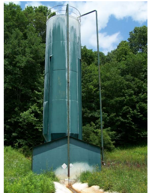
Figure 9 — Carbondale calcium oxide doser, courtesy of Amy Mackey, Raccoon Creek Partnership Watershed Coordinator
