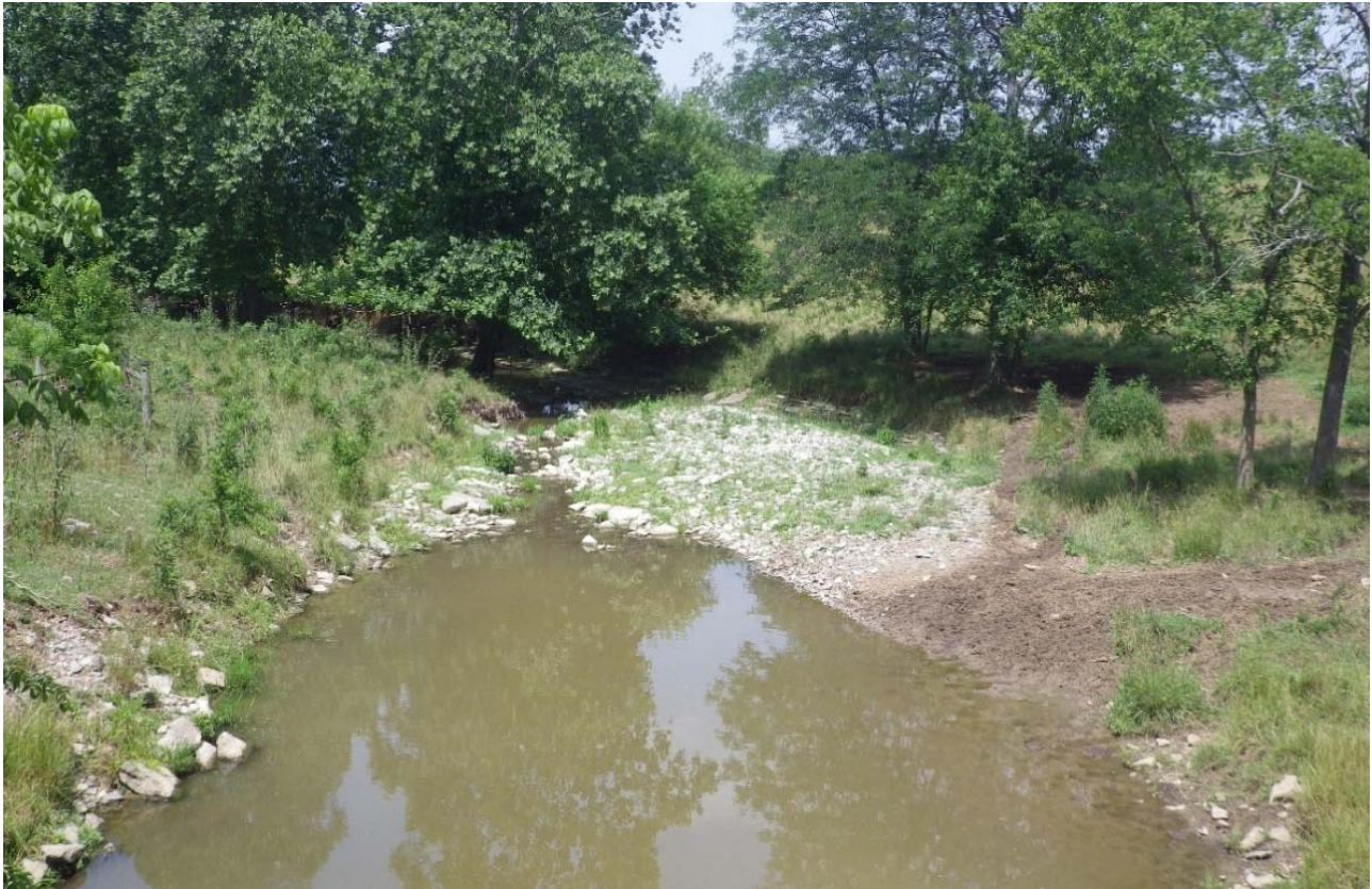
Figure 13 — Illustrated above is a well-used path to Redoak Creek from instream livestock watering which contributes to erosion and siltation. Out of stream livestock watering is encouraged where possible.
