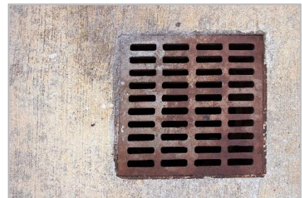
Label floor drains and consider having them capped or plugged if not in use.
