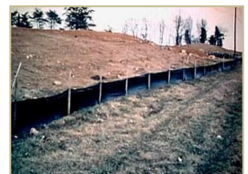
A silt fence can help keep sediment from running into nearby waterways.
