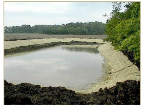
A sediment pond is effective in helping to control contaminated runoff.
