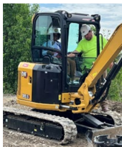
(Left to right) ApprenticeOhio Team Member Traci Carter tried her hand at excavating during Construction Career Days.
