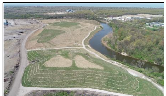
Figure 9. Reclamation Site after construction.
