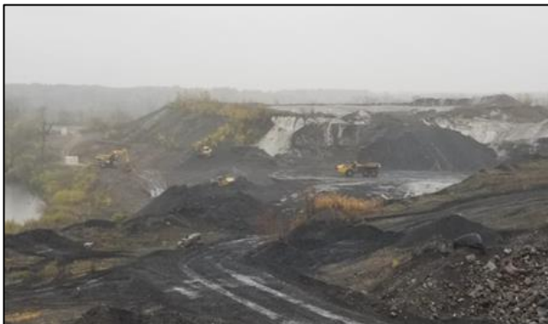
Figure 8. Reclamation Site during capping.
