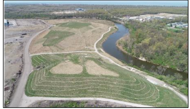
Figure 7. Reclamation Site after construction
