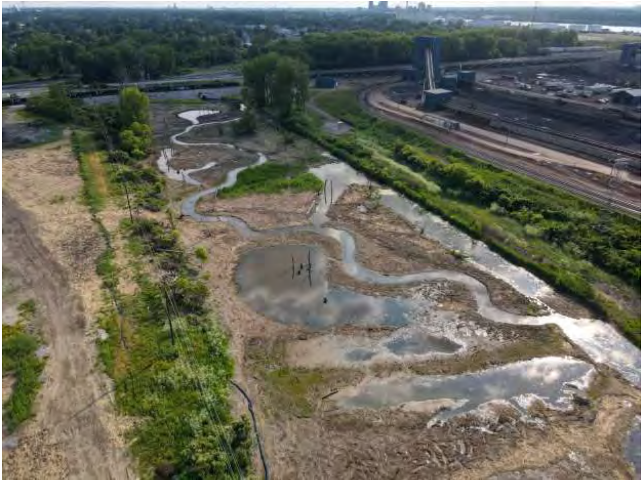
Figure 134. Post-construction (June 2023) aerial image of the Duck and Otter Creek Project wetland, depicting the reconfigured meandering natural channel and wetland pools. Photo credit: EnviroScience.
