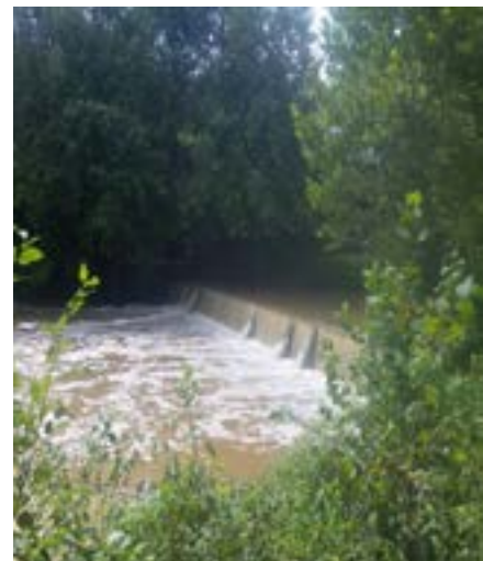
Vinton Dam located at river mile 40.3.
