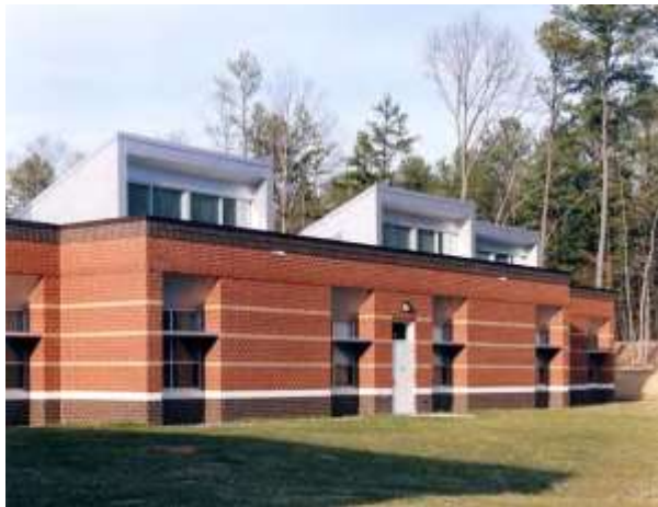
a) South-facing daylighting roof monitors
