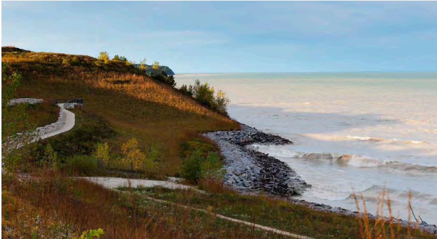
Bluffs may be stabilized with deep-rooted native vegetation that provides habitat benefits and improves visual connections between top-of-bluff areas and the lake. These restored and stabilized bluffs are not incompatible with public access; they may be shaped and locally retained to provide fully-accessible pathways despite their steepness and height.
