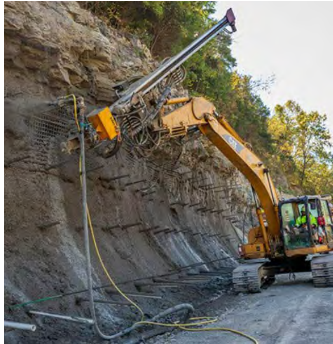
Gunite applied to the face of the bluff.
