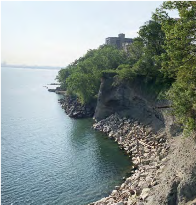
Bluff toe protection (revetment) mitigates wave erosion at base of the bluff, preventing undermining of the bluff face and resulting slides and collapses.
