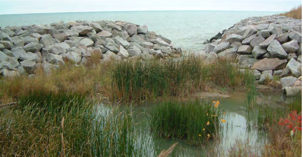
Revetments may be used to create stormwater treatment areas. These green infrastructure best practices add ecological complexity to the shoreline.
