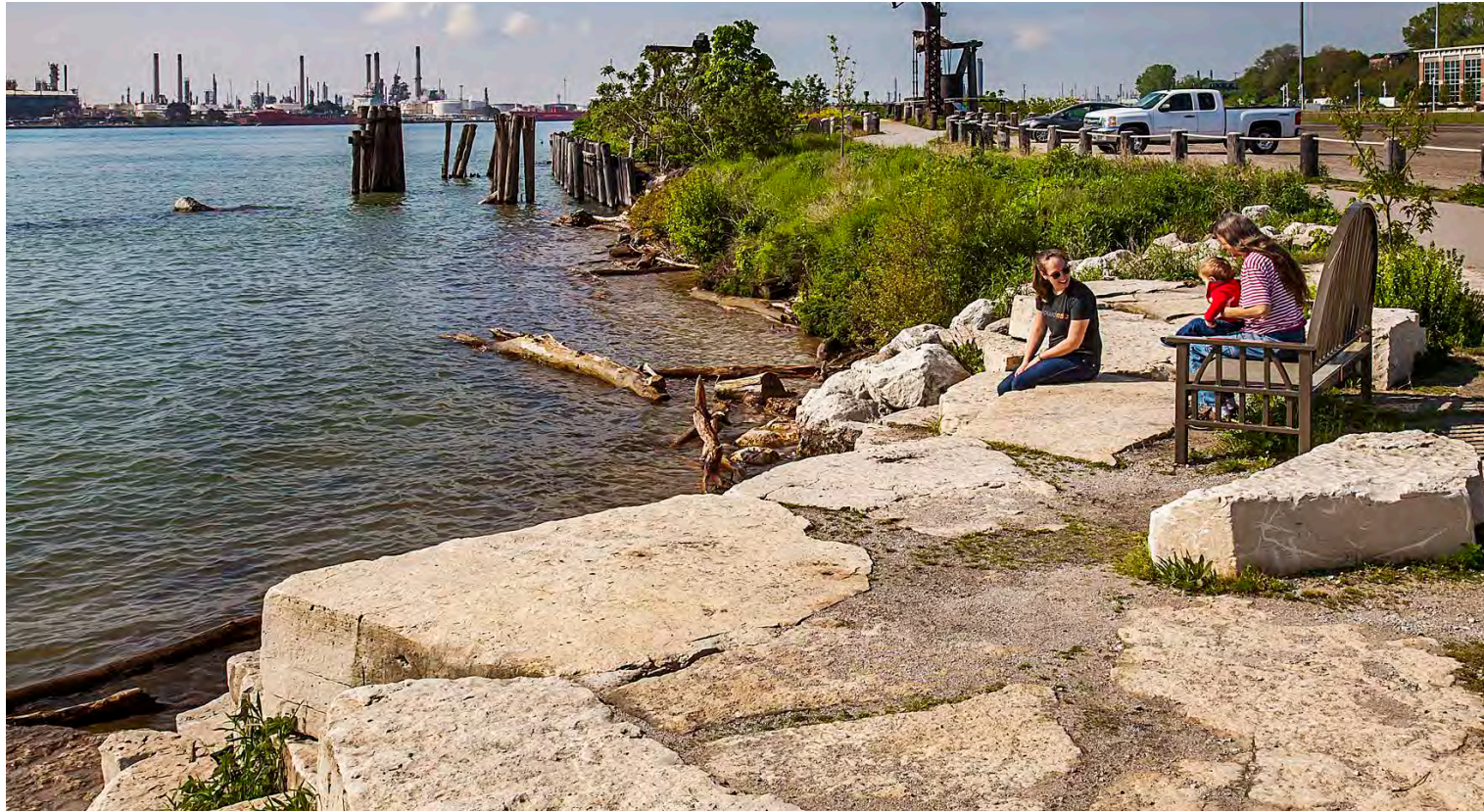
While pathways and revetments are necessarily located high above Lake Erie's typical water level, stepped revetments and accessible lakeshore edges provide opportunities for direct lake access.
