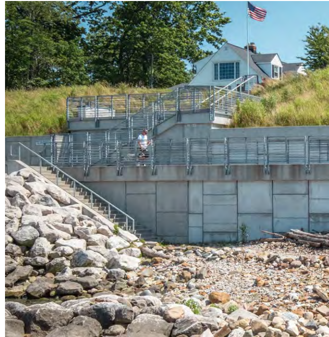
Where required, retaining structures may be utilized to stabilize bluffs without impacting existing top-of-bluff improvements.
