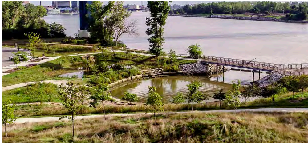
Off-site and site-adjacent stormwater can be treated in stormwater cells that functionally and visually extend lakeshore pockets and beaches.
