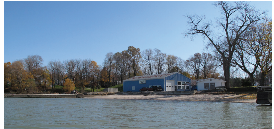
The west jetty Cranberry Creek Marina is shown at the left. The beach present west of the jetty is bounded by a groin seen at the above photo's far right.
