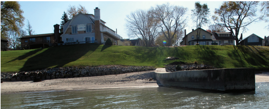
A revetment is at landward of the beach along the toe of the regarded bluff.
