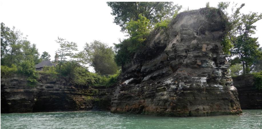
The breakwaters at Miller Road Park and the Avon Lake power plant help stabilize the beach along the shore between the structures (top and middle). The shore of Avon Point consists of shale bluffs along several small headlands separated by narrow embayments (bottom).
