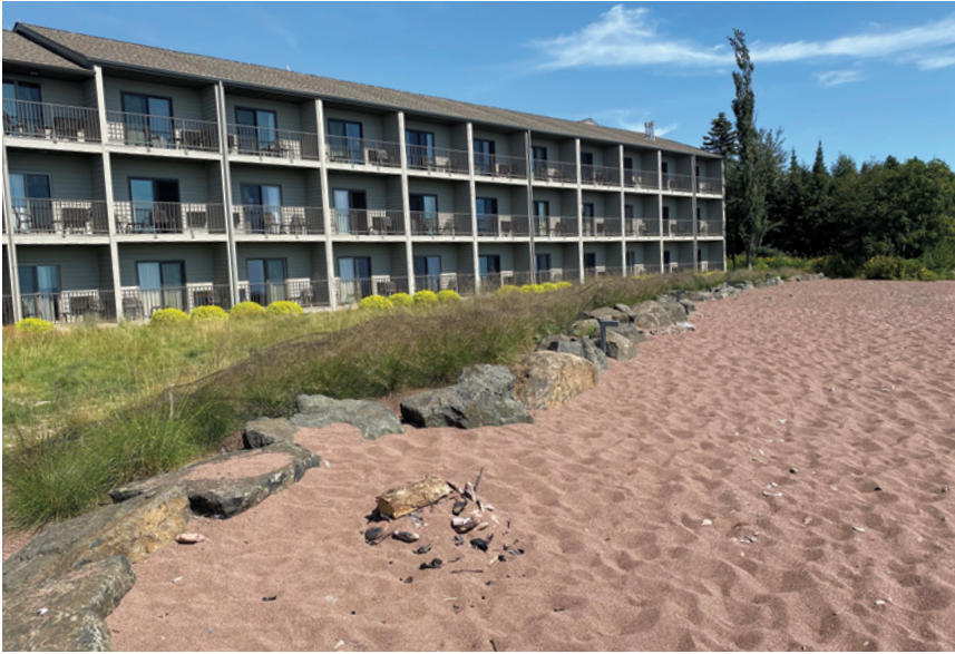
Rock edging used to protect upland vegetation from waves and the overwash of beach sand into the vegetation on Lake Superior in Grand Marais, Minn. Melanie Perello
