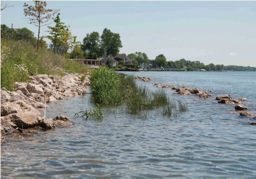
After – High Water At high water levels the marsh may be completely submerged. In this case the sill will dissipate some wave energy and stone edging will provide protection to the shoreline. Michigan Department of Environment, Great Lakes, and Energy
