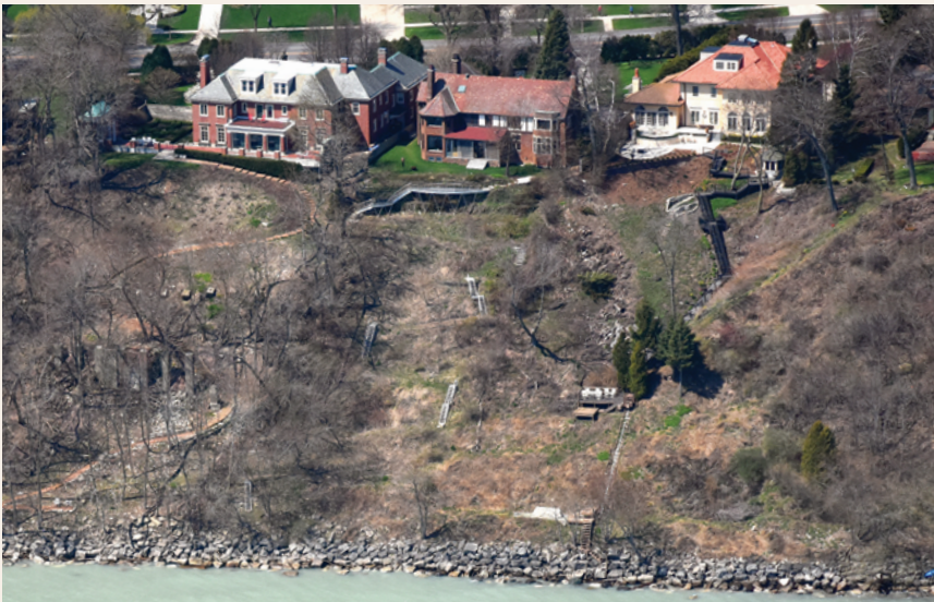
After Oblique aerial image (2019) of the stabilization project with the vegetated terrace wall and new staircase near the residence, as well as a revegetated bluff face. Capt. Dennis Carr
