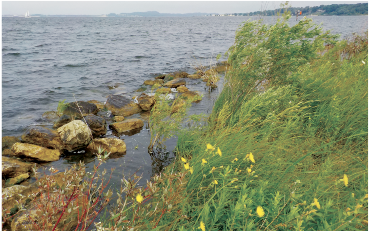
A rock sill built near the Center Point Bay Marina in Muskegon Lake, Mich. Brian Majka
