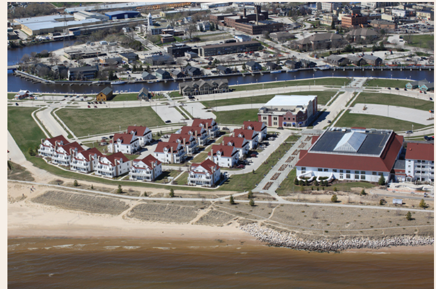
After Nourishment – Low Lake Levels (2012) The beach and buried revetment (left half of shoreline in image) several years after the nourishment project. USACE
