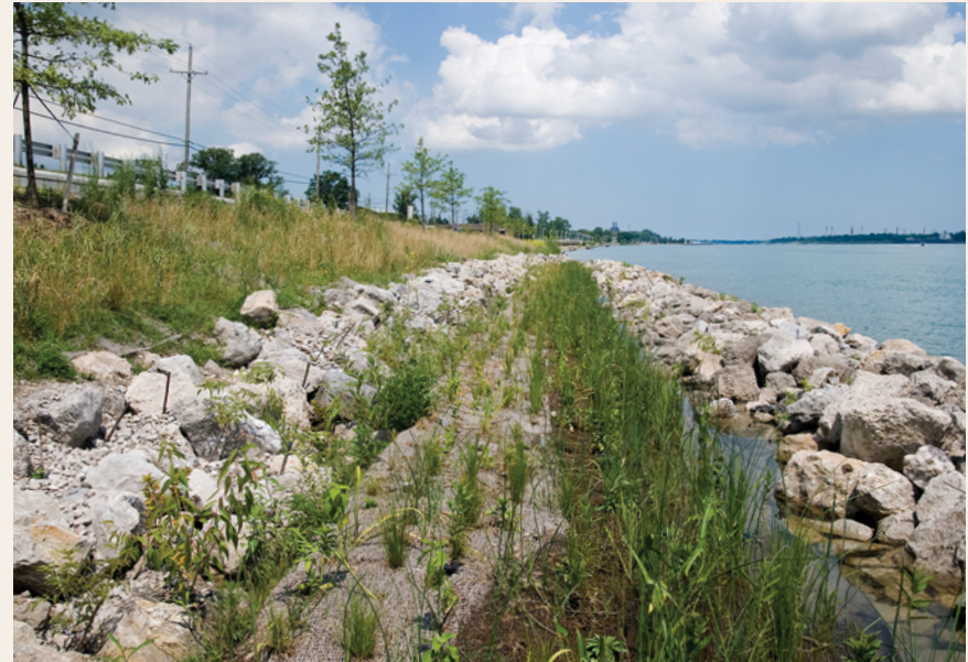
After – Low Water The area was protected by a sill with marsh vegetation. New vegetation was also planted along the shore. At low water levels, the marsh may be above the water line and the sill is emergent. Michigan Department of Environment, Great Lakes, and Energy
