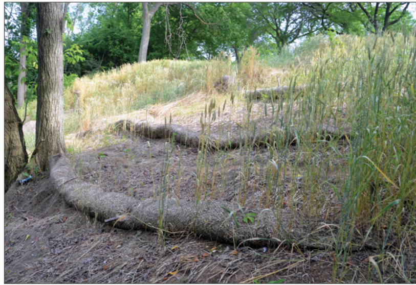
Coir logs staked into the bluff to slow surface water flow down the bluff face and help vegetation establish. Lydia Salus
