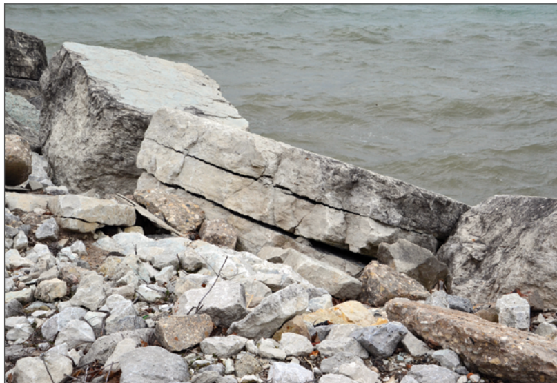
TOP Displaced armor stone has exposed the underlying filter layer to wave forces. Adam Bechle BELOW Cracked armor stone has split into smaller pieces. Adam Bechle
