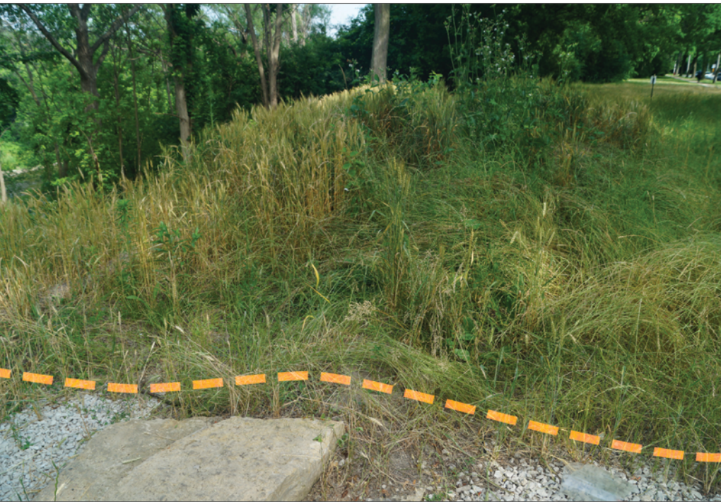
LEFT A small, vegetated berm prevents runoff from flowing over the bluff-top edge. Land surface profile is represented by the dashed line showing the berm rising slightly near the slope edge. Lydia Salus CENTER Rock spillway to take runoff to the base of the bluff without eroding bluff face soils. Adam Bechle RIGHT Surface runoff drainage pipe has become disconnected in multiple locations, depositing flows of water to the middle of the bluff rather than the base of the bluff. Adam Bechle
