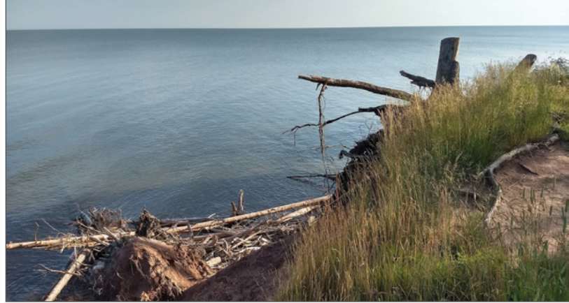
A tree cut down near the bluff-top edge reduces weight on the bluff. Adam Bechle
