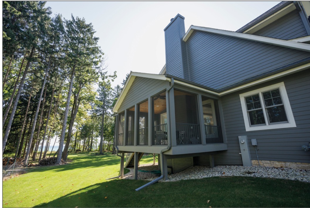
Downspout draining away from bluff-top edge. Sara Stathas
