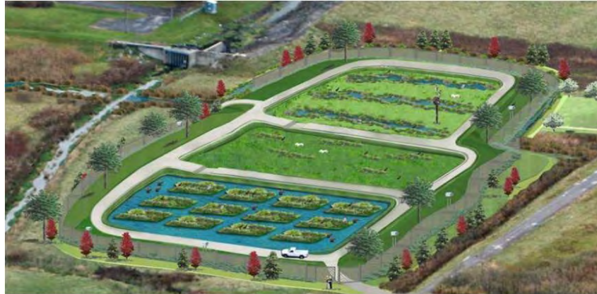
Harbor Brook CSO Treatment Wetland Photo: Onondaga County 'Save the Rain'
