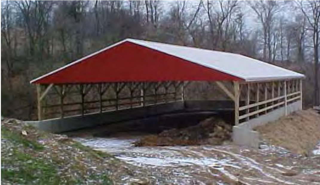
Animal Waste Storage Facility
