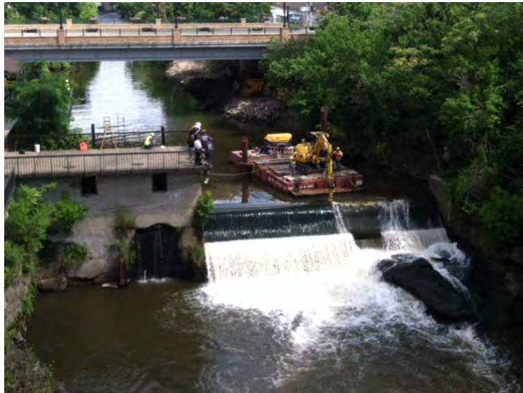
Dam Removal – Cuyahoga Falls Photo: ODNR
