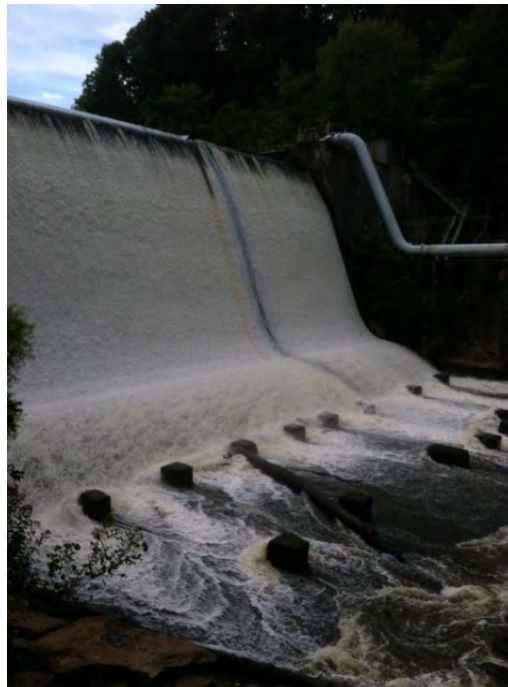
Gorge Dam - Cuyahoga Falls (Former Hydroelectric Dam) Photo: ODNR
