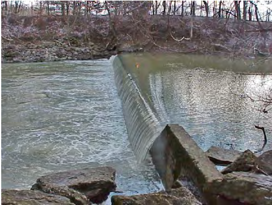
Former Coho Dam – Huron, Ohio Photo: ODNR
