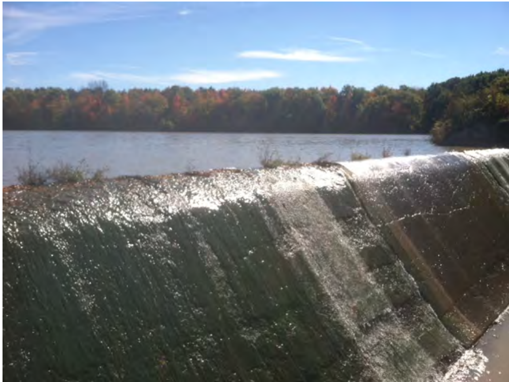
Dam spillway at Van Buren State Park Photo: ODNR
