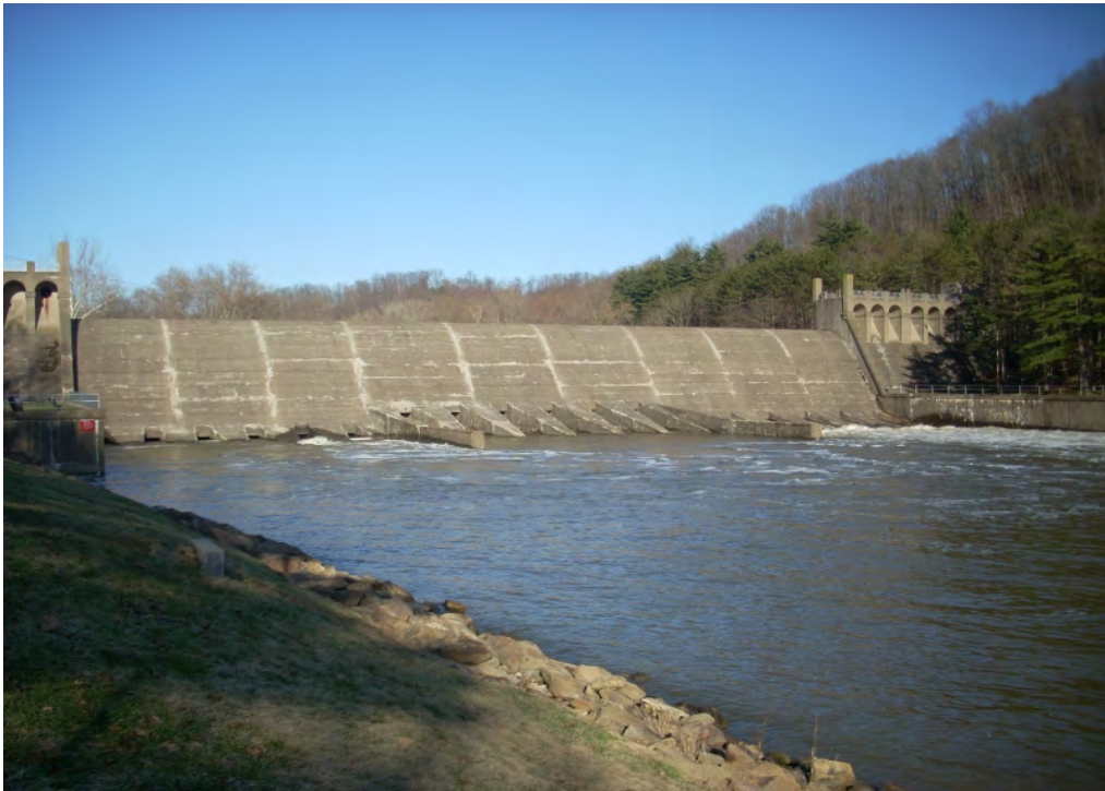
Dover Flood Control Dam Photo: Muskingum Watershed Conservancy District
