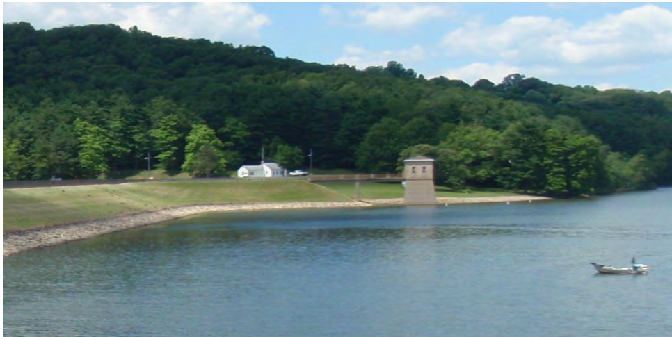
Leesville Lake Dam Photo: Muskingum Watershed Conservancy District
