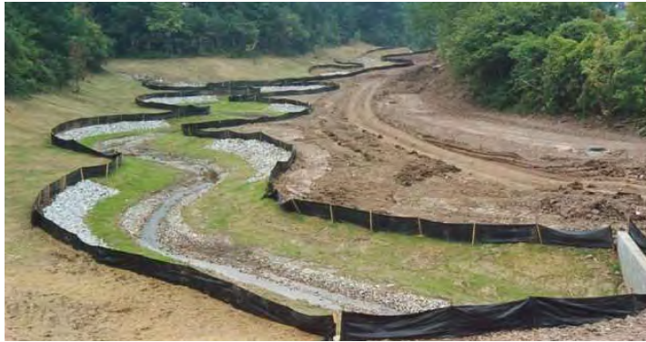
Silt Fence/Vegetative Cover Photo: Armtec Infrastructure Inc.
