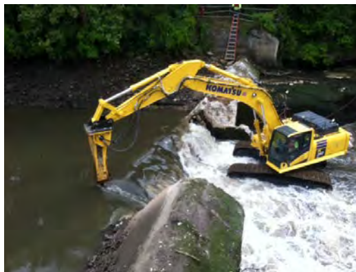
Lowering of water levels upstream of Lefever Dam
