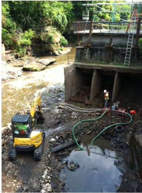
Removal of Sediment/Debris Photo: Ohio DNR
