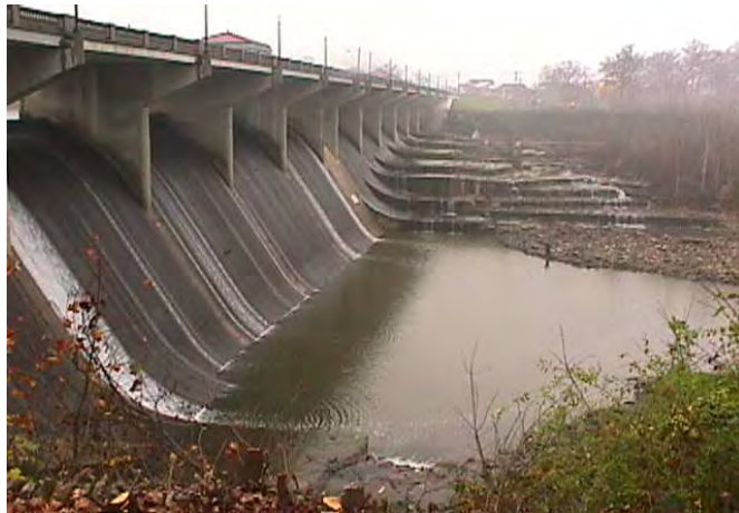
The O'Shaughnessy Dam on the Scioto River near Columbus Photo: ODNR
