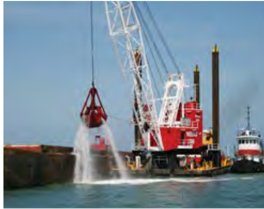
Dredge with Clamshell bucket
