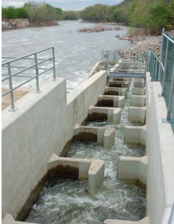
Vertical Slot Fish Ladder
