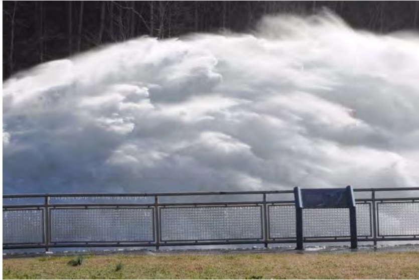
Water Release from Dam
