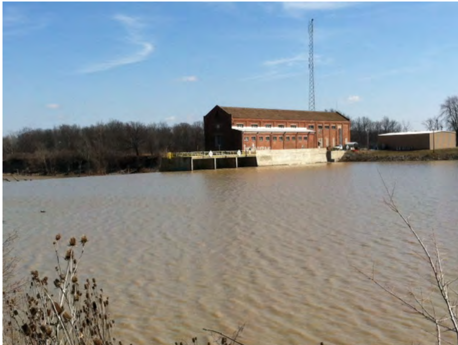
Defiance Hydroelectric Power Dam Photo: Ohio DNR
