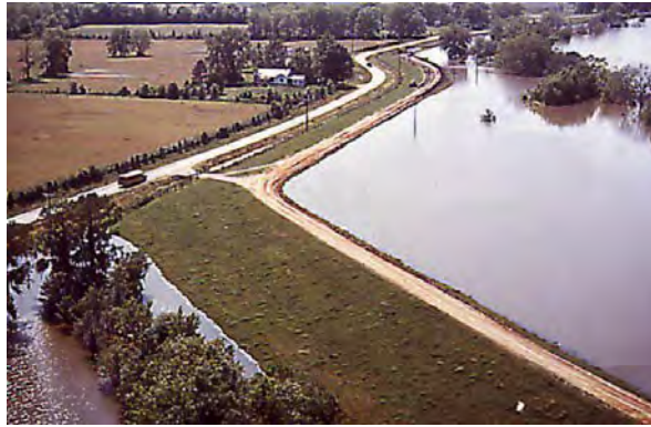
Flood Control Levee Photo: US Army Corps of Engineers
