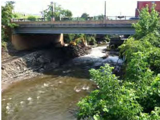
Access road constructed under bridge
