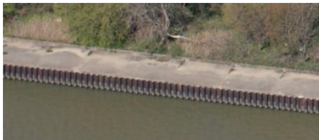
SEAWALLS AND BULKHEADS ARE RETAINING WALLS THAT STABILIZE THE SHORE AND PROVIDE ACCESS TO THE WATER FROM THE SHORE. PHOTO CREDIT: U.S. ARMY CORPS OF ENGINEERS GREAT LAKES OBLIQUE IMAGERY (GREATLAKES.USACE.ARMY.MIL)
