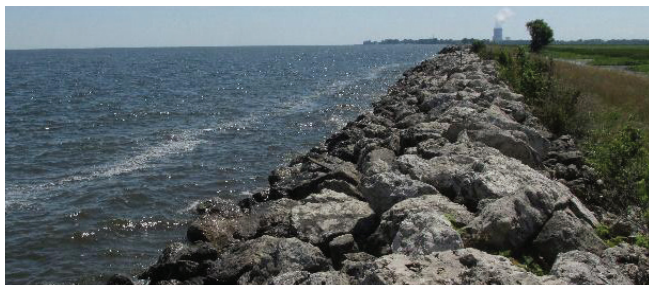
REVETMENTS ARE BUILT OF STONE THAT VARIES FROM THE SIZE OF A SUITCASE TO THE SIZE OF A CAR. THESE BOULDERS ARE LAID ALONG THE SHORE ABOVE AND BELOW THE WATER. PHOTO CREDIT: PRABHA RUPASINGHE, BGSU
