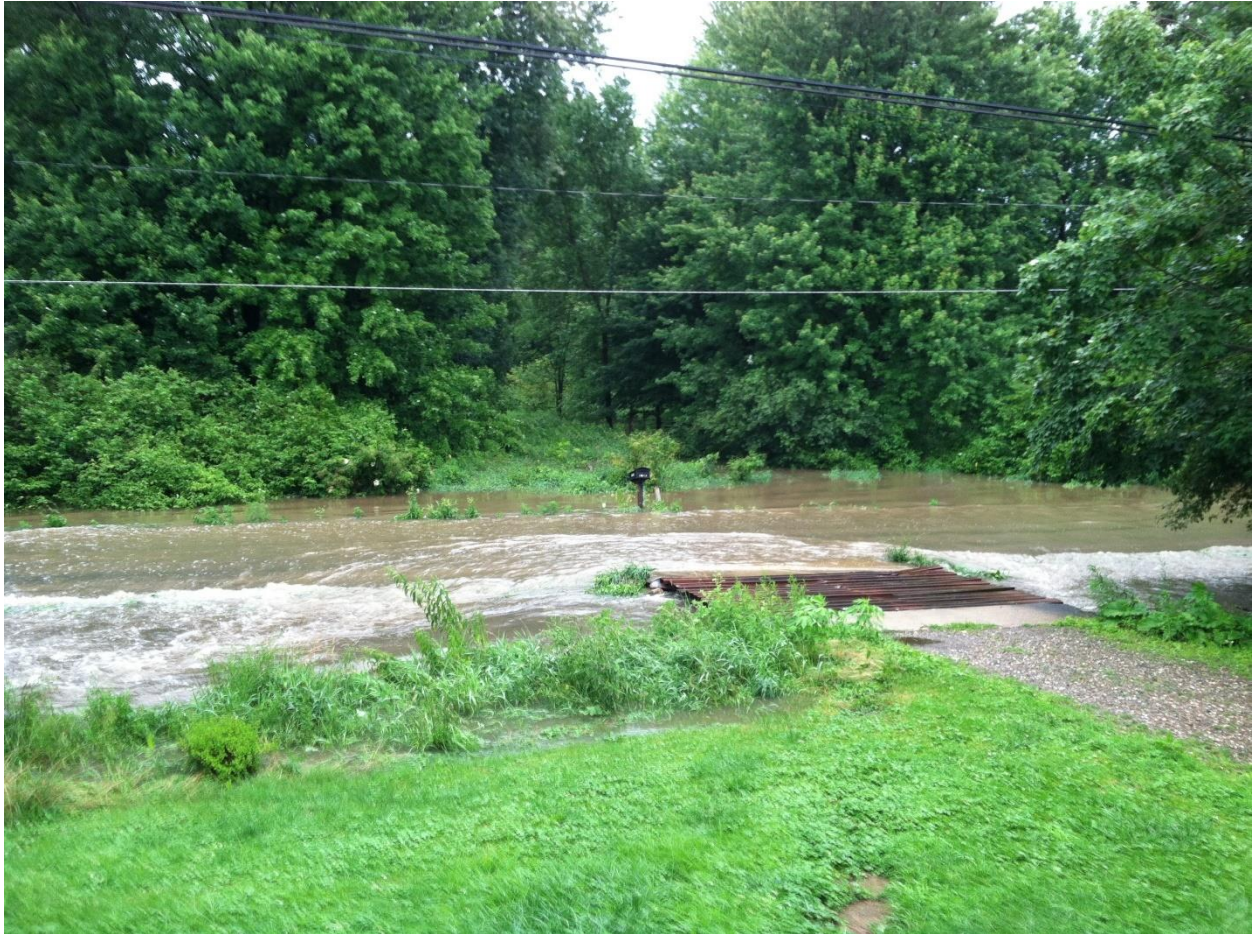
Figure 9: Overflowing ditches along Mantua Center Road. Photo taken July 11, 2013 by resident.
