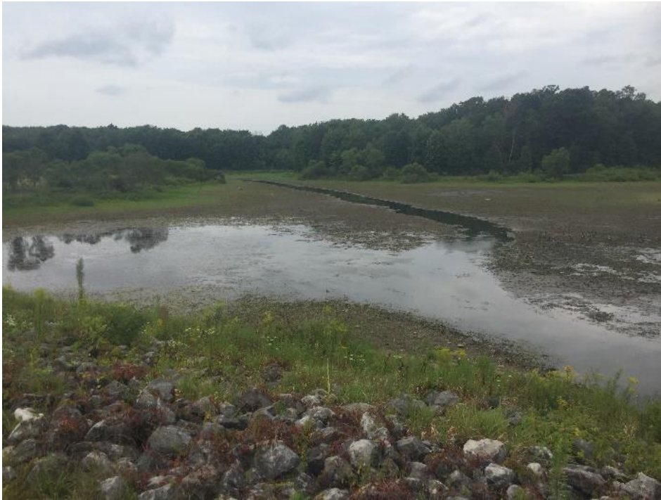
Figure 15: City of Akron property north of Black Brook dike. August 17, 2017. Photo by Alicia Beattie.
