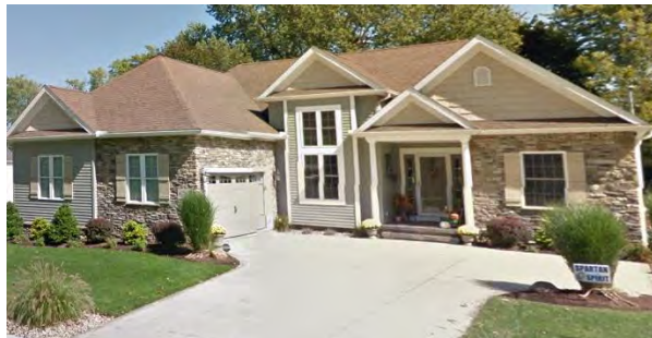
New Housing Construction
