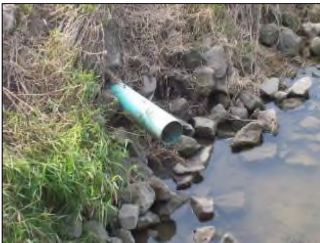
Figure 27. Tile drain along Pipe Creek.
