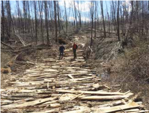
Figure 40. Sawmill slabs used to armor a forwarder trail.
