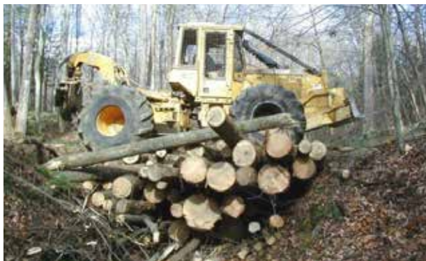
Figure 27. Temporary pole crossing used to cross an ephemeral drainage.
