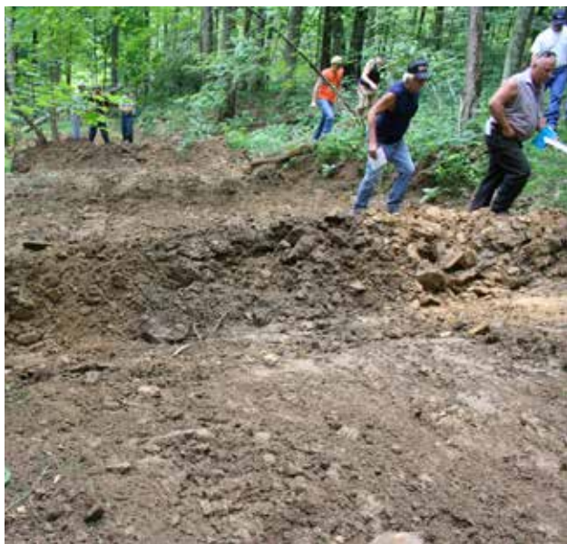
Figure 23. Water bars for water diversion.
