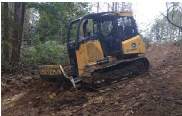
Figure 29. A dozer addressing maintenance issues on a skid trail.
