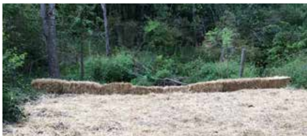
Figure 5. An effective straw bale barrier.
