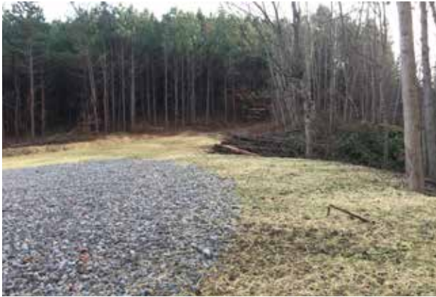
Figure 34. A properly closed log landing with vegetation established. Note the water bar to divert runoff from the approaching skid trail. Landings such as this are a low risk for environmental issues and promote a positive image of the forest industry.
