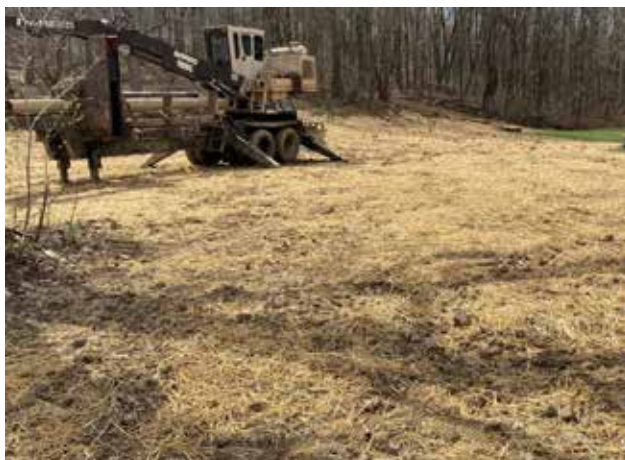
Figure 37. Properly installed mulch on new seeding.
