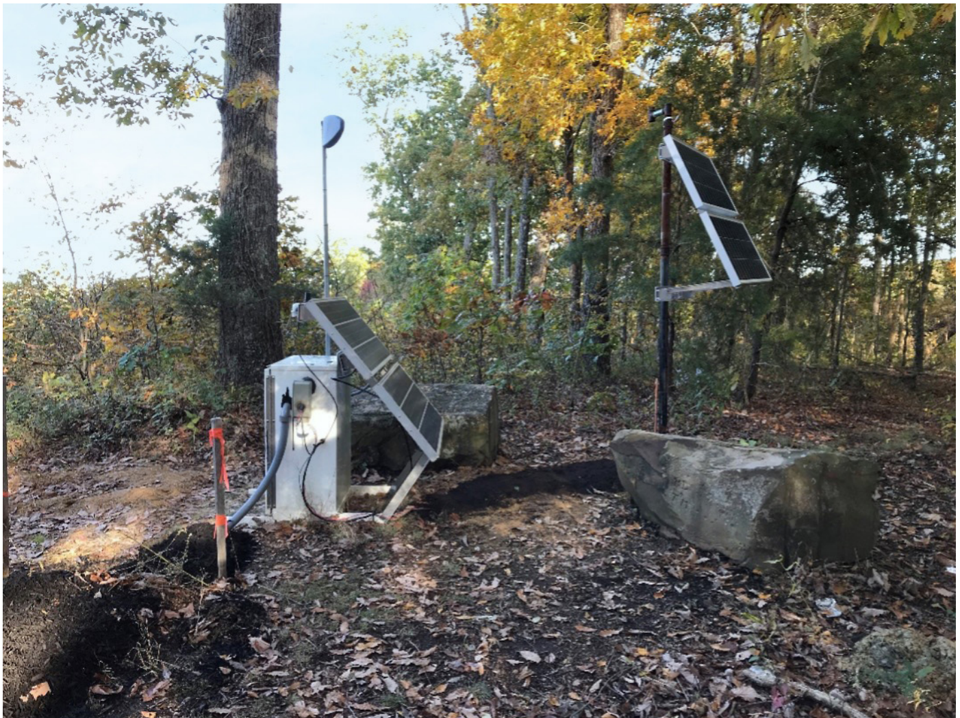
FIGURE A-2. OhioSeis seismic station SSF2 (formerly station SSFO) at its new location in Shawnee State Forest.
