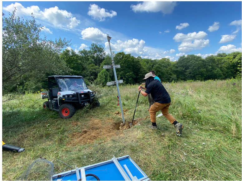
FIGURE A-6. Disassembly and removal of OhioSeis/TA station P52A.
