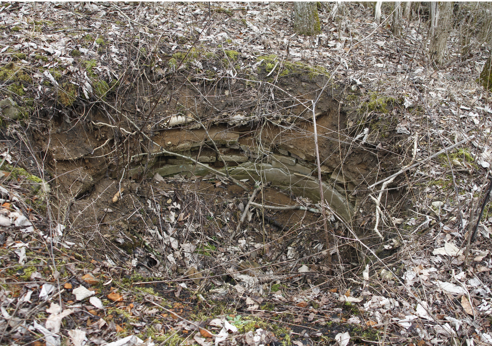
FIGURE 7. An old collapsing well unrelated to karst in Butler County, Ohio.
