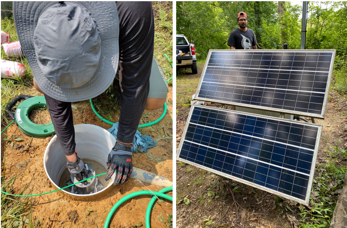
FIGURE A-9. Photos of field work being performed at two OhioSeis stations in 2023. Left: OhioSeis intern installing seismometer in new vault at station SROH (Shade River State Forest) in Meigs County, Ohio. Right: OhioSeis intern performing maintenance at station SSF2 (Shawnee State Forest) in Scioto County, Ohio.
