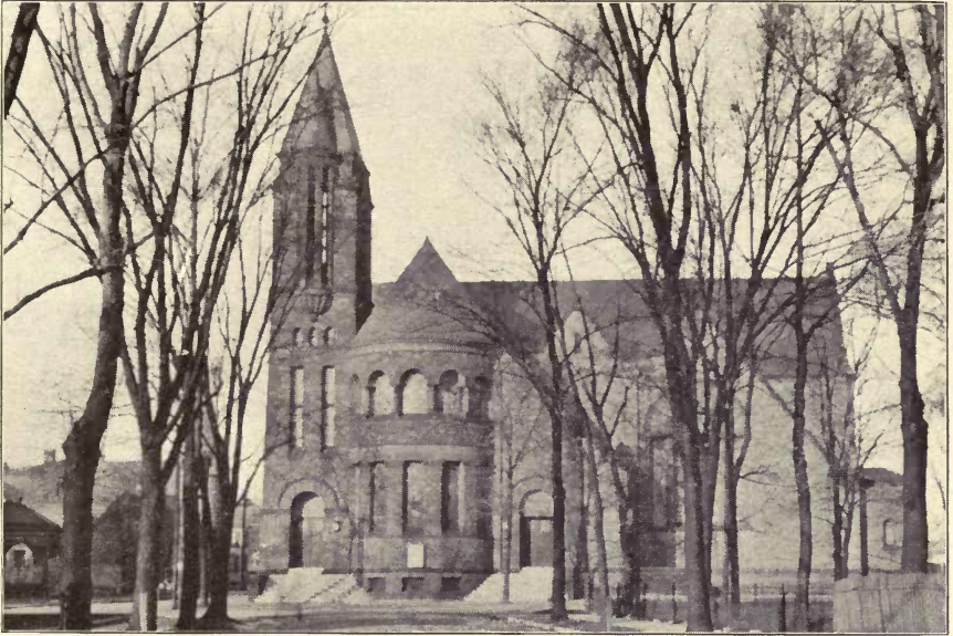
A.—Broad Street Presbyterian Church, Columbus. Built of Conemaugh sandstone from Tippecanoe, Harrison County and Sherrodsville, Carroll County. The brown sandstone trimming is from Holmes County, Ohio, and the south shore of Lake Superior. Photograph by T. M. Hills.
