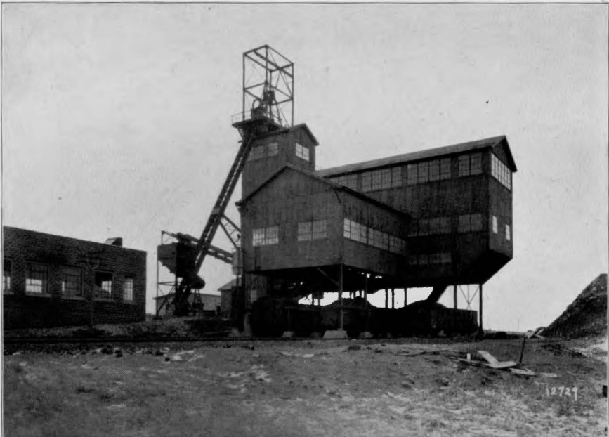
B—A coal tippie in Belmont County. The coal is raised from the mine and after screening loaded directly into the cars. (Courtesy the Jeffery Mfg. Co.)
