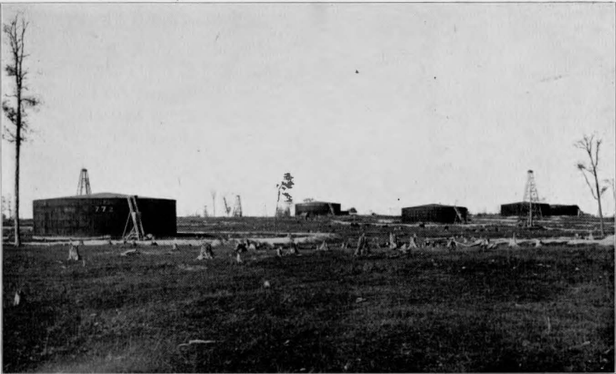
B—A tank farm in Fairfield County. In regions of oil production long lines of huge tanks are erected to store the oil from the wells. From here it is pumped to the refineries.
