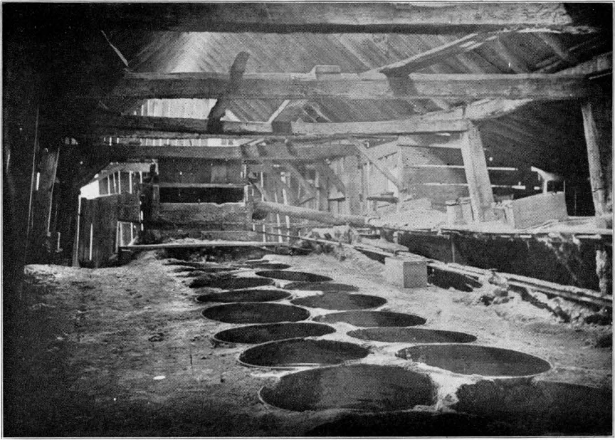
A—An old salt furnace in Morgan County. This shows the kettles used in evaporating the brine. (Photo by Bownocker)
