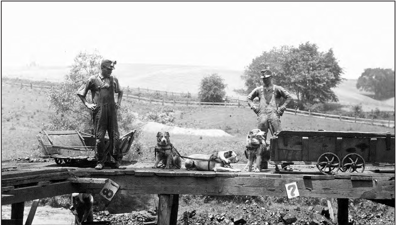
FIGURE 97.—Three dogs hitched in tandem at a Middle Kittanning (No. 6) coal mine on the property of Lewis Fisher in Wayne Township, Muskingum County (see Hansen, 1990, p. 1). Ohio Division of Geological Survey file photo taken by Wilber Stout in 1917.
