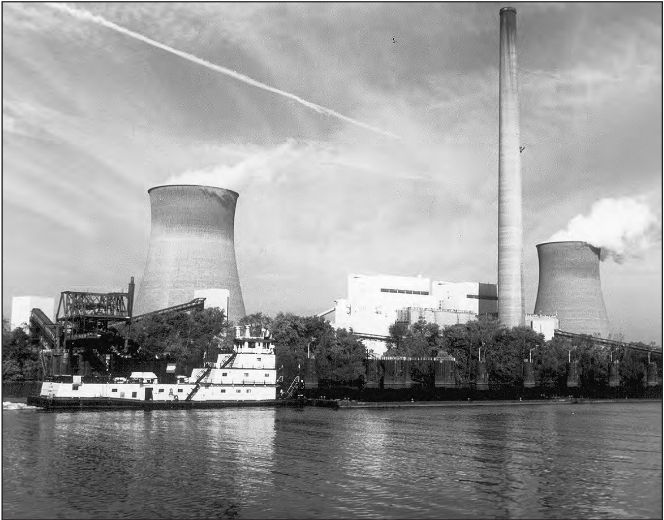
FIGURE 216.—The Gen. James M. Gavin power-generating station on the Ohio River at Cheshire, Gallia County, began service in 1974 and is the largest electricity-generating station in Ohio; generating capacity is 2.6 million kilowatts. Most of the fuel consumed by this generating station comes by conveyor from the Southern Ohio Coal Company Meigs Division underground mine complex (Meigs No. 2 and No. 31 mines, Ms-294 and Ms-293). The remaining fuel is delivered by rail or river barge (foreground). Circa 1990. Photo courtesy of American Electric Power Service Corporation. (See also figs. 46, 201, 219.)
