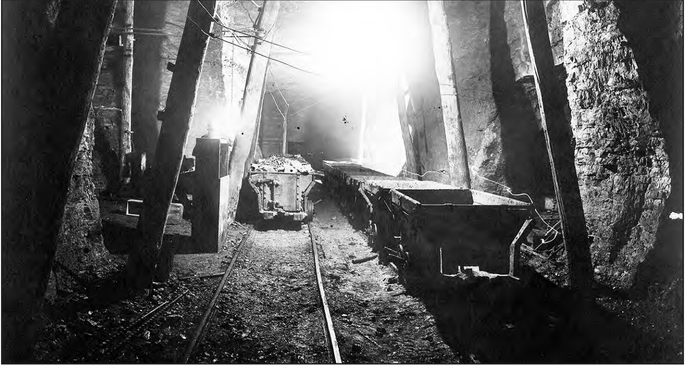
FIGURE 105.—The inside of a typical turn-of-the-century coal mine in southeastern Ohio (possibly near Shawnee or New Straitsville). Note the poor lighting, the height of the entry in comparison to the coal cars, and the wooden roof-support timbers. Ohio Division of Geological Survey file photo.
