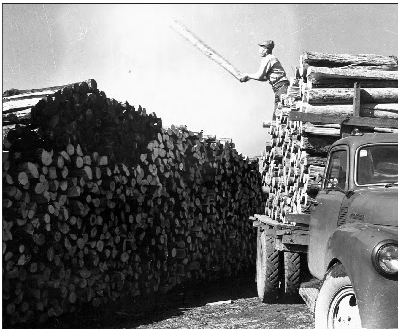
FIGURE 110.—An employee of the Hanna Coal Company Willow Grove No. 10 mine busily stacking timbers to be used as roof support in the mine. As this man unloads the truckful of timber, he probably wishes the stack of timber would last longer than half a week! Circa 1937. Photo courtesy of Dale Davis. (For other photos of this mine see figs. 35, 79, 82, 93, 117, 119, 120, 123, 140-142, 153, 154, 193.)
