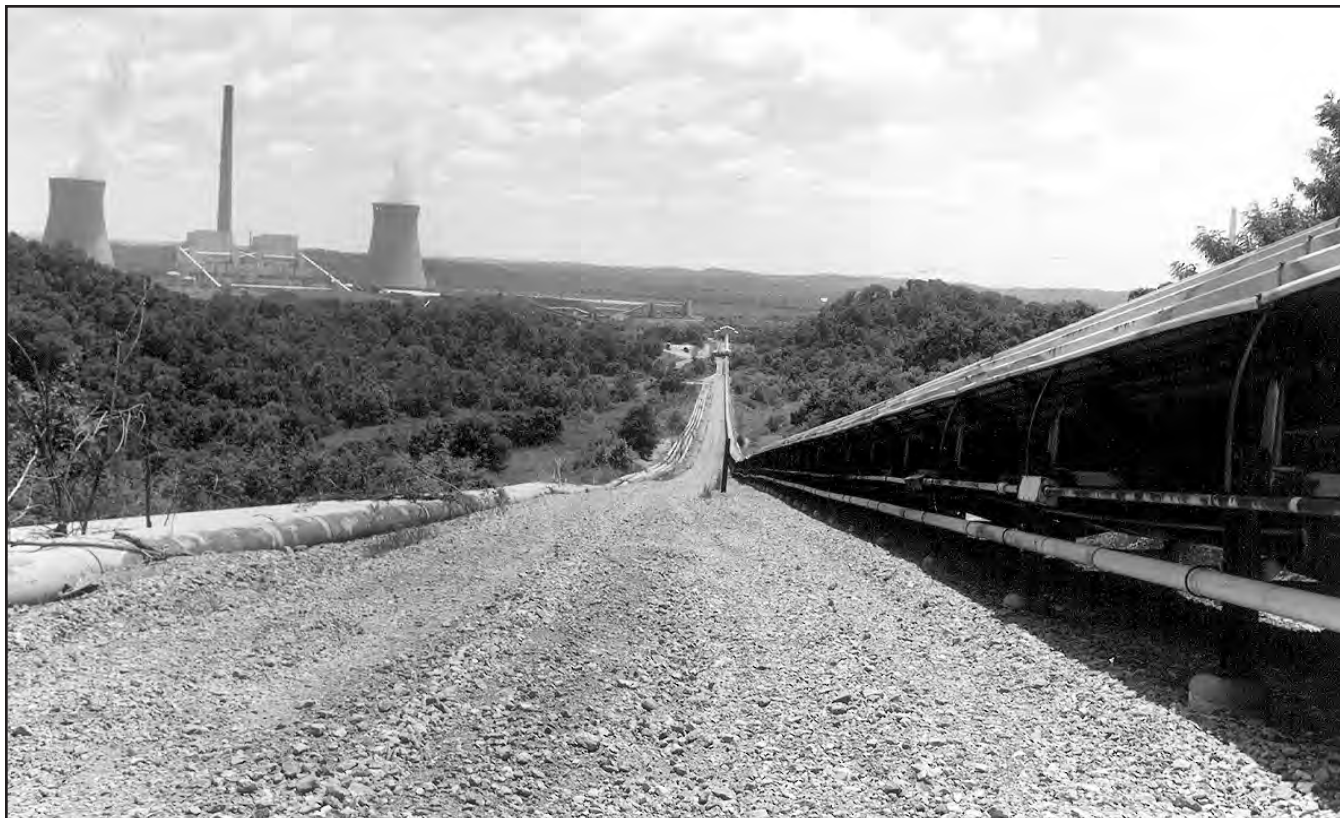
FIGURE 201.—Portion of a 10-mile-long overland conveyor that carries coal from the Southern Ohio Coal Company Meigs Division underground mine complex (Meigs No. 2 and No. 31 mines, Ms-293 and Ms-294) to the Gen. James M. Gavin generating station (background). The belt line of this conveyor runs at speeds up to 1,000 feet per minute. Date unknown. Photo courtesy of American Electric Power Service Corporation. (See also figs. 46, 216, 219.)
