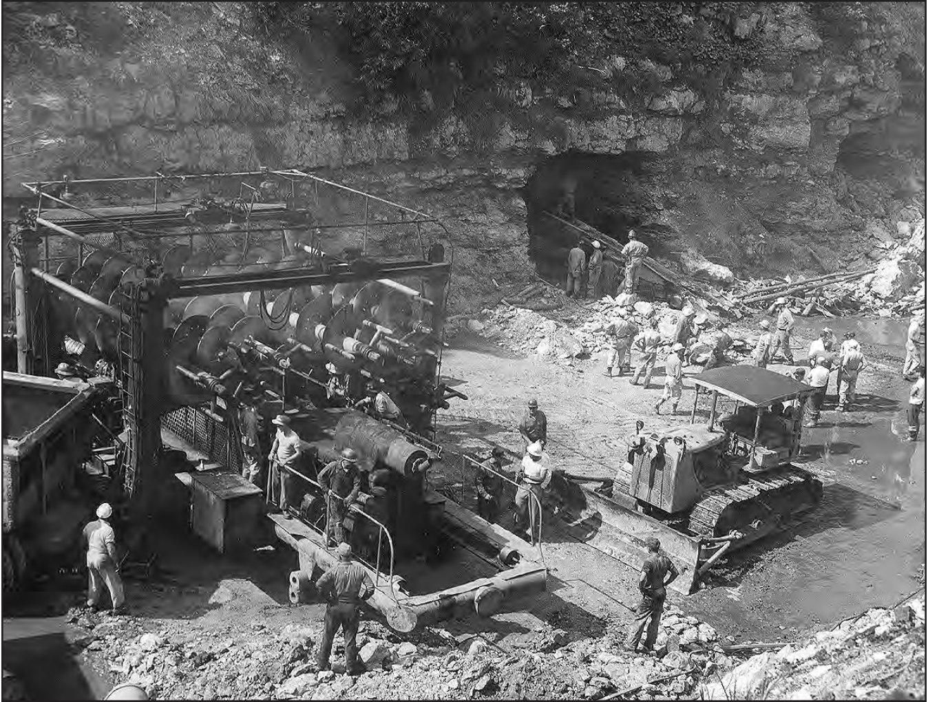
FIGURE 144.—Auger used to rescue trapped miners on June 26, 1957, at the Powhatan Mining Company Betsy No. 3 mine (Jfn-258) near Fernwood, Cross Creek Township, Jefferson County. Photo courtesy of Ohio Department of Industrial Relations, Division of Mines.
