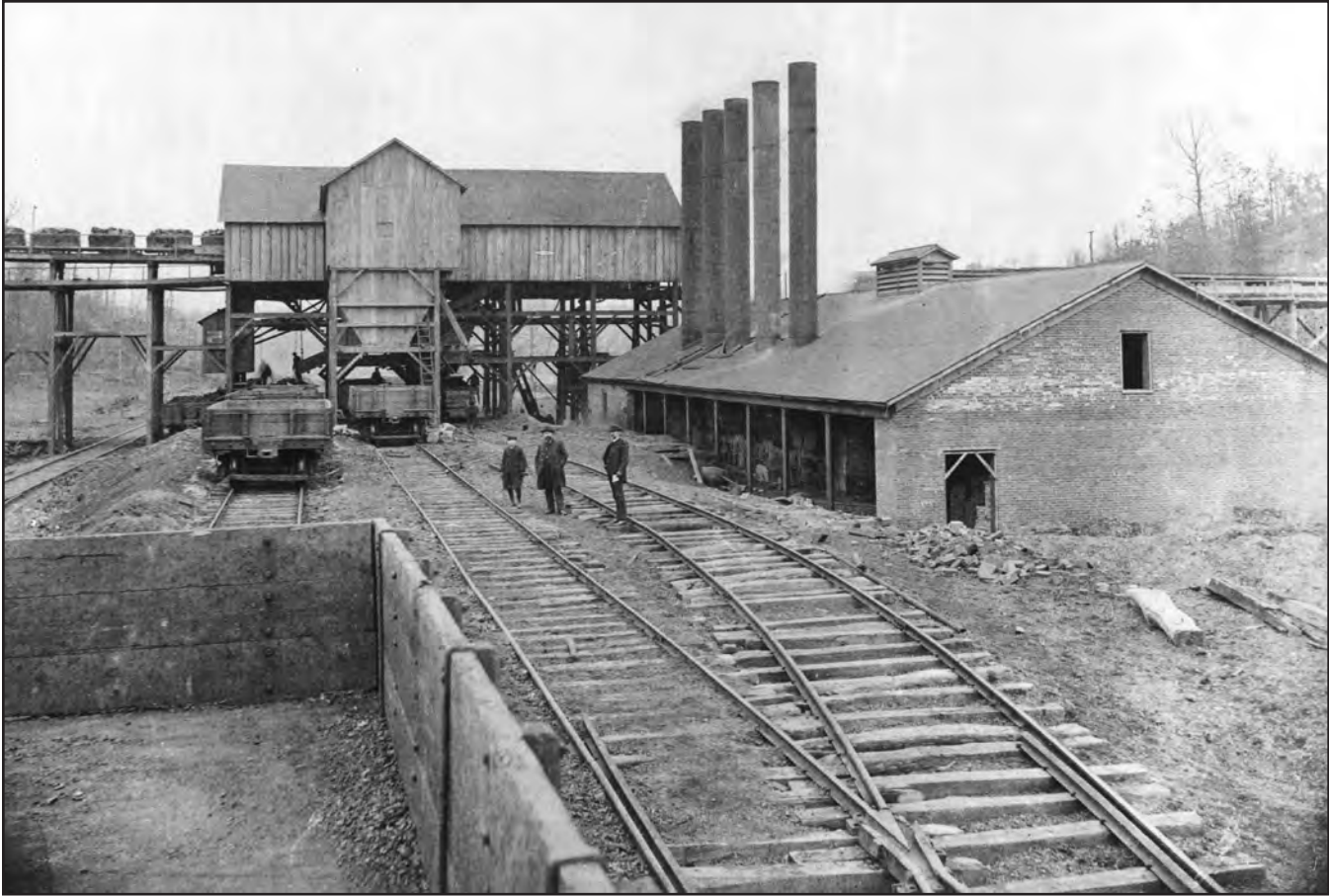
FIGURE 3.—Scene typical of eastern Ohio coal-mining operations during the 1890's. Wooden-side railroad cars are waiting to be loaded at a coal tipple. Note the loaded mine cars on the trestle (top left) en route to the tipple. Location unknown. Photo courtesy of Ohio Historical Society.
