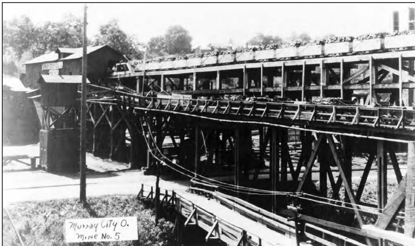
FIGURE 8.—Loaded mine cars en route to the coal tipple of Murray Coal Company mine No. 5 (As-168, As-175, and Hg-161) near Murray City in Ward Township, Hocking County, and Trimble Township, Athens County. This drift mine in the Middle Kittanning (No. 6) coal was operated by the Sunday Creek Coal Company until 1938, then under a variety of leases until it was abandoned in 1952. Date unknown. Photo courtesy of Ohio University, Vernon R. Alden Library, from the Mathaney collection.
