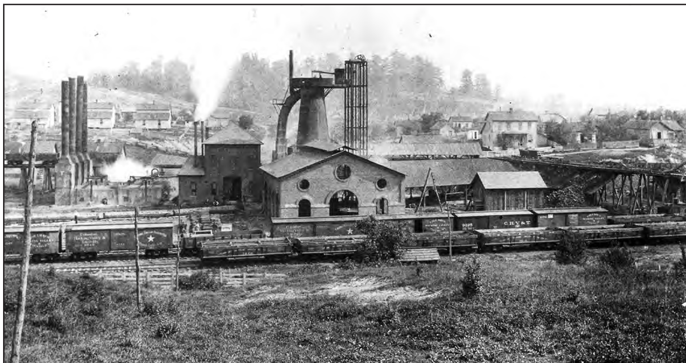
FIGURE 209.—Gore Furnace, at Gore, Hocking County. This coal-fired furnace, built in 1876, was one of the largest of the Hocking Valley iron furnaces. Circa 1887. Photo courtesy of Ohio Historical Society, from the W. E. Buchanon collection.
