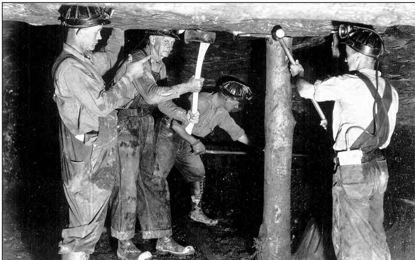
FIGURE 106.—Coal miners setting roof-support timbers in an underground mine near New Straitsville, Perry County. Circa 1936. Photo courtesy of Ohio Historical Society, from the WPA Ohio collection.
