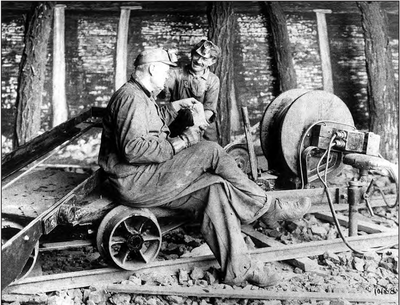
FIGURE 99.—Two miners on break in an eastern Ohio coal mine. Note the cloth miner's caps with carbide lamps, the numerous logs used as roof support, and the electrical cables draped across the mine-car rails. Circa early 1900's. Photo courtesy of Ohio Historical Society, from the Jeffrey Mining Equipment collection.
