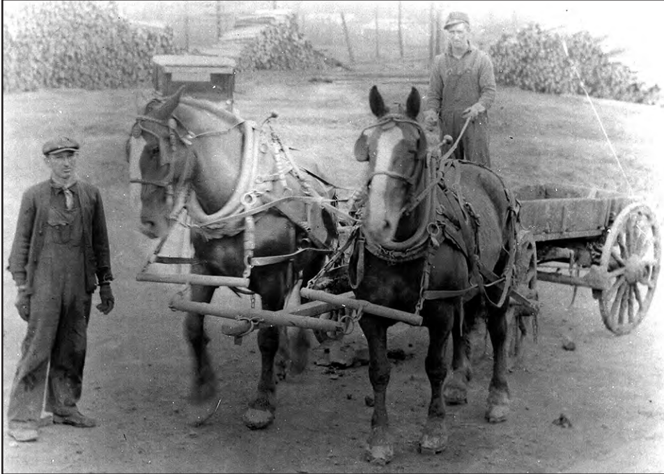
FIGURE 111.—Stacks of roof-support timbers to be used in the mine form the backdrop for two outside workers at the Crow Hollow (Bradley) mine (Jfn-179). This mine is about 2 miles north of Dillonvale (at Bradley), in Smithfield Township, Jefferson County. Ten drift openings were driven into the Pittsburgh (No. 8) coal by the United States Coal Company in 1902. For a brief period following the opening of the mine, these drift openings were grouped into districts. Openings Nos. 1 through 4 were known as Bradley District No. 1, openings Nos. 5 and 6 were Bradley District No. 2, openings Nos. 7 and 8 were Bradley District No. 3, and openings Nos. 9 and 10 were Bradley District No. 4. In 1912, the name Bradley was dropped and Crow Hollow was adopted. The Crow Hollow mine was operated by the United States Coal Company from 1902 to 1932 and by the Jefferson Coal Company from 1932 to 1944, when it was abandoned. In 1907, the mine had a daily capacity of 2,500 tons. Circa 1910. Photo courtesy of Dale Davis, from the Leonard Corona collection.
