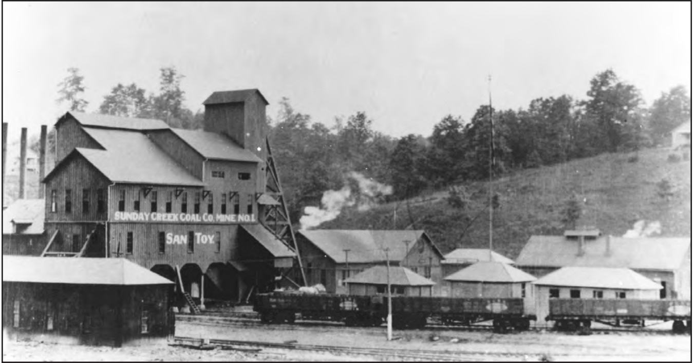
FIGURE 6.—Hoisting-shaft headframe, tibble, and company buildings of the Sunday Creek Coal Company San Toy mine No. 1 (Ohio Division of Mines abandoned-mine-map file number Py-63; see footnote 1 on p. 29 for explanation). This underground mine, located in San Toy, Monroe Township, Perry County, was opened by the New England Coal Company in 1902 to mine the Middle Kittanning (No. 6) coal. In 1915, Sunday Creek Coal Company took over the operation. This mine operated until 1927, when it was abandoned. The hoisting shaft was 195 feet deep and 26 feet by 13 feet wide. Date unknown. Photo courtesy of Ohio University, Vernon R. Alden Library, from the Mathaney collection.
