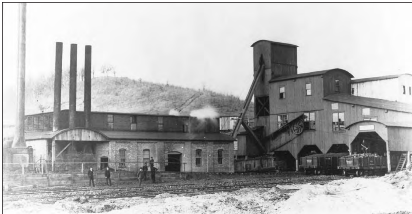
FIGURE 9.—Hoisting-shaft headframe, tipple, and powerhouse of New York Coal Company mine No. 25 (As-157) at Chauncey in Dover Township, Athens County. This mine, formerly known as mine No. 275 and operated by the Sunday Creek Coal Company, had a 125-foot-deep shaft, mined Middle Kittanning (No. 6) coal, and was abandoned in 1952. Date unknown. Photo courtesy of Ohio University, Vernon R. Alden Library, from the Mathaney collection.
