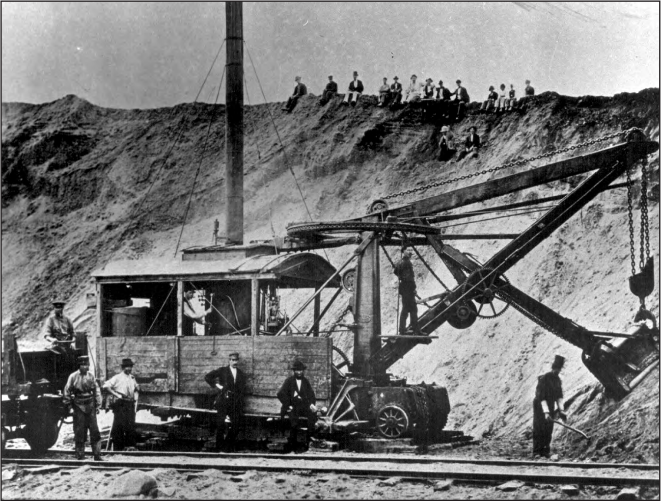
FIGURE 18.—A coal-fired steam shovel that operated on rails. Circa 1890's, location unknown. Photo courtesy of Ohio Department of Natural Resources, Division of Reclamation, from the Dale Davis collection.
