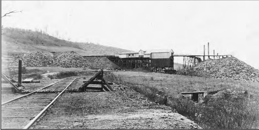
FIGURE 54.—Railroad-car-loading tippel of the Sterling mine (Cl-59), about 1 mile west of Salineville, in Fox Township, Carroll County. The Sterling mine had drift openings into the Mahoning (No. 7A) coal, which averaged 3 feet in thickness. This mine was opened by the Sterling Mining Company in 1901 and was abandoned, under the ownership of the Hirst Coal Company, in 1961. Note the large piles of “gob” or waste material, a by-product of the coal mining or coal cleaning process. Circa 1910. Ohio Division of Geological Survey file photo by D. Dale Condit.
