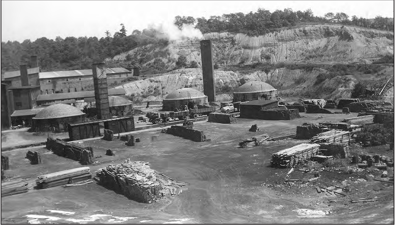
FIGURE 210.—Plant and shale pit of the General Clay Products Company, 1/2 mile northeast of Baltic, in Clark Township, Holmes County. The Lower Kittanning (No. 5) and Middle Kittanning (No. 6) coals were used until the mid-1960's to heat kilns in the manufacture of tile. Circa 1949. Ohio Division of Geological Survey file photo by George W. White.
