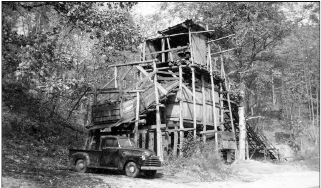
FIGURE 55.—Small truck-loading tippel for a drift mine in the Clarion (No. 4A) coal along Ohio Route 278, in Brown Township, Vinton County. Tippels such as this were common throughout eastern Ohio to supply local domestic fuel needs. Circa 1953. Ohio Division of Geological Survey file photo.
