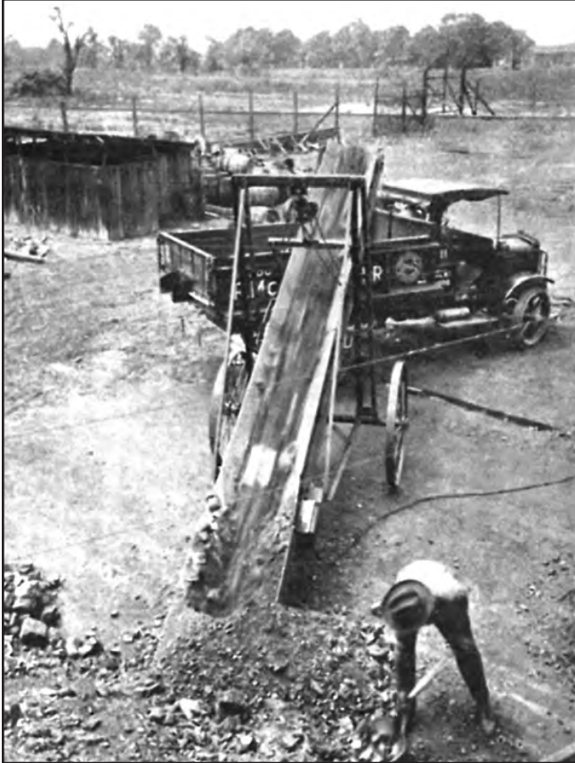
FIGURE 199.—One man, shoveling coal by hand onto an electric-powered conveyor, could load a 2-ton delivery truck in 5 minutes. Without the conveyor, four good men took 30 minutes to load the same truck. Photo from The Coal Trade Bulletin (1923, v. 49, no. 5, p. 215).
