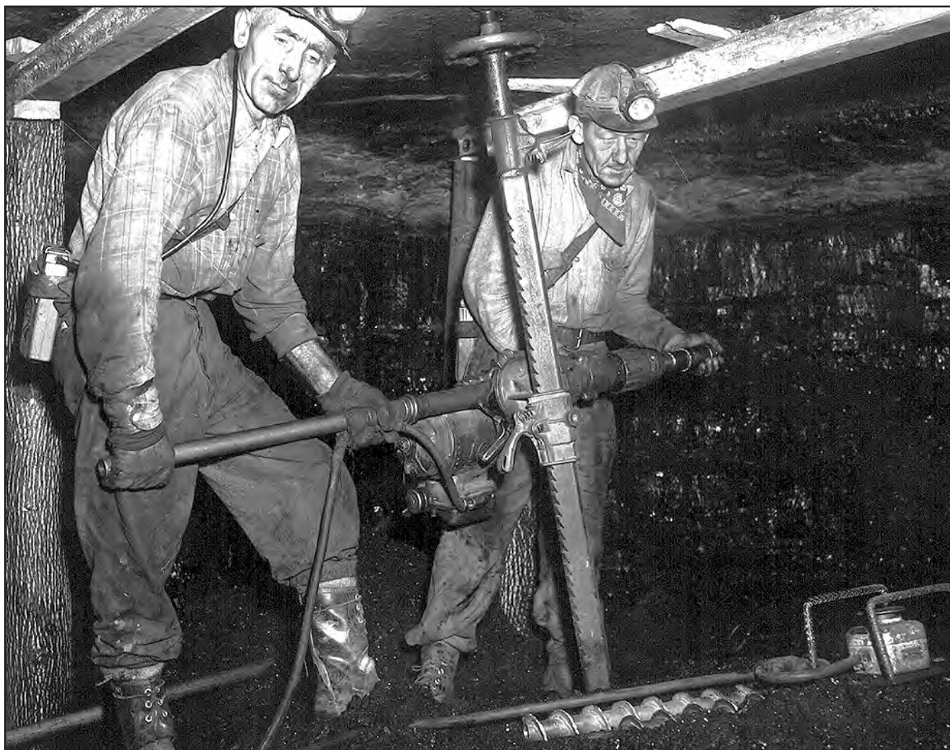
FIGURE 76.—Coal miners operating a compressed-air-driven drill in an eastern Ohio coal mine. Miners usually worked in pairs and never alone for the purpose of safety. Date unknown. Photo courtesy of Ohio Department of Industrial Relations, Division of Mines.
