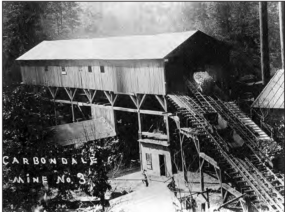
FIGURE 183.—Railroad-car-loading tipple of the Carbondale Coal Company mine No. 3 (As-256). This mine, located northwest of Carbondale, in York Township, Athens County, was abandoned in 1952. Note the loaded and empty coal cars being moved by wire-line hoists. Date unknown. Photo courtesy of Mark Wharton.
