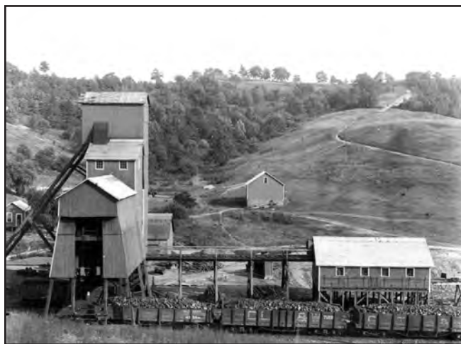
FIGURE 57.—Loading a string of railroad cars at the railroad-car-loading tippel and hoisting-shaft headframe of the Midvale No. 4 mine (Ts-337), formerly Beaver Dam No. 2 mine and Scott B No. 1 mine. This mine, located about 1 1/2 miles east of Midvale, in Union Township, Tuscarawas County, opened in 1904 and used an 85-foot-deep shaft to mine a 4-foot-thick seam of Middle Kittanning (No. 6) coal. It was operated at various times by the Goshen Coal Company, the Beaver Dam Coal Company, the Scott Coal Company, and John Marchesi and was abandoned in 1943 under the ownership of the Midvale Coal Company, Inc. Date unknown. Photo courtesy of Tuscarawas County Historical Society.
