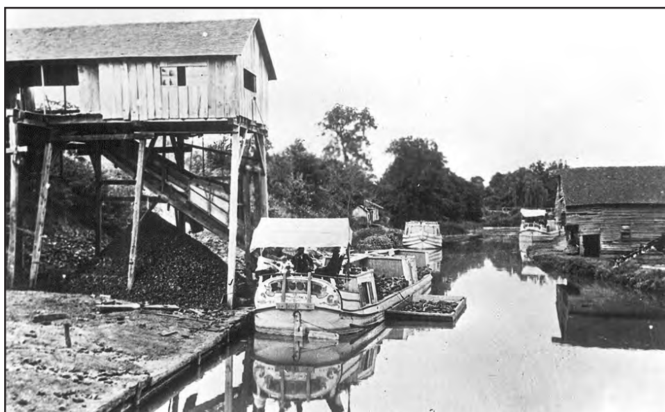
FIGURE 170.—The canal boat E. Moore taking on a load of coal from the tippie of the Trenton mine (Ts-74), on the west bank of the Ohio and Erie Canal at Tuscarawas (formerly Trenton), in Warwick Township, Tuscarawas County. The Trenton mine, a drift mine in the Middle Kittanning (No. 6) coal, was operated by Henry C. Minnich and was abandoned in 1902. Coal from the Trenton mine was taken to northern markets. Coal mined in the vicinity of Trenton, amounting to 48 boatloads, was first shipped to Cleveland via the Ohio and Erie Canal in 1836 (Heydinger, 1974, p. 36). Circa 1889. Photo courtesy of The University of Akron Archives, Canal Society of Ohio collection.
