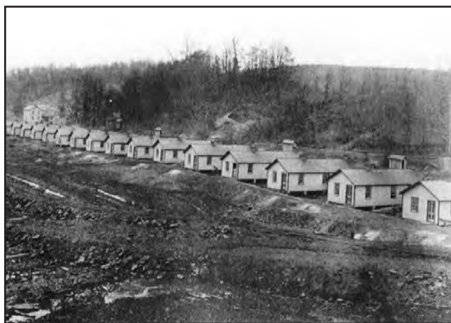
FIGURE 65.—Even when newly constructed, multi-family company housing in this Hocking Valley coal town was stark and primitive (Boryczka and Cary, 1982, p. 65). Circa mid-1890's. Photo courtesy of Ohio Historical Society, from the Frank W. Jennings collection, collection number P6.
