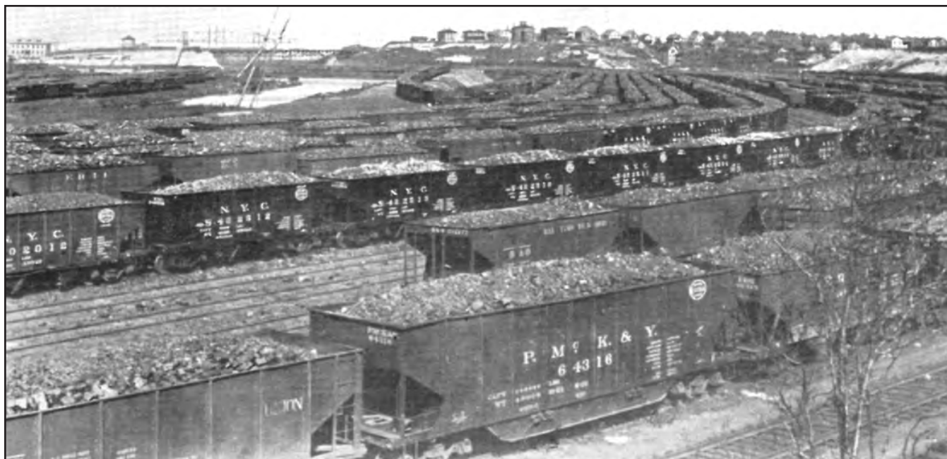
FIGURE 180.—A typical scene at Ashtabula Harbor during the 1920's—coal from approximately 3,000 coal-filled railroad cars, including coal cars of the New York Central Railroad (NYC) and the Pittsburgh, McKeesport & Youghiogheny Railroad (P McK & Y), waiting for transport by lake freighter. Photo from The Coal Trade Bulletin (1923, v. 48, no. 3, p. 111).
