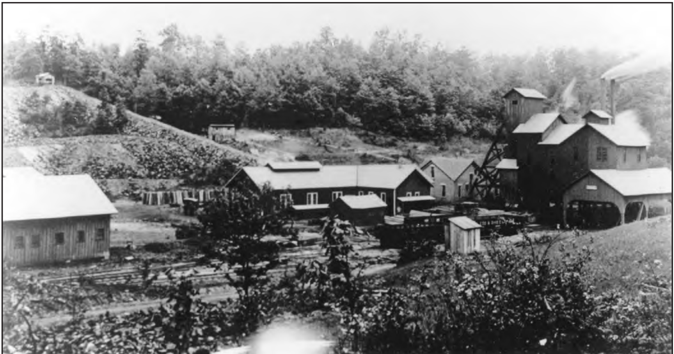
FIGURE 7.—Hoisting-shaft headframe, tibble, and company buildings of Gem Coal Company mine No. 255 (As-191 and As-132) on Baily Run about 2 miles southwest of Jacksonville in Dover Township, Athens County. Mine No. 255 had a 135-foot-deep shaft to the Middle Kittanning (No. 6) coal. This mine was opened in 1903 by the Continental Coal Company and was operated by the Sunday Creek Coal Company from about 1907 to 1918, the Drydock Coal Company from 1918 to 1955, and the Gem Coal Company from 1955 until its abandonment in 1963. This mine used horses until about 1906, when electric locomotives were installed for coal haulage. A new tibble, replacing the one shown here, was built in 1945. Date unknown. Photo courtesy of Ohio University, Vernon R. Alden Library, from the Mathaney collection.
