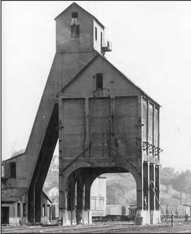
FIGURE 185.—Coal tippie at the railroad yards in Dennison, Tuscarawas County. Circa 1955. Photo courtesy of Dennison Railroad Museum, Don Case collection.
