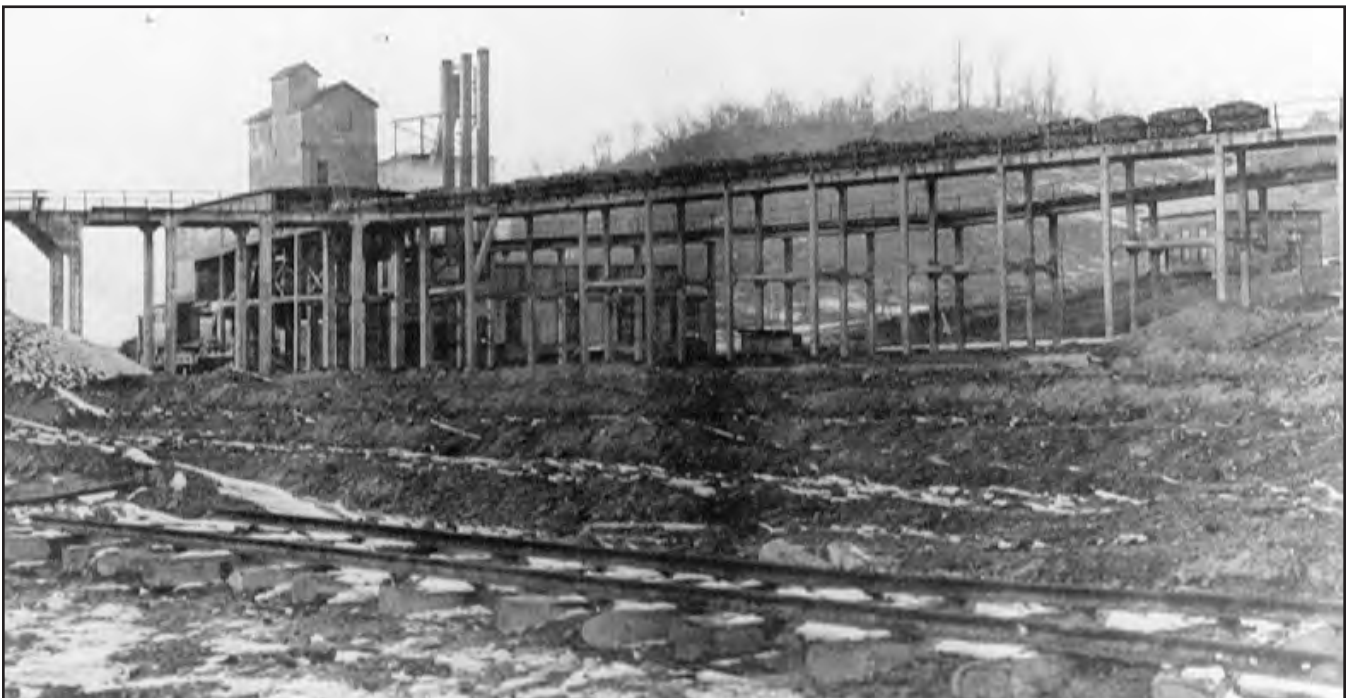
FIGURE 62.—Unique concrete coal tippie and trestle of the Black Diamond No. 2 mine (As-141), operated by the Black Diamond Coal Company near Lathrop, in Bern Township, Athens County. Photo from State Inspector of Mines Report (1912, p. 289).
