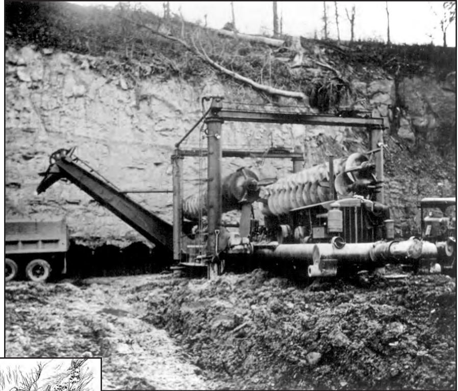
FIGURE 48.—Coal-auger mine. Circa 1956. Location unknown. Photo courtesy of Ohio Department of Natural Resources, Division of Reclamation.
