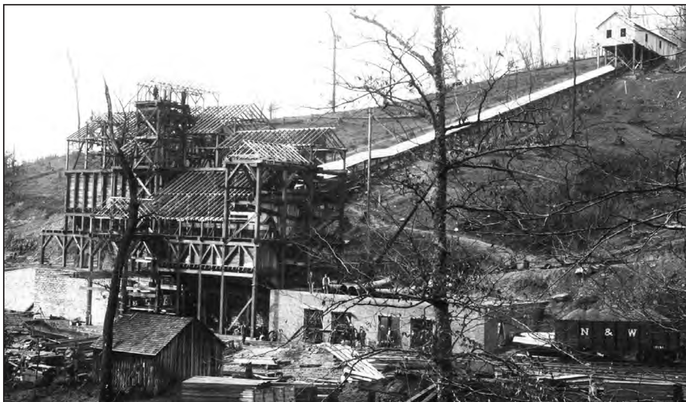
FIGURE 53.—Coal tipple under construction. Coal was moved downhill from the mine mouth to the tipple, where it was separated by size (see fig. 51) for shipment by rail. Circa 1890's. Location unknown. Photo courtesy of Ohio Historical Society, Jeffrey Mining Equipment collection.
