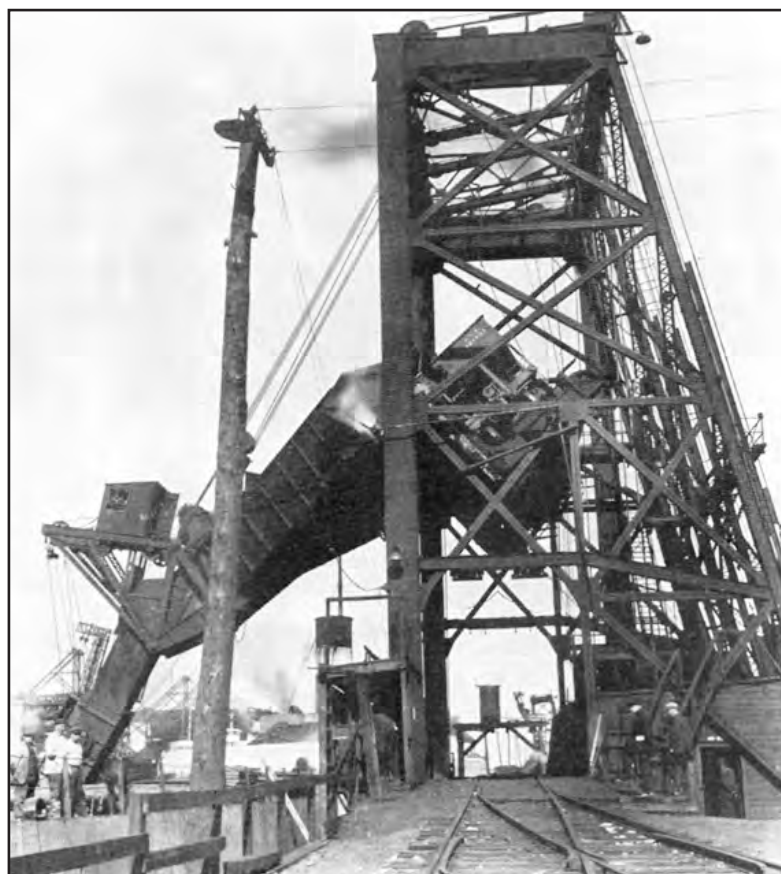
FIGURE 181.—Coal elevator at Ashtabula Harbor dumping coal into lake freighters a carload at a time. The elevator raises the railroad car to the level of the hopper, where the railroad car is tipped over, dumping the coal into the hopper, which feeds the freighter. The entire process of raising, dumping, and lowering a railroad car takes only a minute. Photo from The Coal Trade Bulletin (1923, v. 48, no. 3, p. 110).
