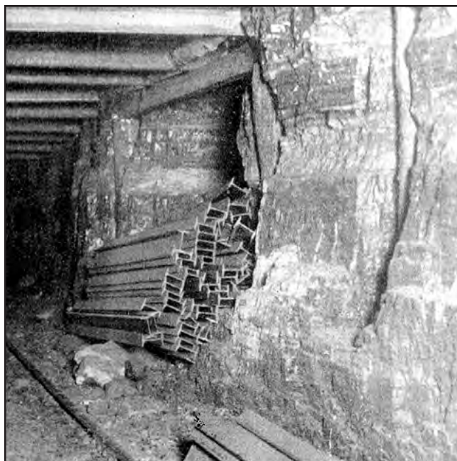
FIGURE 113.—Steel beams were used as roof support instead of wood timbers in the Youghiogheny & Ohio (Y & O) Coal Company Boggs mine (Bt-252), located approximately 1 mile east of St. Clairsville, in Richland Township, Belmont County. The Boggs mine, a drift mine, was opened in 1887 and was operated until 1906 by E. N. Boggs. Y & O operated the Boggs mine from 1906 until it was abandoned in 1927. Pittsburgh (No. 8) coal, 5½ feet thick, was produced from this mine. Photo from The Coal Trade Bulletin (1909, v. 21, no. 5, p. 21).
