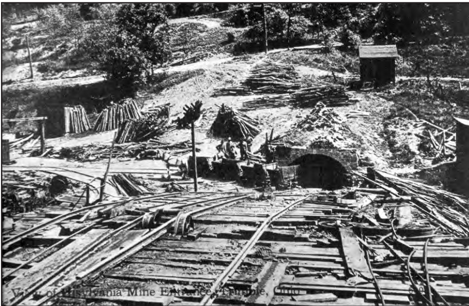
FIGURE 41.—Opening and coal-haulage tracks to the Hisylvania Coal Company mine No. 22 (As-22) in Trimble, Trimble Township, Athens County. This slope mine was abandoned in 1925. Circa 1901.
