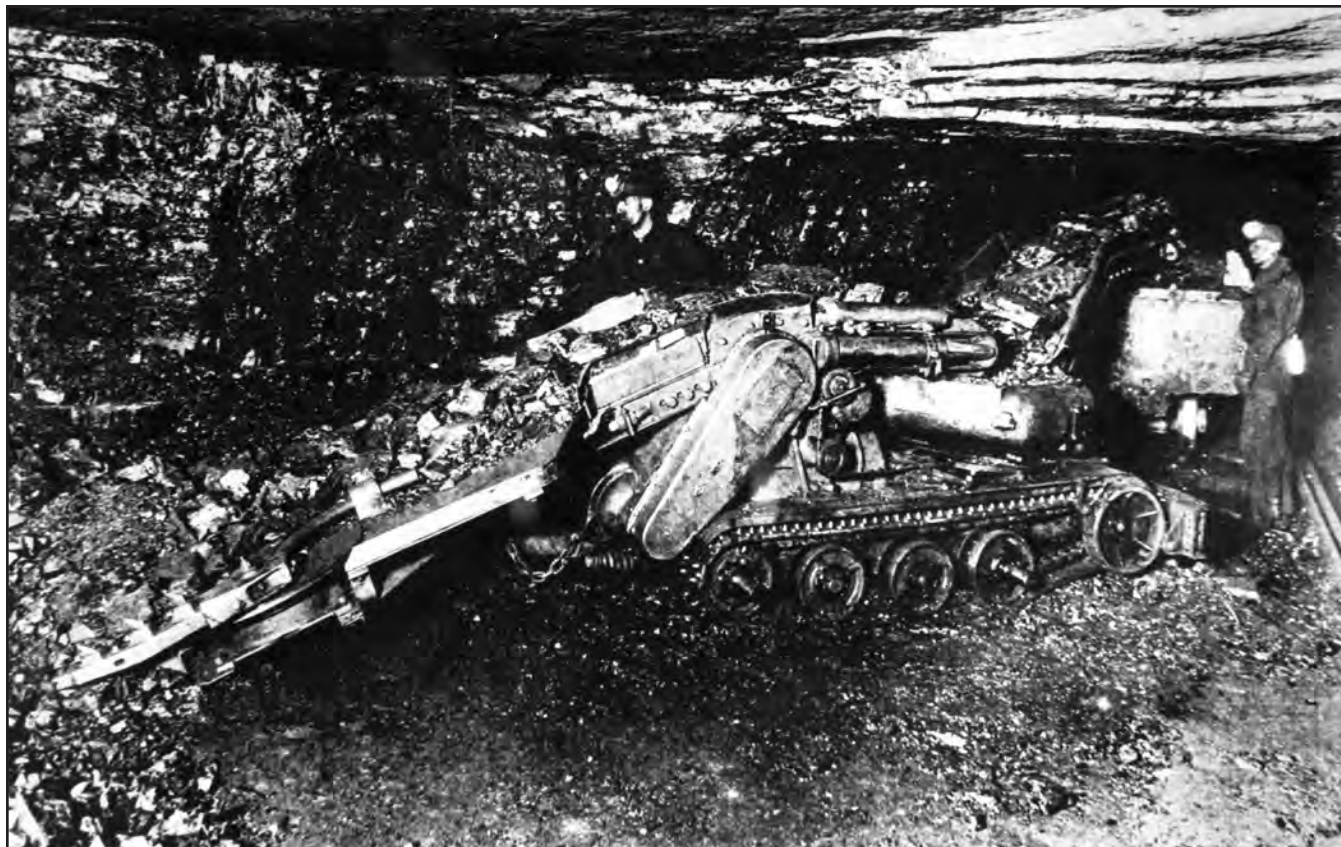
FIGURE 4.—Coal being loaded into a mine car by conveyor of a gathering/loading machine. Evidence of a roof-support system is lacking in the portion of the mine shown in this photograph. Ohio's current mine law specifies roof-support procedures, including the use of roof bolts and timbers. These procedures also limit the mining activity beyond an unsupported roof. Date and location unknown. Photo courtesy of U.S. Bureau of Mines.
