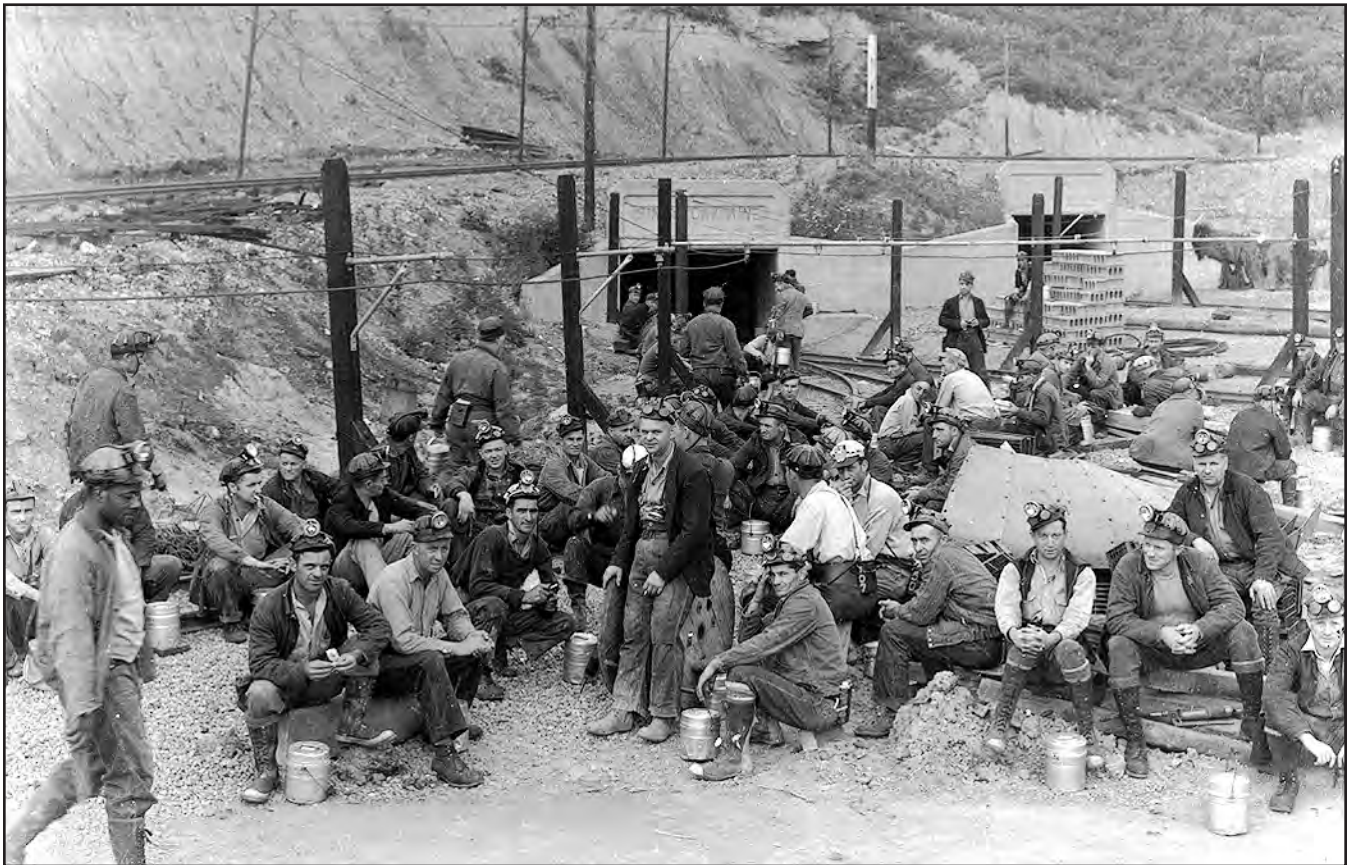
FIGURE 74.—Miners waiting to start the afternoon shift at the Hanna Coal Company Piney Fork No. 1 mine (Jfn-243) in 1943. During World War II this mine employed over 1,000 men and was one of the country's leading coal producers. This drift mine near Smithfield, Jefferson County, was abandoned in 1959. Note the dinner buckets at many of the miners' feet. Photo courtesy of Ohio Department of Natural Resources, Division of Reclamation, from the Dale Davis collection. (For other photos of this mine see figs. 36, 101, 116, 121, 159.)
