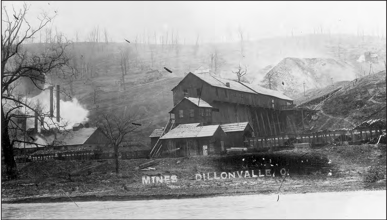
FIGURE 179.—Tipple at Dillonvale in Mount Pleasant and Smithfield Townships, Jefferson County, supplying coal to the Wheeling & Lake Erie Railroad. Circa 1910. Photo courtesy of Ohio Historical Society.
