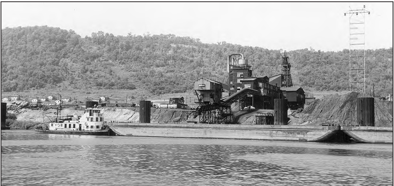
FIGURE 166.—Coal being loaded into barges at the barge-loading dock at the North American Coal Corporation Powhatan No. 1 mine (Bt-270). The Powhatan No. 1 mine, a slope mine in York Township, Belmont County, produced Pittsburgh (No. 8) coal from about 1923 to 1981, when it was abandoned. Circa 1953. Photo courtesy of North American Coal Corporation.
