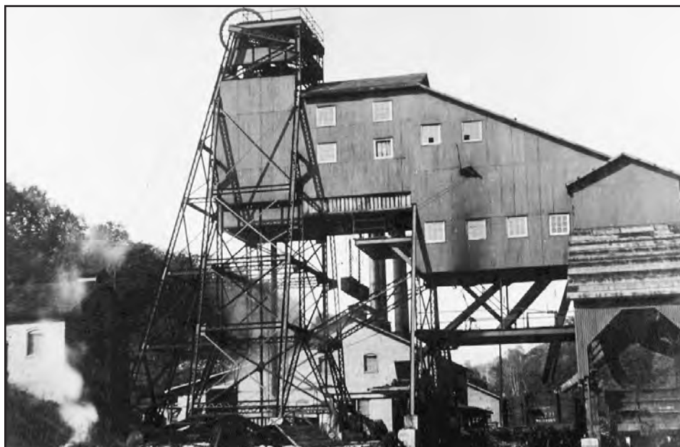
FIGURE 60.—Top photo, men and hoisting equipment used to construct the 450-foot-deep shaft of the Canaanville mine No. 1 (As-134), located at Canaanville, in Canaan Township, Athens County. Bottom photo, hoisting-shaft headframe and tippel of the Canaanville mine No. 1 as it appeared in 1909. This mine, built in 1905, was operated by the Canaan Coal Company until it was abandoned in 1925. Top photo courtesy of Ohio University, Vernon R. Alden Library, from the Mathaney collection; bottom photo courtesy of Mark Wharton.
