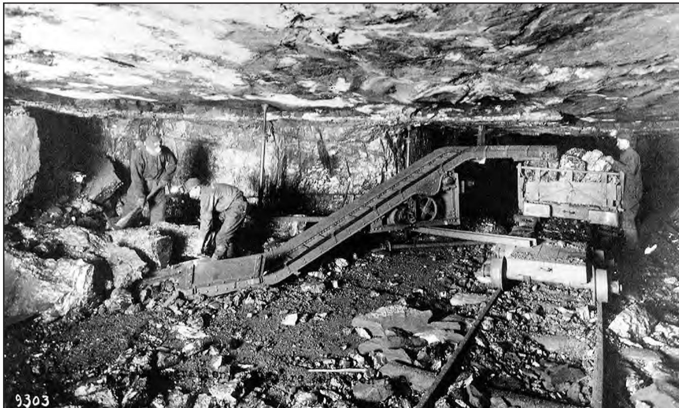
FIGURE 84.—A pair of miners loading coal by hand in an eastern Ohio coal mine. Coal was lifted or shoveled onto a chain conveyor, which loaded a mine car. Until the mid-1930's and the development of automatic coal-loading machines, coal was loaded into mine cars by hand. Circa early 1900's. Location unknown. Photo courtesy of Ohio Historical Society, from the Jeffrey Mining Equipment collection.
