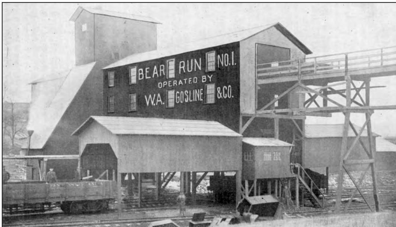
FIGURE 52.—Tipple of the Bear Run No. 1 mine (Py-214), which is about 3 miles east of New Lexington, in Pike Township, Perry County. This mine, operated by W. A. Gosline & Son, was served by the Cleveland & Marietta branch of the Pennsylvania Railroad. The Bear Run No. 1 mine was abandoned in 1924. Photo from State Inspector of Mines Report (1905, p. 32).
