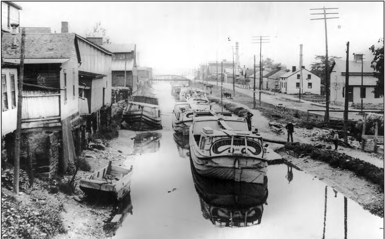
FIGURE 171.—Canal boats on the Ohio and Erie Canal south of West Tremont Avenue in Massillon, circa 1890's. Photo courtesy of The Massillon Museum.
