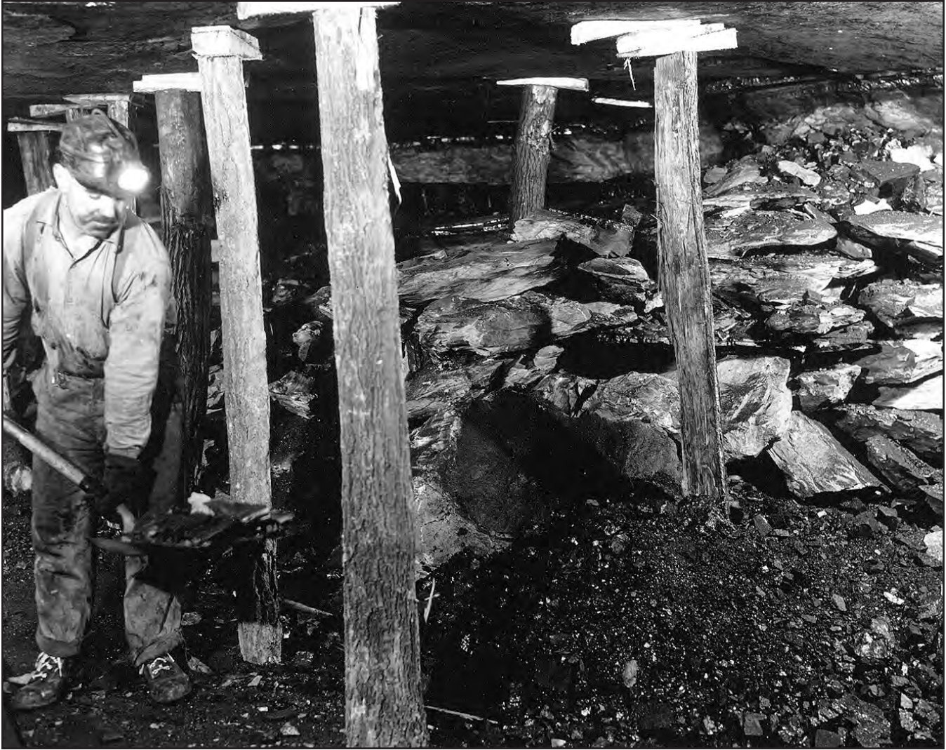
FIGURE 107.—Coal miner shoveling gob (waste material). Note the roof-support system of timbers and wooden wedges. Date and location unknown. Photo courtesy of Ohio Department of Industrial Relations, Division of Mines.
