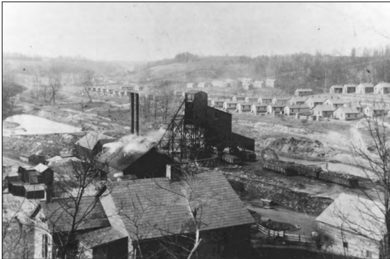
FIGURE 63.—Hoisting-shaft headframe and railroad-car-loading tiple of the Sunday Creek Coal Company San Toy mine No. 2 (Py-64) surrounded by company-owned homes and buildings. Date unknown. Photo courtesy of Forrest Walton. (For another photo of this mine see fig. 59.)
