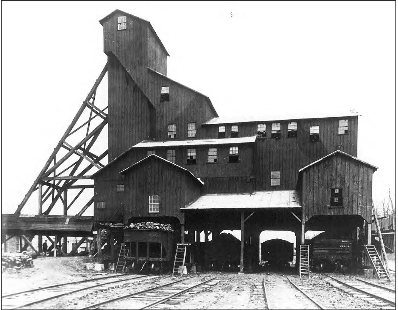
FIGURE 135.—Hoisting-shaft headframe and tippel of the Sunday Creek Coal Company mine No. 6 (As-142). This mine is about 1 mile east of Millfield, in Dover Township, Athens County, and was the site of Ohio's worst coal-mine disaster in 1930. Circa 1940. Photo courtesy of Walter R. Ervin.
