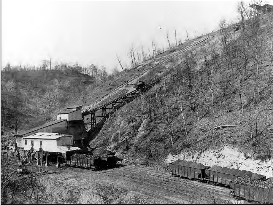
FIGURE 182.—Crusher and railroad-car-loading coal tipple to the Beech Flats mine (Jfn-56), located near Rush Run, in Wells Township, Jefferson County. This surface mine, operated by the Beech Flats Coal Company, was abandoned in 1924. Date unknown. Photo courtesy of Ohio Historical Society.
