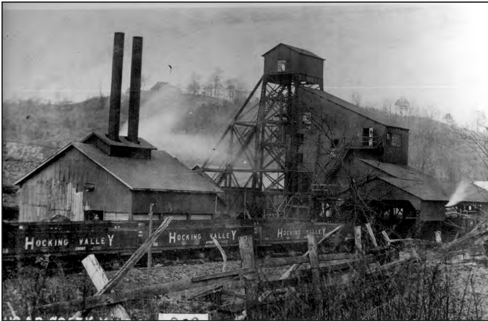
FIGURE 30.—Construction (top photo) of the hoisting-shaft headframe and tippel of the Continental Coal Company mine No. 209 (As-111) was completed in early 1905. This structure was built near Sugar Creek, in Dover Township, Athens County. Mine No. 209 provided Middle Kittanning (No. 6) coal to the Hocking Valley Railroad (bottom photo; date unknown) for 19 years until it was abandoned in 1923. Photos courtesy of Mark Wharton.
