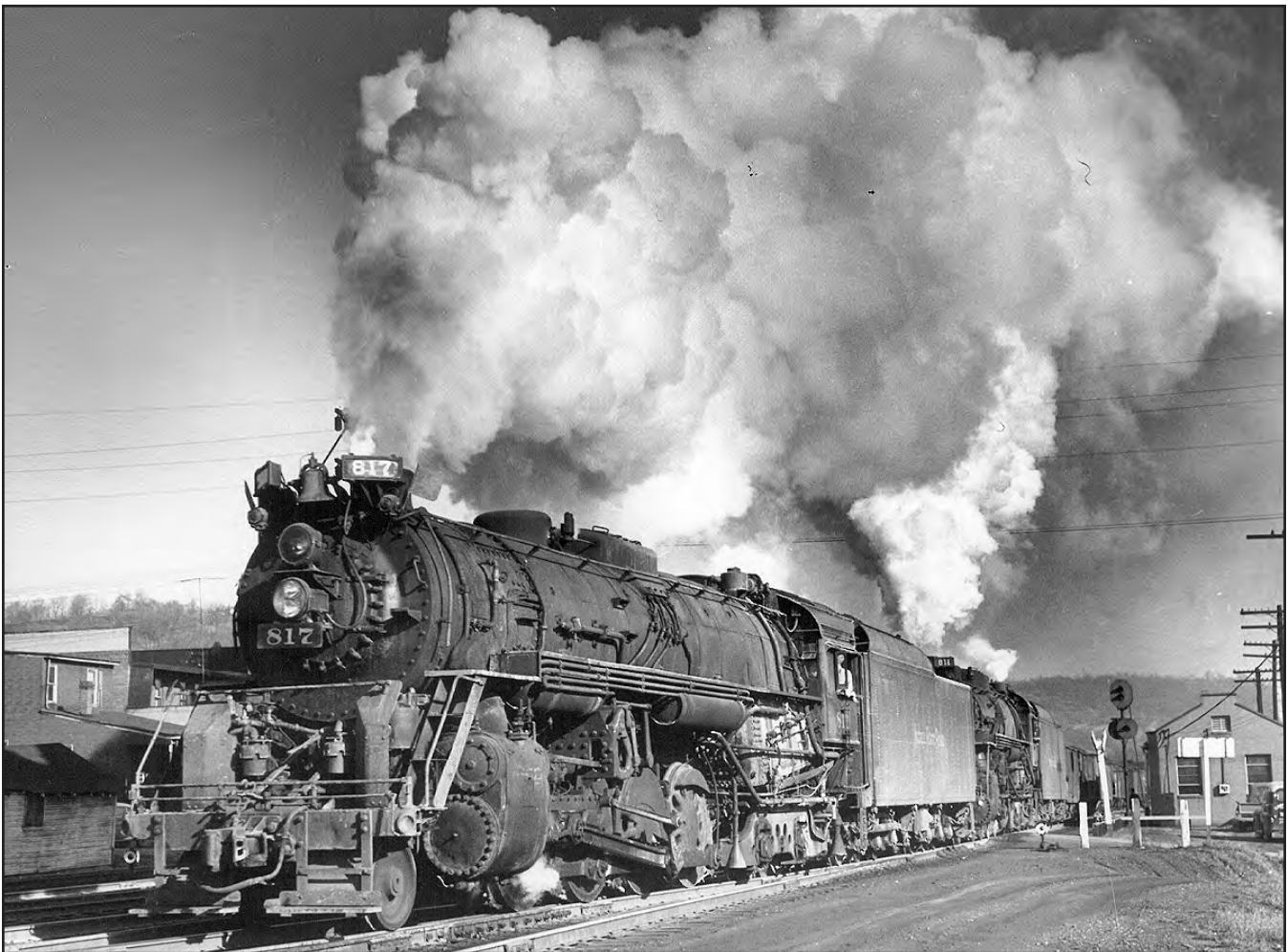
FIGURE 190.—On a brisk December afternoon in 1956, a pair of Nickel Plate Railroad 2-8-4's, #817 and #811 (nee W & LE #6417 and #6411), pulled 6,500 tons of Pittsburgh (No. 8) coal from the Pine Valley yards at Dillonvale (Jefferson County) on the tough grade out of the Ohio River valley bound for Brewster (Stark County). Photo and information courtesy of J. J. Young, Jr.
