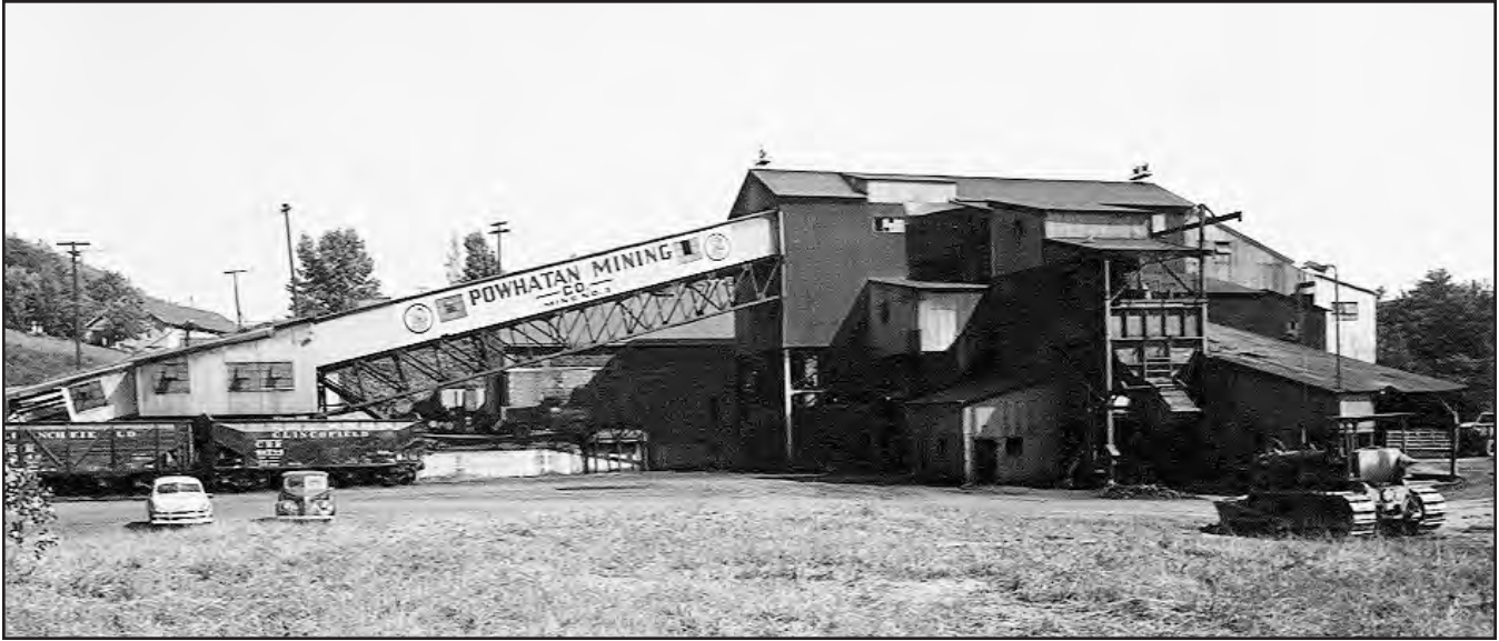
FIGURE 58.—Railroad-car-loading tippel of the Powhatan No. 3 mine (Bt-282), operated by the Powhatan Mining Company (formerly by North American Coal Corporation). This slope mine in Mead Township, Belmont County, mined the Pittsburgh (No. 8) coal from 1911 to 1986, when it was abandoned. Circa 1950. Photo courtesy of North American Coal Corporation.
