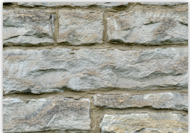
Weathered "Homewood" sandstone of the Stone Academy in West Zanesville, Muskingum County. The "Homewood" is very similar to the "Clarion" sandstone originally used for the second Ohio Statehouse in Zanesville.
