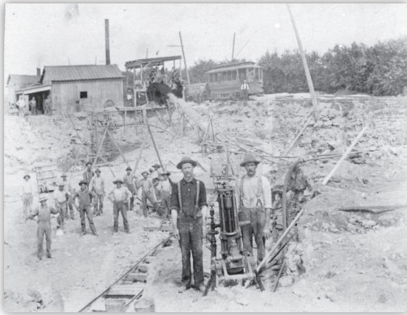
Workers in a quarry near Dublin Pike and Grandview Avenue, circa 1900. Photo courtesy of Grandview Heights/Marble Cliff Historical Society Archives.
