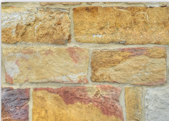
Berea Sandstone of the Adena Mansion in Chillicothe, Ross County. The Berea Sandstone was used to construct Ohio's first statehouse, also in Chillicothe.
