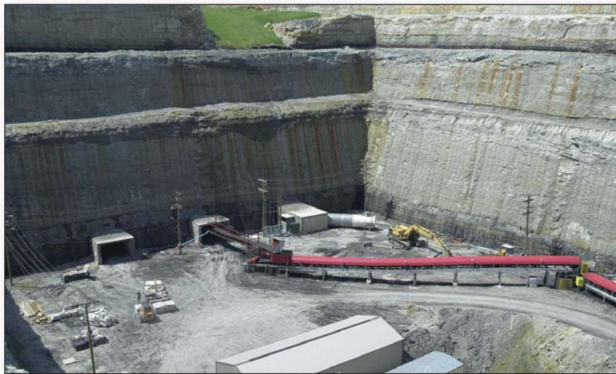
Two drift openings in the Middle Kittanning (known commercially as the No. 6 coal) operated by the Buckingham Coal Company at Glouster, Athens County, 2001. Photo by Mike Williams.
