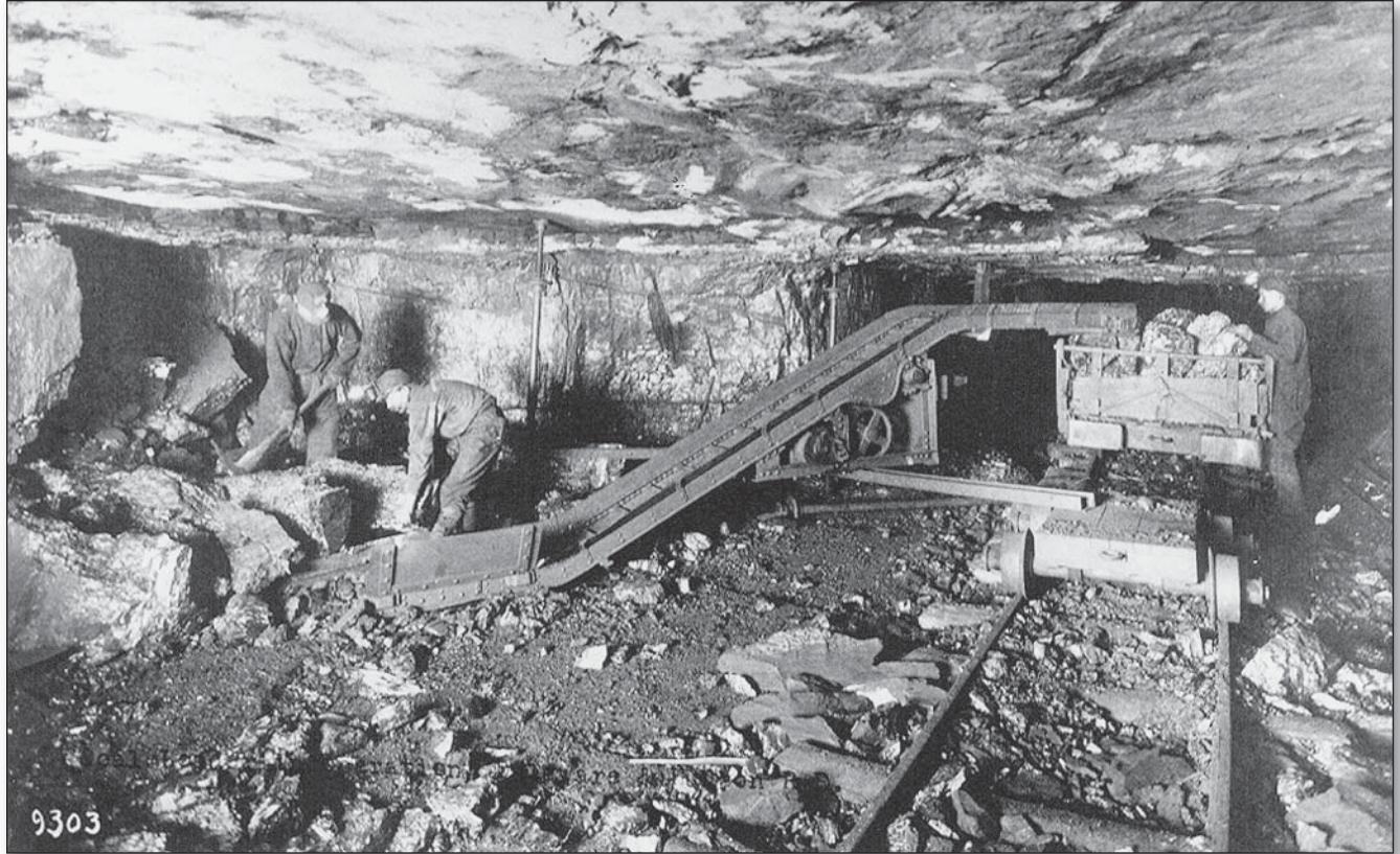
A pair of miners loading coal by hand in an underground coal mine in eastern Ohio, circa early 1900s. Coal was lifted or shoveled onto a chain conveyor, which loaded a mine car. Until the mid-1930s and the development of automatic coal-loading machines, coal was loaded into mine cars by hand. From Crowell, 1995, p. 63; photo courtesy of the Ohio Historical Society, from the Jeffery Mining Equipment collection.
