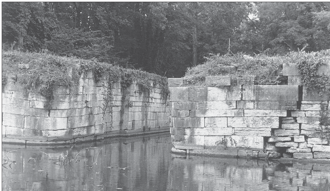
FIGURE 64.—Lock 8, Piqua Historical Area. Note greater deterioration of stone at water level and the leaning of the locks inward. Photo taken from the Genl. Harrison at a turn-around of the canal boat ride. August 1994 photo.
