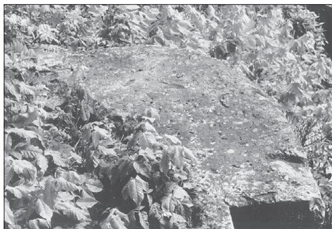
FIGURE 45.—Coping of West Portsmouth lock, made of sandstone from the Buena Vista Member of the Cuyahoga Formation. Lock is west of Ohio Rtes. 73/104 and north of turn-off to Ohio Rte. 239. Note rounded edge of lock and poison ivy. June 1995 photo.
