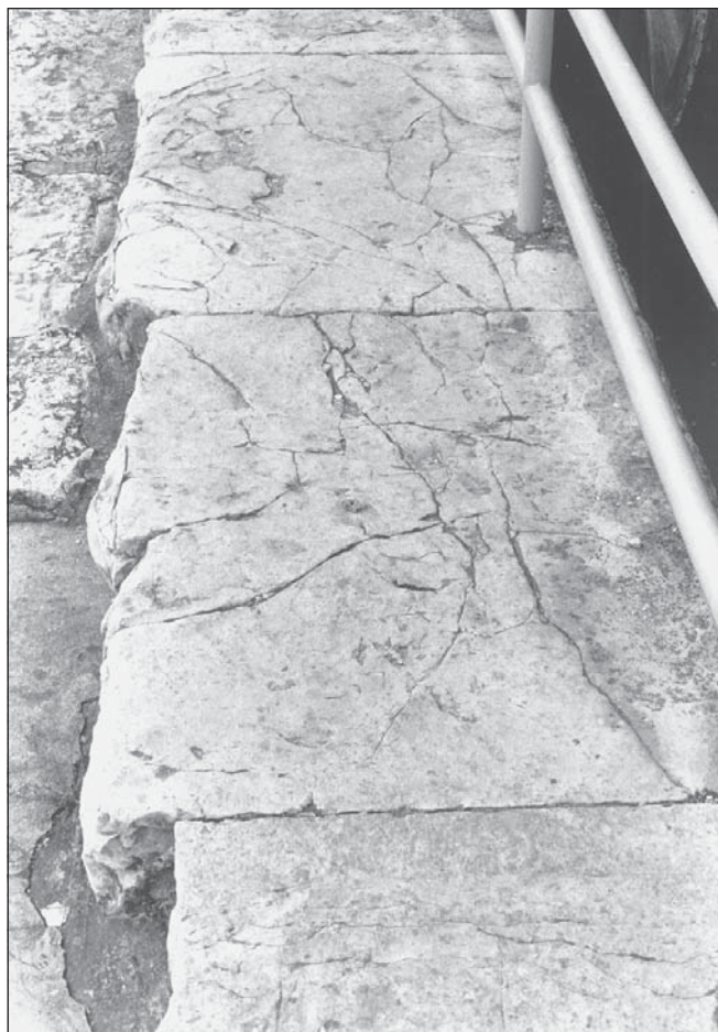
FIGURE 77.—Cracking in limestone used for coping of middle of south wall of Lock 25 at Metamora, Indiana. Pattern of cracks is typical of many limestones. August 1995 photo.
