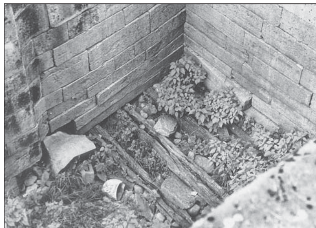
FIGURE 61.—Decaying wood at base of Lock 3, Lockington. Note slipping blocks of stone. August 1994 photo.
