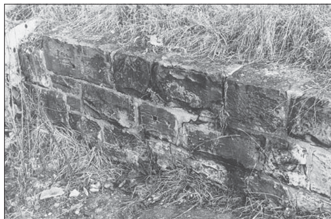
FIGURE 23.—Spillway, constructed of conglomeratic sandstone, probably the Sharon conglomerate, adjacent to Lock 14, Cascade Mills Lock, part of Cascade Valley Metropark. December 1997 photo.
