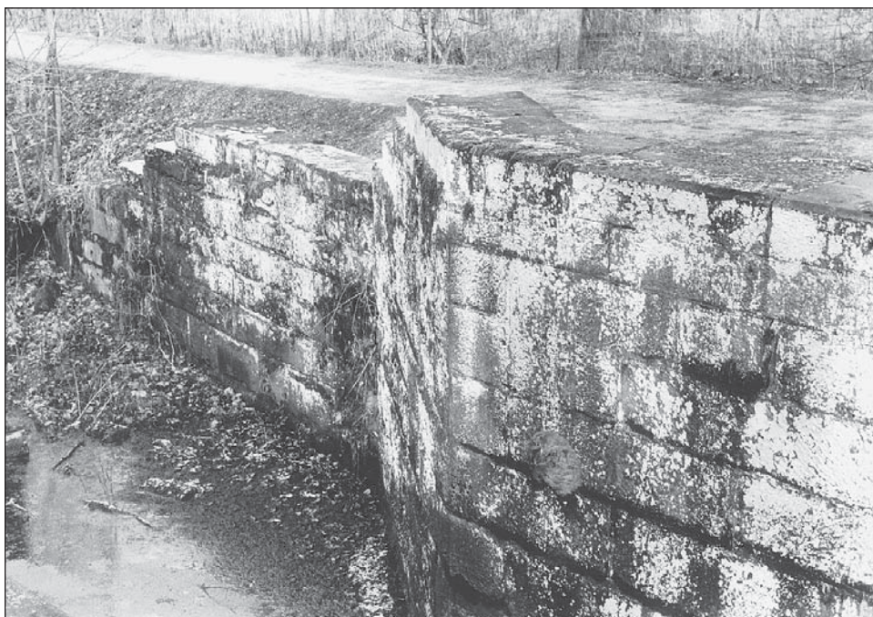
FIGURE 21. —Lower level end of Deep Lock, which is heavily encrusted by lichen and moss. Note towpath trail at top of photo. December 1997 photo.
