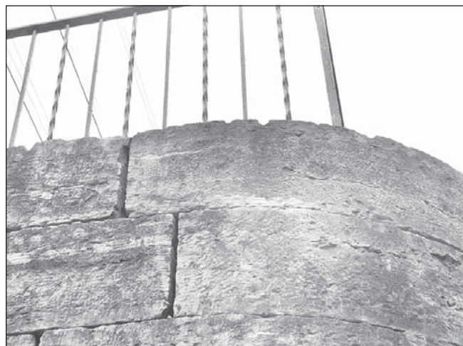
FIGURE 66.—West side of Lock 17, Carillon Historical Park, Dayton. Note grooves (in cross-sectional view here) made by ropes in top of coping of lock. Some horizontal bedding features of the limestone are preferentially weathered. August 1995 photo.
