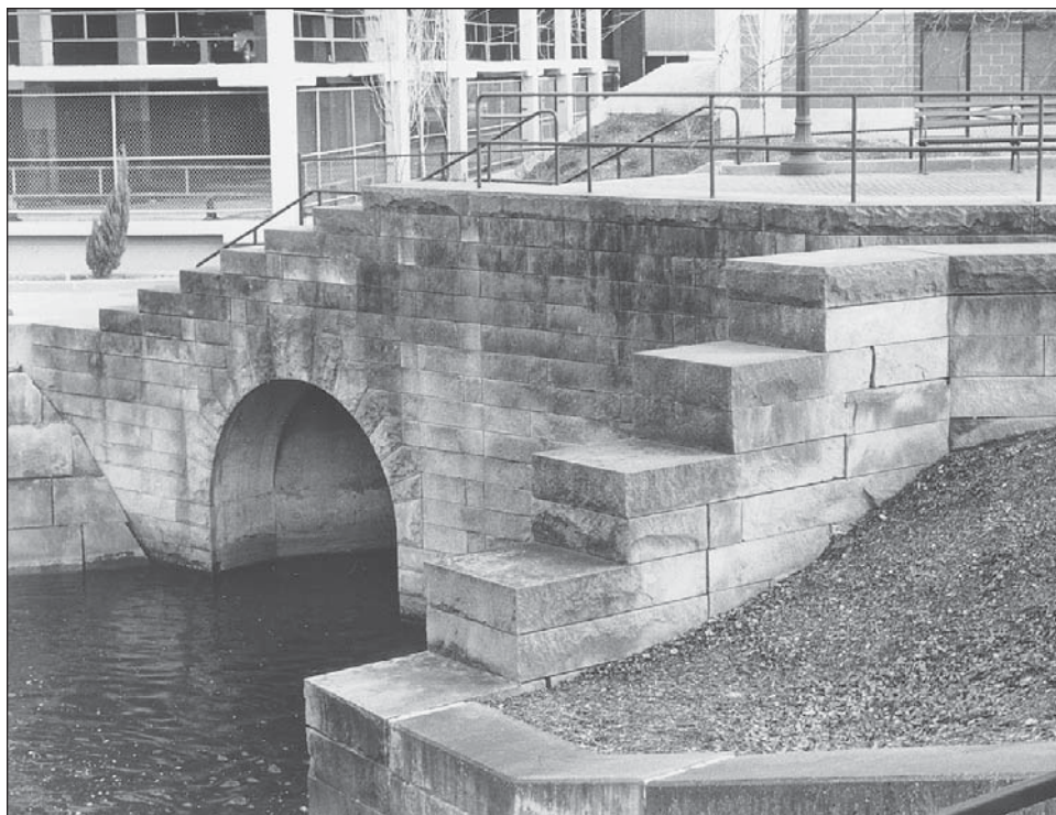
FIGURE 25.—Detail of Lock II Park. Stone used for reconstructed lock and as armoring for canal is Massillon sandstone. December 1997 photo.
