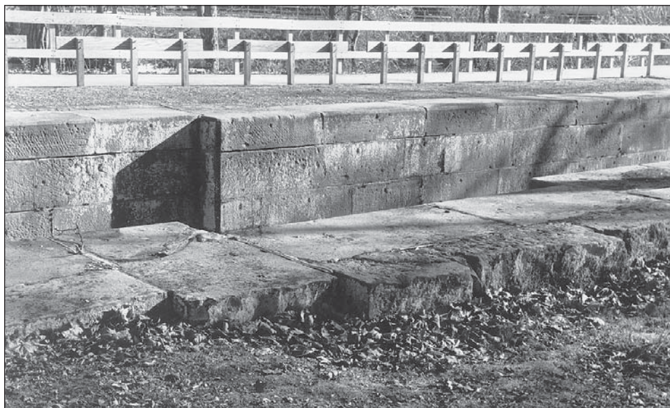
FIGURE 15.—Top portion of Lock 29. Note the angular quoins of the lock recess and the rough, unfinished outer edges of the stone across the center of the photo. November 1997 photo.
