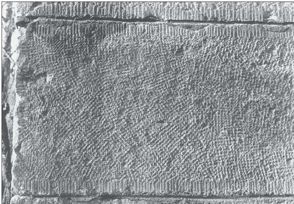
FIGURE 51.—Finely tooled stone block of Lock 4, Side Cut Metropark, Maumee. Note drafted margins and bush-hammered interior. December 1997 photo.
