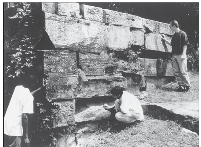
FIGURE 43.—Structure associated with Lock 44, Canal Park, Waverly. Several blocks have severely deteriorated. June 1995 photo.
