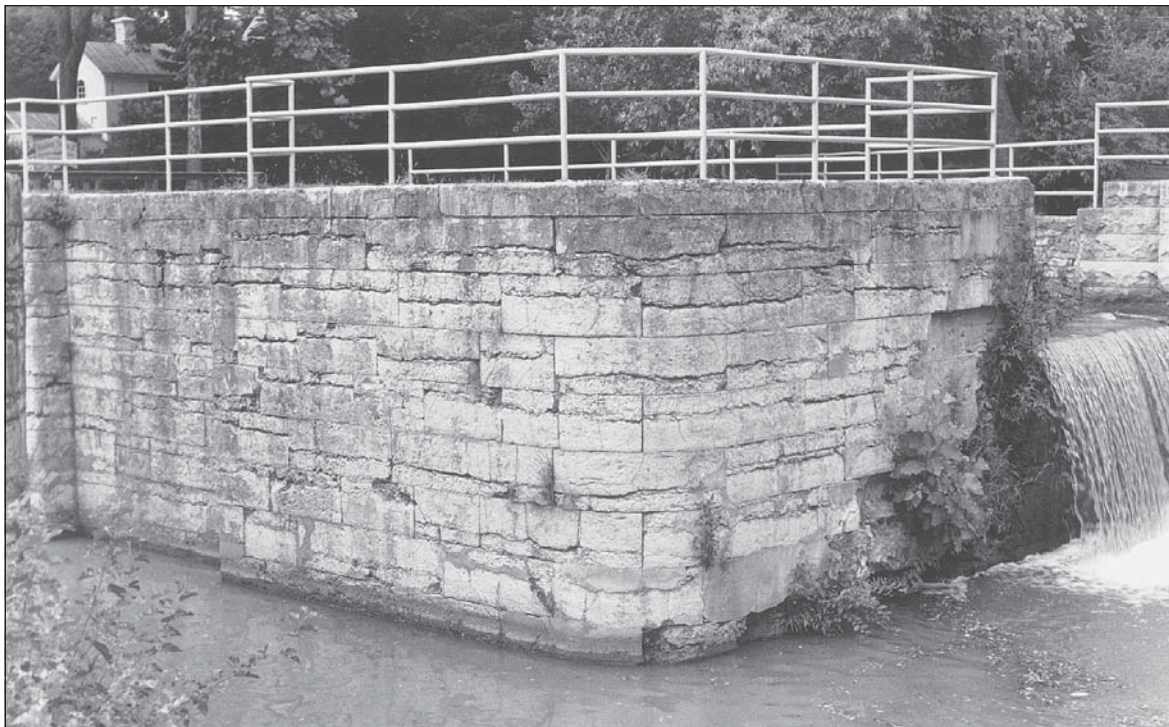
FIGURE 76.—Lock 25 and spillway of the Whitewater Canal, Metamora, Indiana. Many bedding planes of the stone blocks have weathered deeply. August 1995 photo.
