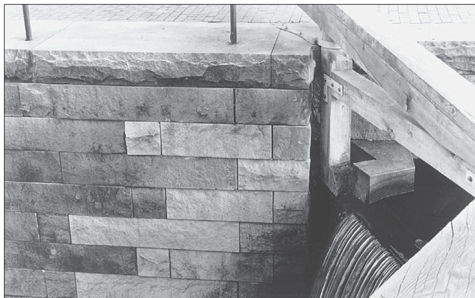
FIGURE 26.—Close-up view of stone used for reconstructed Lock II. Note that the finish of the stone does not attempt to replicate that of the original canal structures. It is split faced instead of bush hammered, as were most original canal stones. This difference in finish helps to identify the lock as a replica. December 1997 photo.
