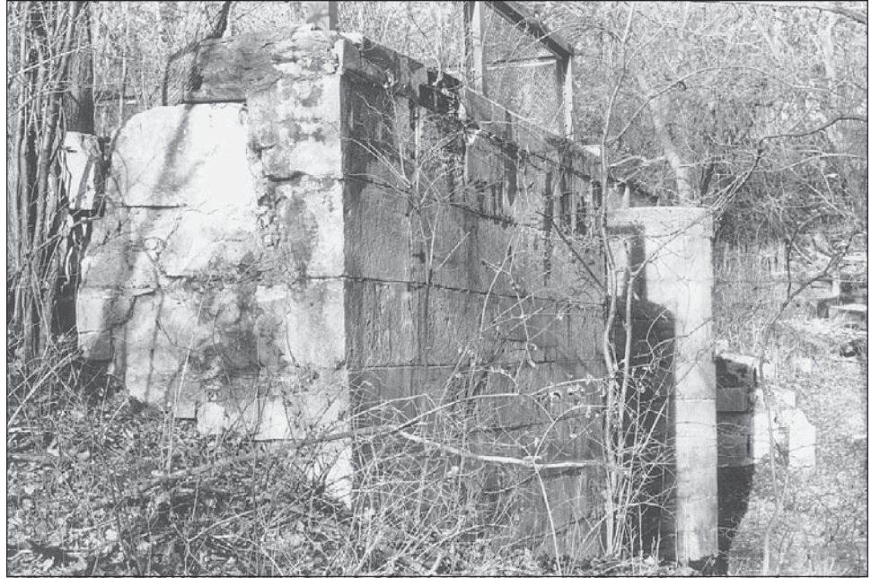
FIGURE 50.—Lock 4, Side Cut Metropark, Maumee. Unfinished stone to the left was not intended to be exposed. December 1997 photo.
