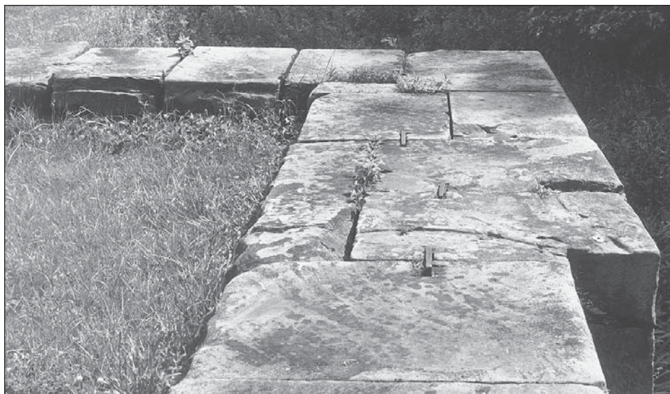
FIGURE 40.—Coping of Lock 26, off Canal Road just northeast of Lockbourne, showing typical squared-off ends of Ohio & Erie Canal locks. Note grooves for the goose necks (center right of photo) and three iron cramps used to tie blocks together. Cramps were used for various purposes along the canals, especially to strengthen coping near the heel posts. June 1997 photo.
