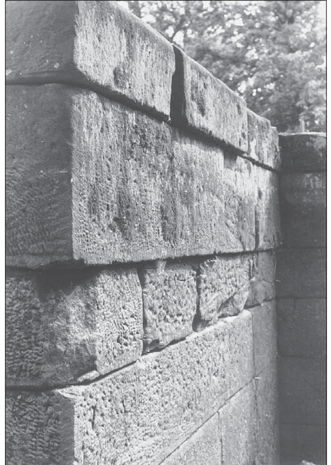
FIGURE 38.—Close-up view of the higher, east end of Lock 30, Lockbourne, showing state of stone blocks, weathered areas, drafted margins, etc. June 1997 photo.
