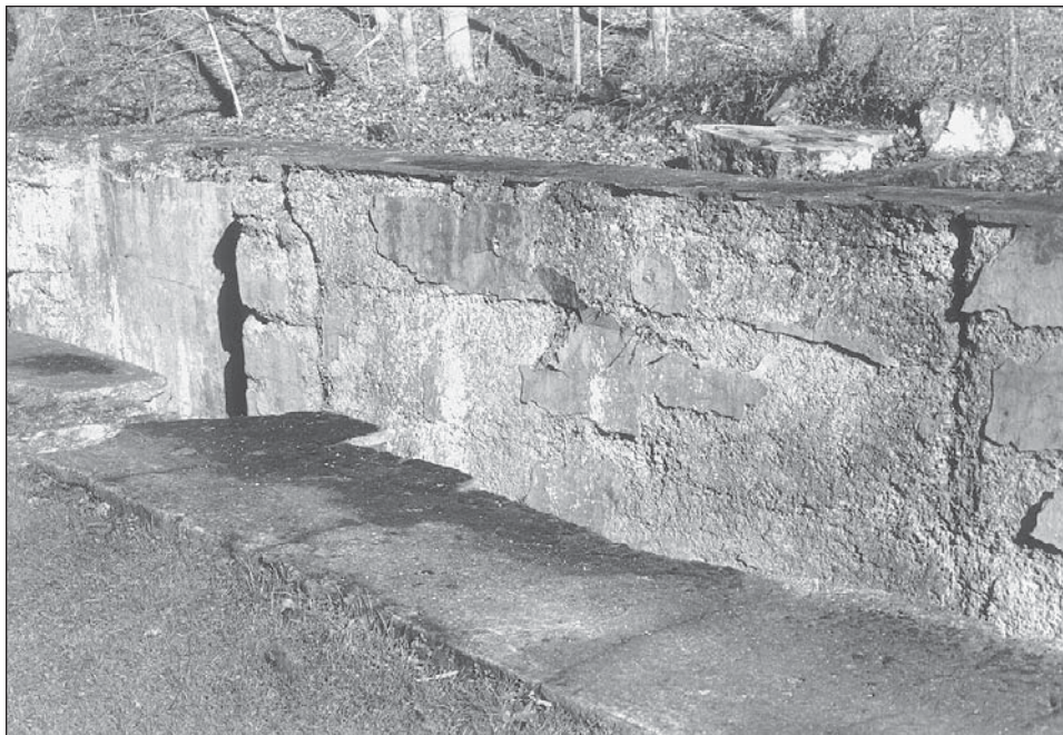
FIGURE 12.—Lock 30 of the Ohio & Erie Canal, Cuyahoga Valley National Recreation Area. This lock is composed mostly of concrete, which is exfoliating. Discarded stone from the original structure can be seen beyond the lock. November 1997 photo.
