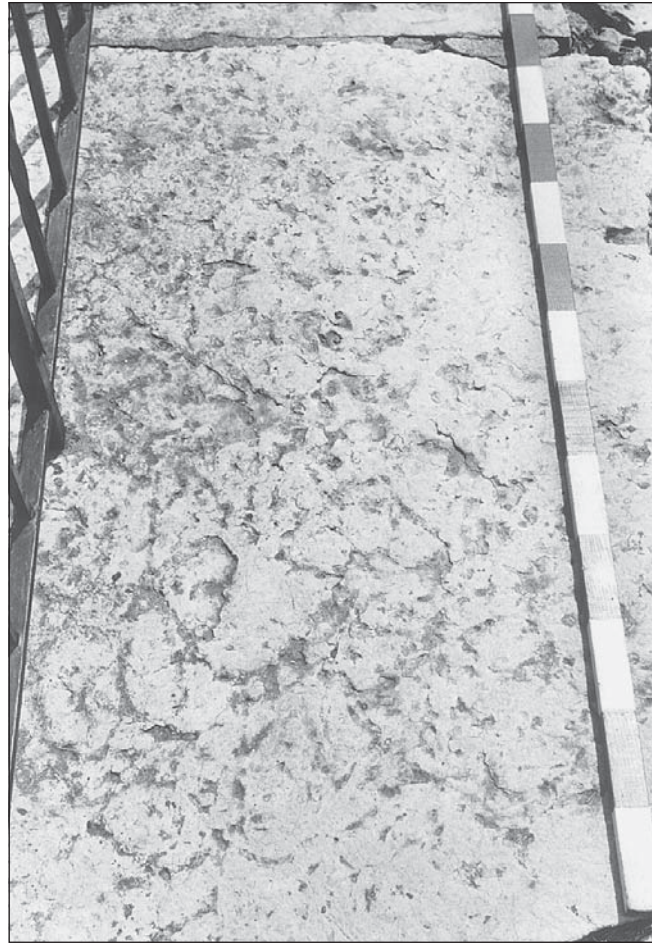
FIGURE 68.—Top of coping of Lock 17, Carillon Historical Park, Dayton, showing differential weathering of limestone. Pattern is probably due to trace-fossil content. Scale in decimeters. August 1995 photo.
