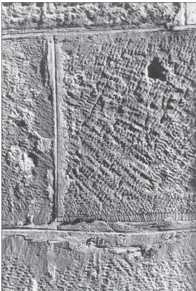
FIGURE 17.—Stone of Lock 29 showing roughly bush hammered interior, drafted margins, and cement mortar. November 1997 photo.
