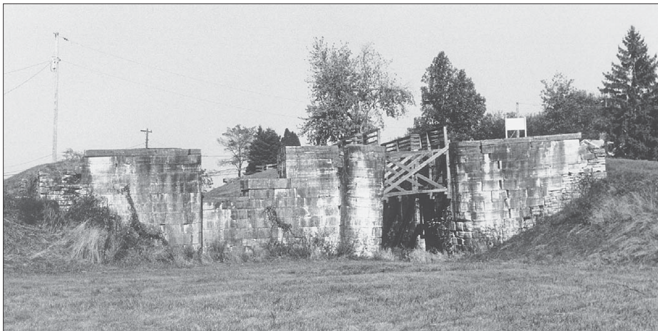
FIGURE 57.—Lower side of Lock 1, Big Lock, at Lockington. The tumble of the spillway is the two-level opening to the left; the lock chamber is to the right. October 1997 photo.
