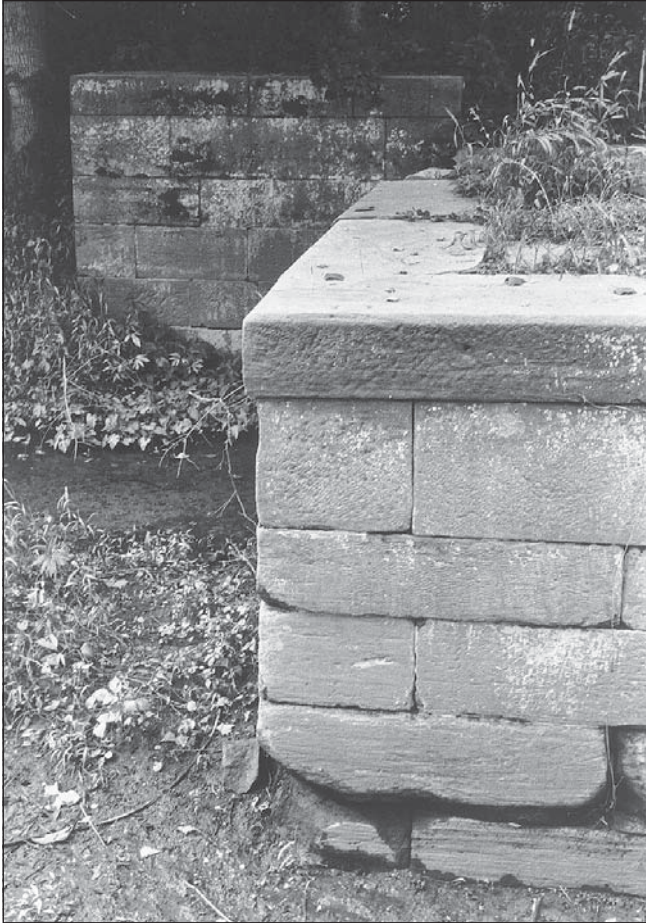
FIGURE 37.—Lock 30, Lockbourne, showing angular corners typical of Ohio & Erie Canal locks. Upper courses show original dressed faces. Lower courses have been weathered, exposing natural bedding of the stone. In the background is an unusual wall that extends from the spillway. June 1997 photo.
