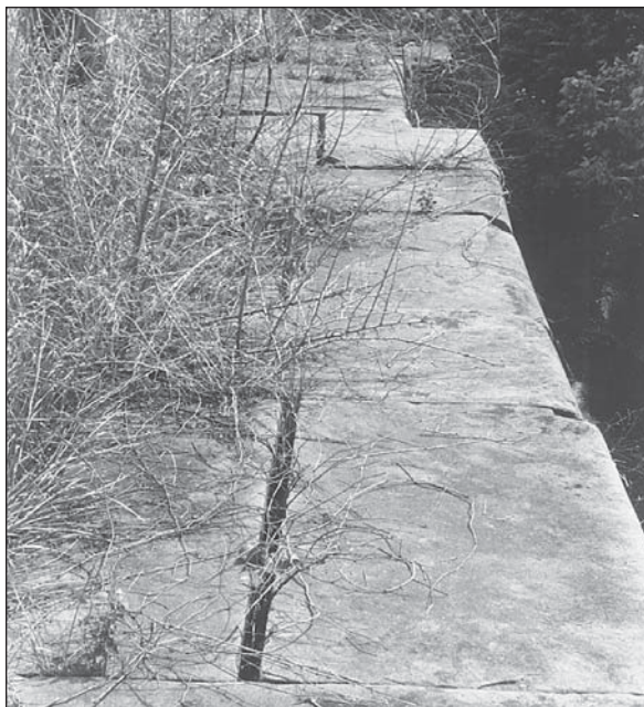
FIGURE 37.—Lock 30, Lockbourne, showing angular corners typical of Ohio & Erie Canal locks. Upper courses show original dressed faces. Lower courses have been weathered, exposing natural bedding of the stone. In the background is an unusual wall that extends from the spillway. June 1997 photo.
