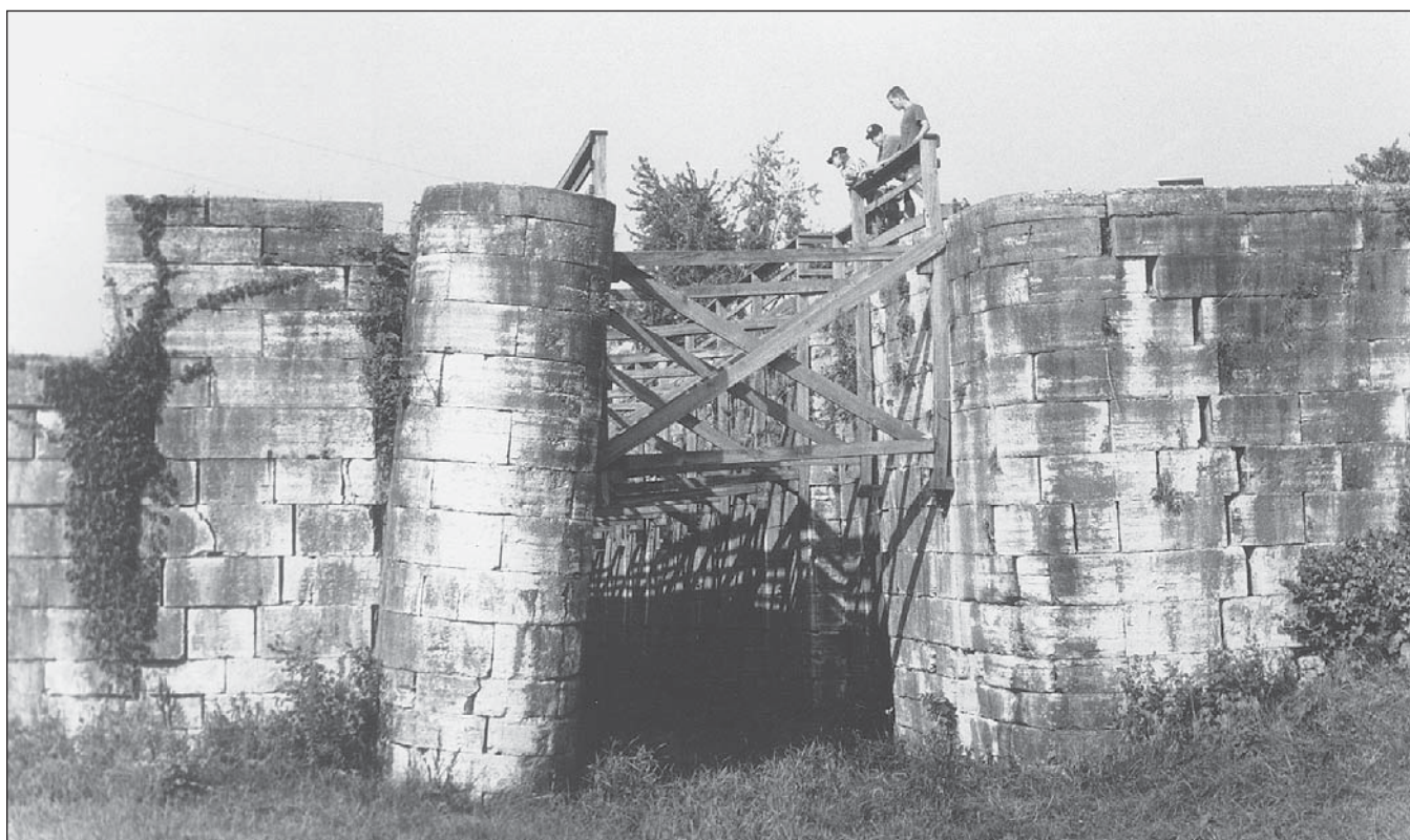
FIGURE 58.—Closer view of lower side of Lock 1, Big Lock, at Lockington. This lock is topographically high and is affected by a storm sewer just uphill. Note the inward tilt of the lock walls, the wooden structure holding the walls apart, and the separation of some of the blocks to the right. The edge of the spillway is to the left. August 1994 photograph.
