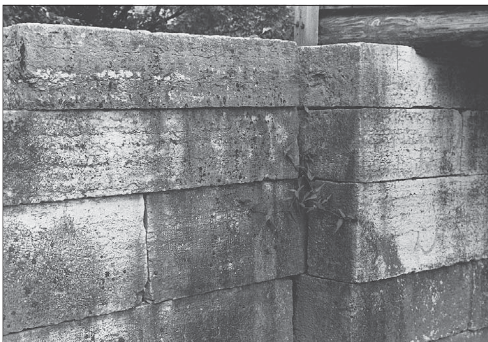
FIGURE 74.—Spillway at Lock 34, Excello, constructed of Dayton limestone . August 1998 photo.
