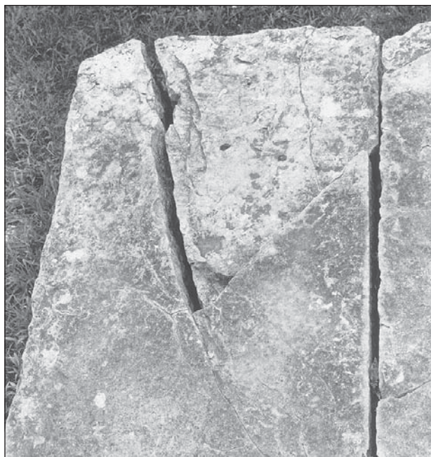
FIGURE 78.—Polygonal chunk of limestone breaking apart from coping of west end of Lock 25 at Metamora, Indiana. August 1995 photo.
